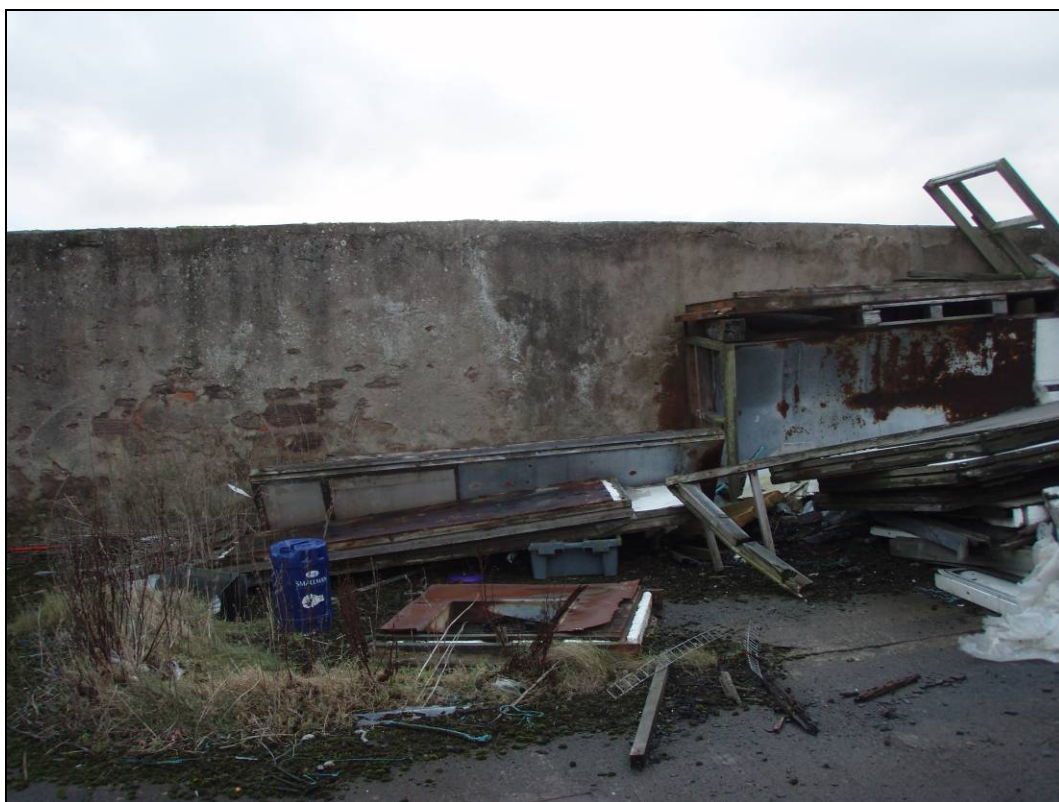
Figure 12. Wall 2 northeast facing elevation
