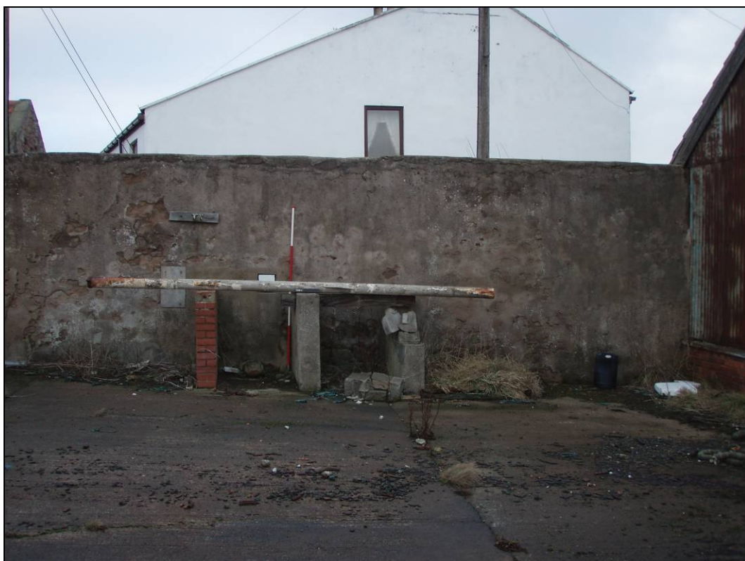
Figure 10 Wall 1 southeast facing elevation
