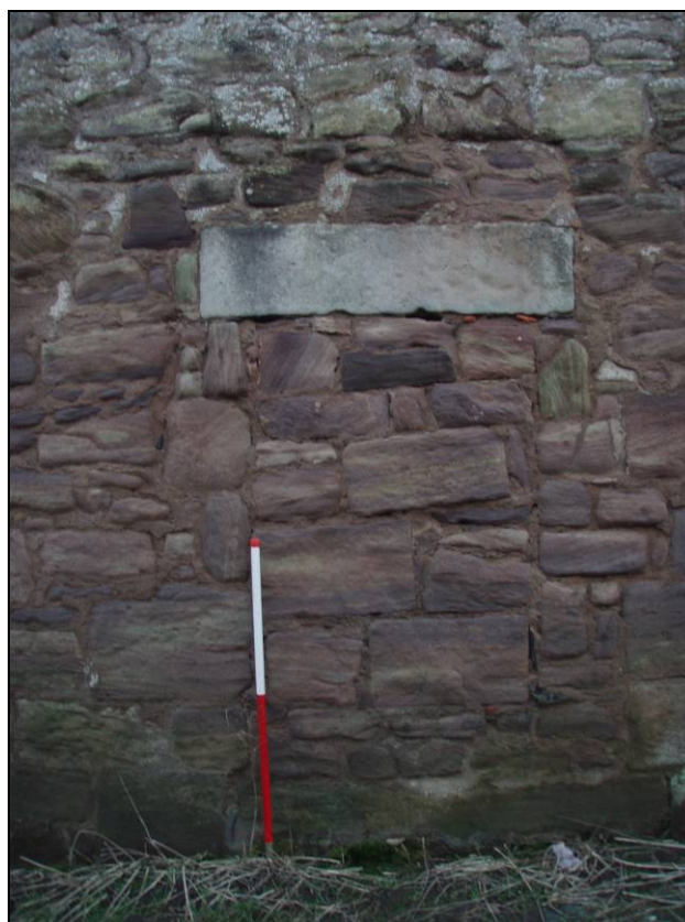
Figure 8. Wall 1 northwest facing elevation, blocked off opening.
