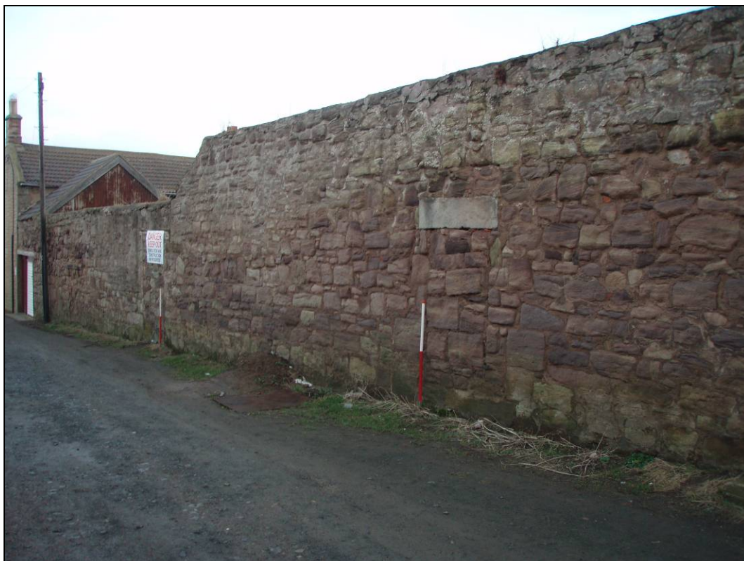
Figure 6. Wall 1 northwest facing elevation
