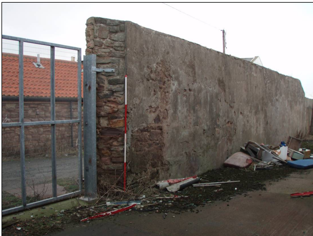
Figure 11. Wall 1 southeast facing elevation
