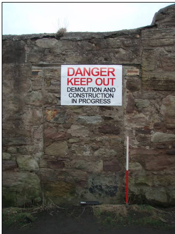
Figure 7. Wall 1 northwest facing elevation, more recent doorway
