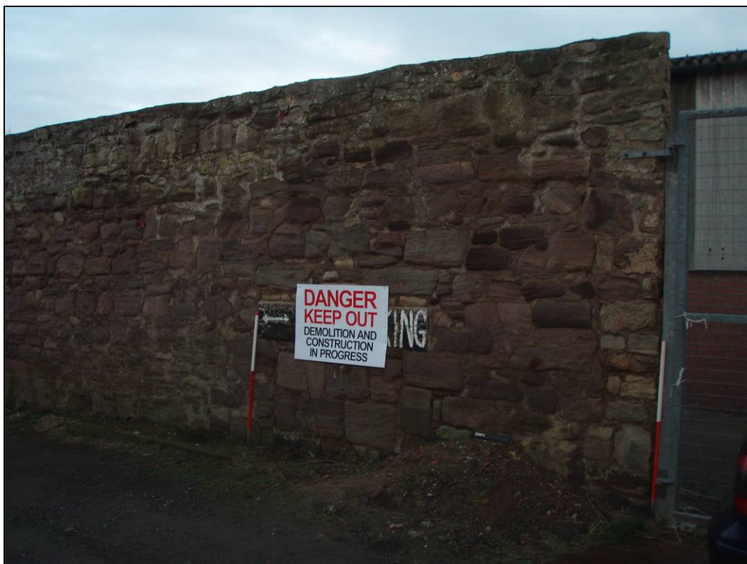
Figure 5. Wall 1 northwest facing elevation, blocked off opening
