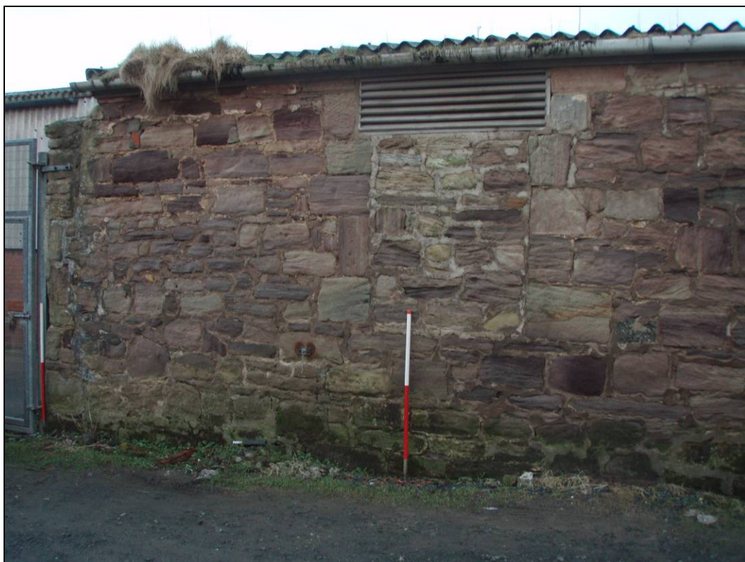
Figure 4. Wall 1 northwest facing elevation, blocked off door
