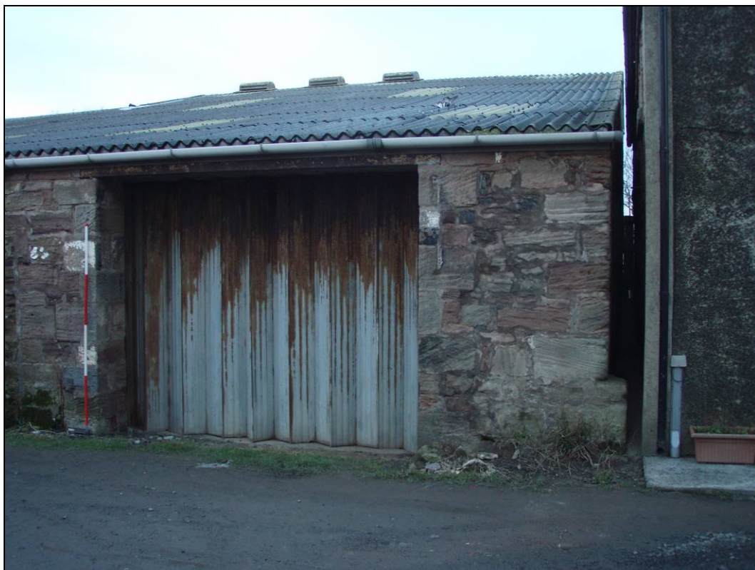
Figure 3. Wall 1 northwest facing elevation
