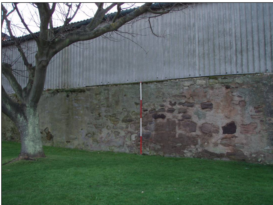
Figure 14. Wall 2 southeast facing elevation
