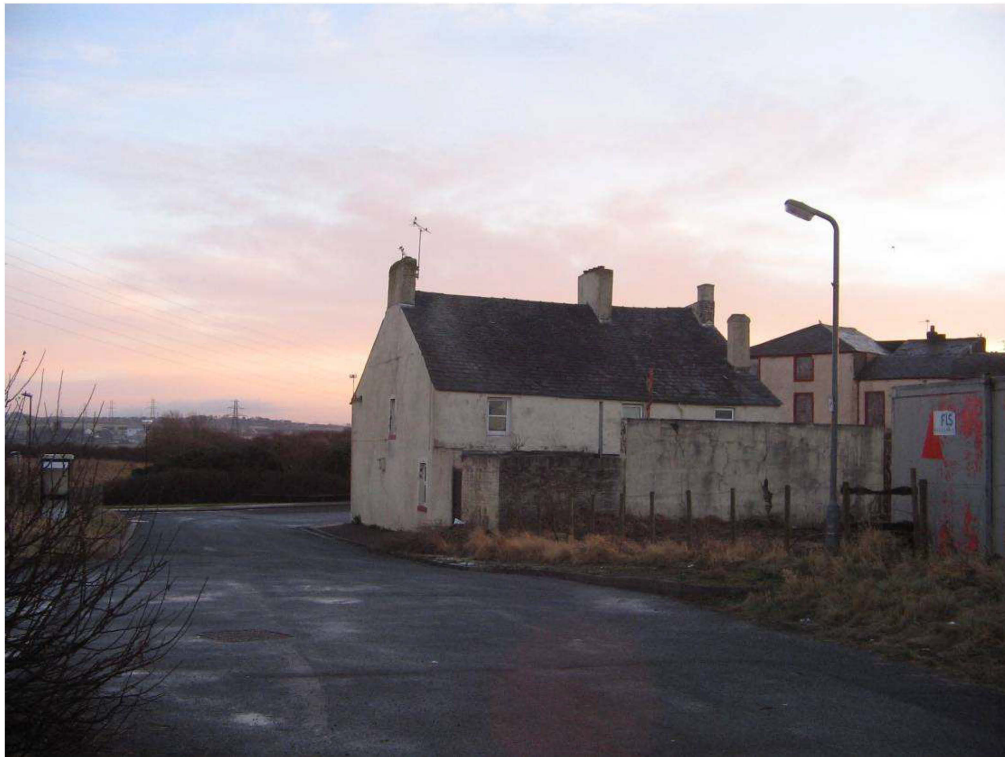
Figure 17: Looking E towards public house from w. extent of Solway Street.
