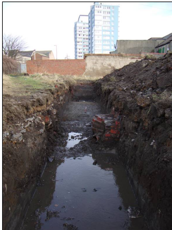
Figure 6 Trench looking west, from middle
