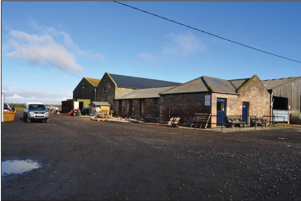
Figure 9. Southeast facing external elevation
