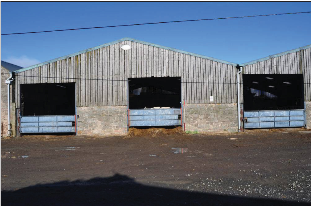
Figure 6. Southeast facing external elevation
