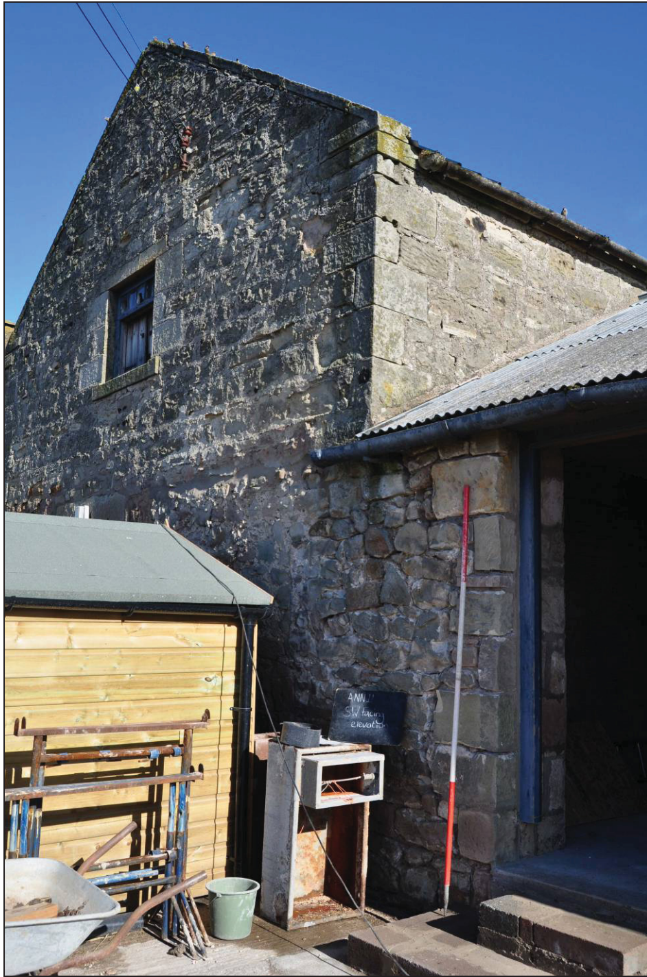
Figure 10. Southeast facing external elevation
