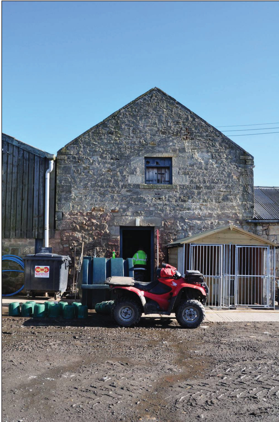
Figure 11. Southeast facing external elevation
