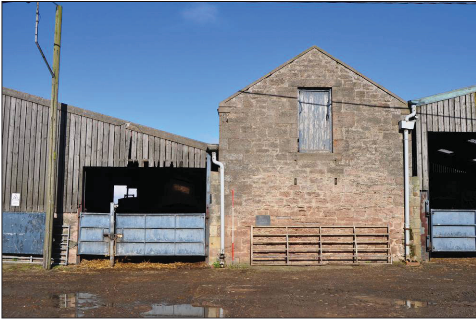
Figure 7. Southeast facing external elevation
