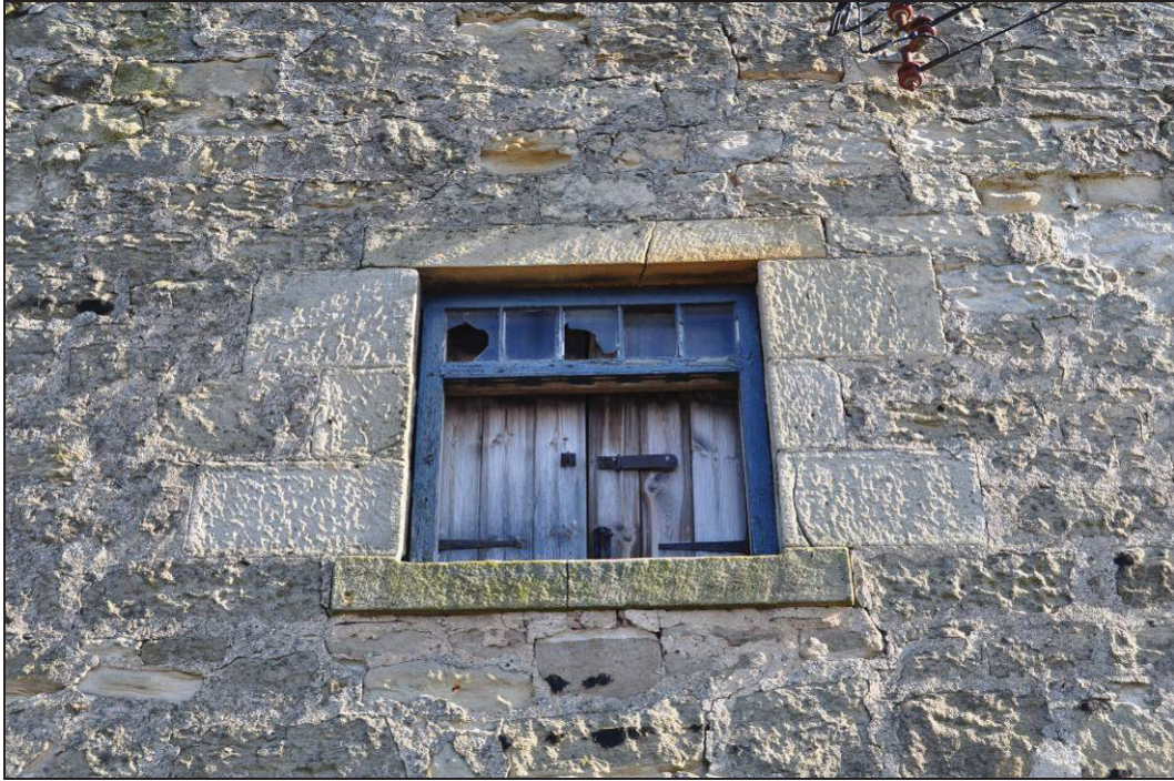
Figure 12. Southeast facing external elevation
