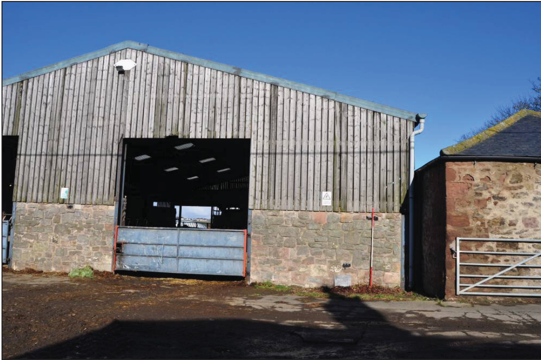
Figure 5. Southeast facing external elevation
