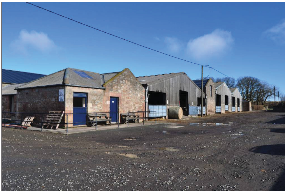
Figure 8. Southeast facing external elevation
