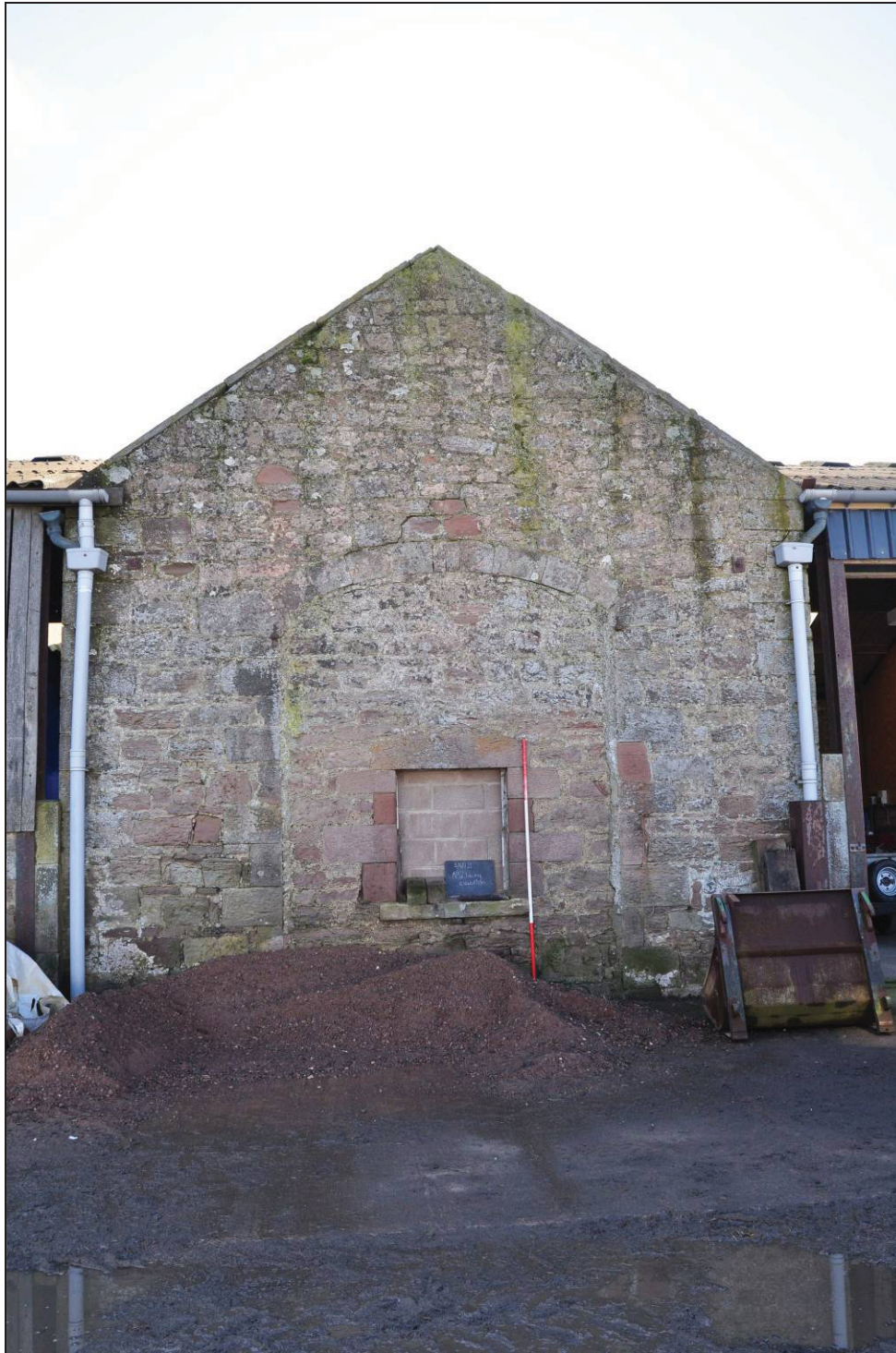
Figure 14. Southeast facing external elevation
