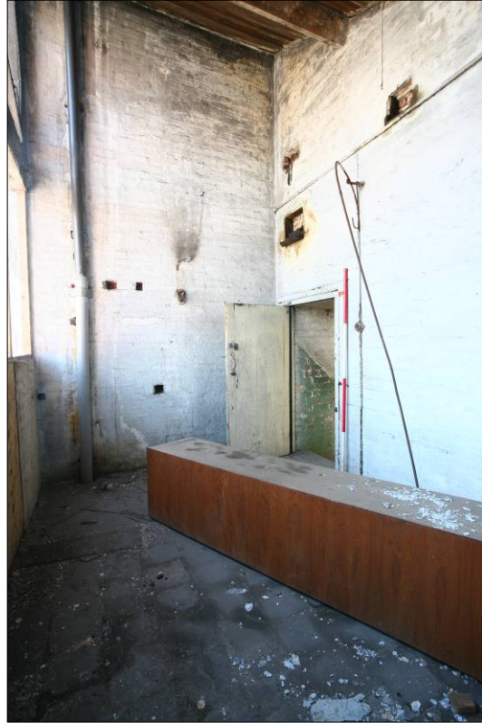
Figure 83. General view of Room F-4
