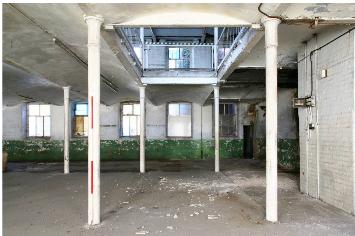
Figure 71. Inserted opening in the ceiling of Room F-1 leading.
