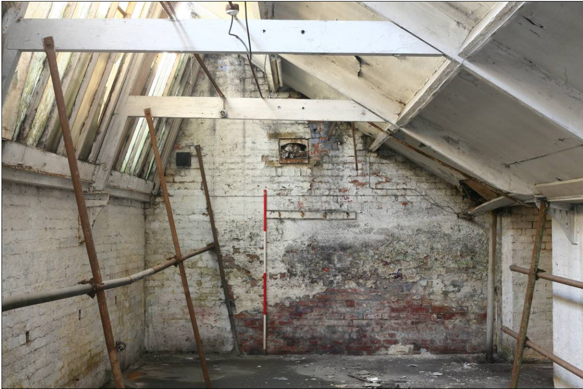
Figure 55. Bearing box in the west wall.
