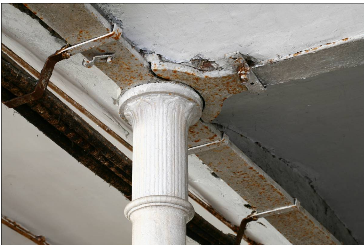
Figure 43. Detail of fluted foliage capitals supporting bowed beams.
