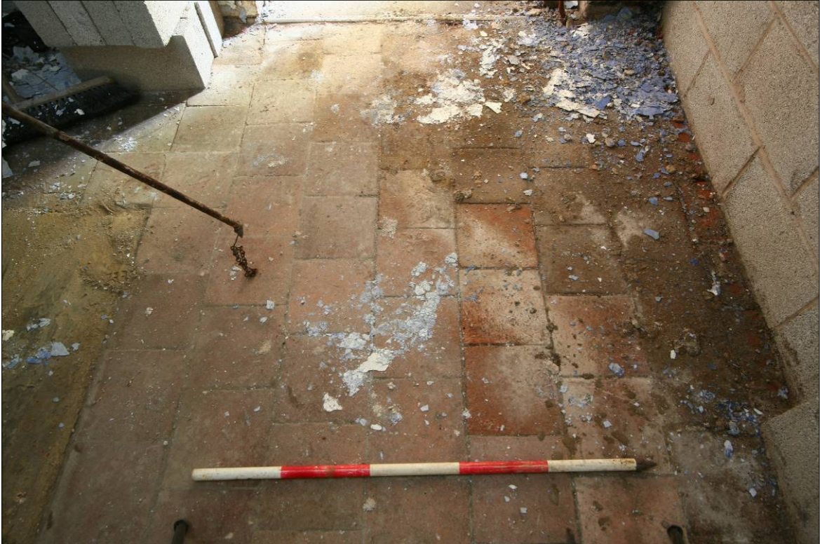
Figure 64. Detail of stone tiles, sandstone base and breeze block walling in room G-5.
