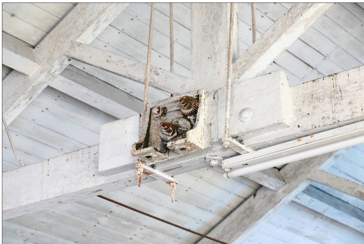
Figure 90. Detail of cast-iron bracket located on the roof truss.
