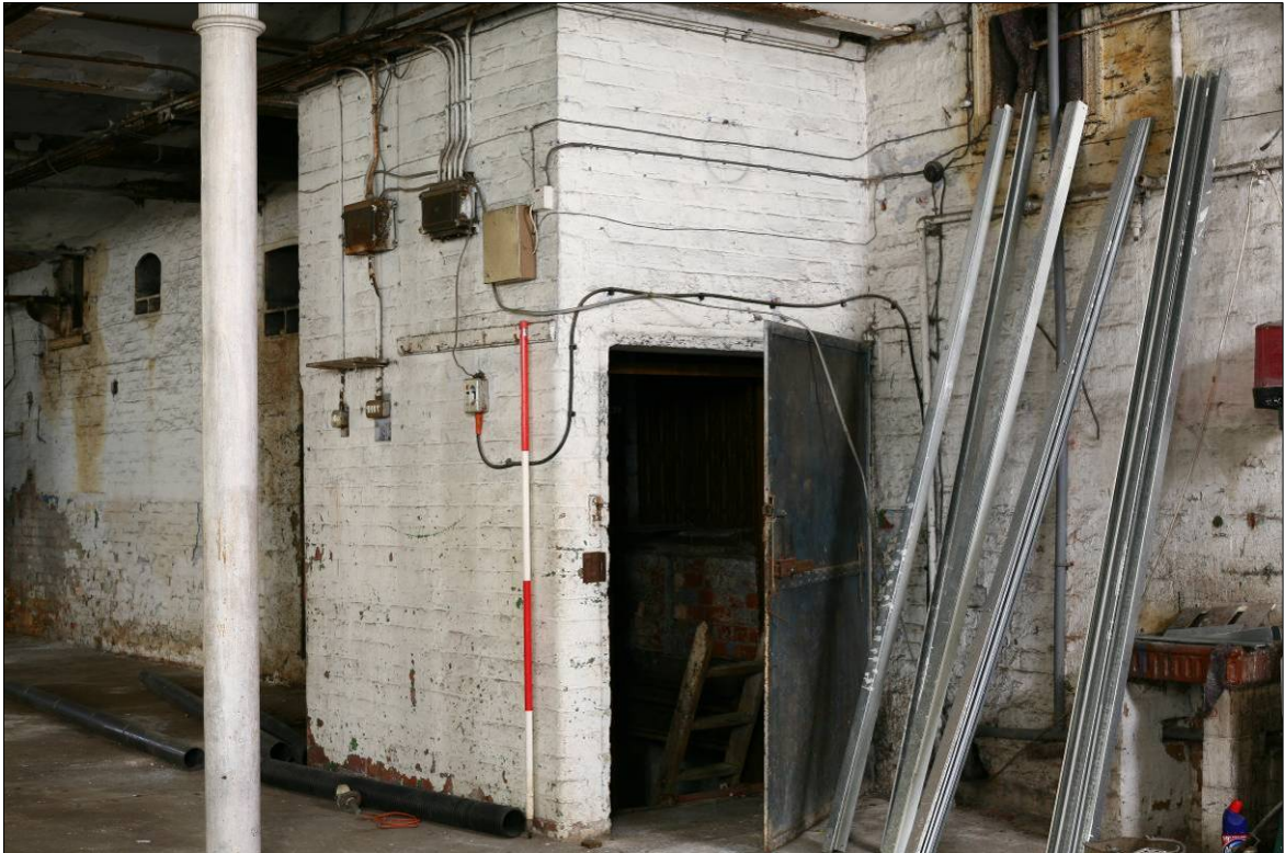
Figure 48. Inserted lift in the centre of the east wall.
