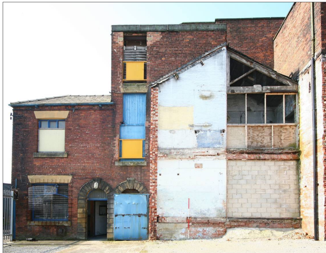
Figure 30. South portion of the East elevation.
