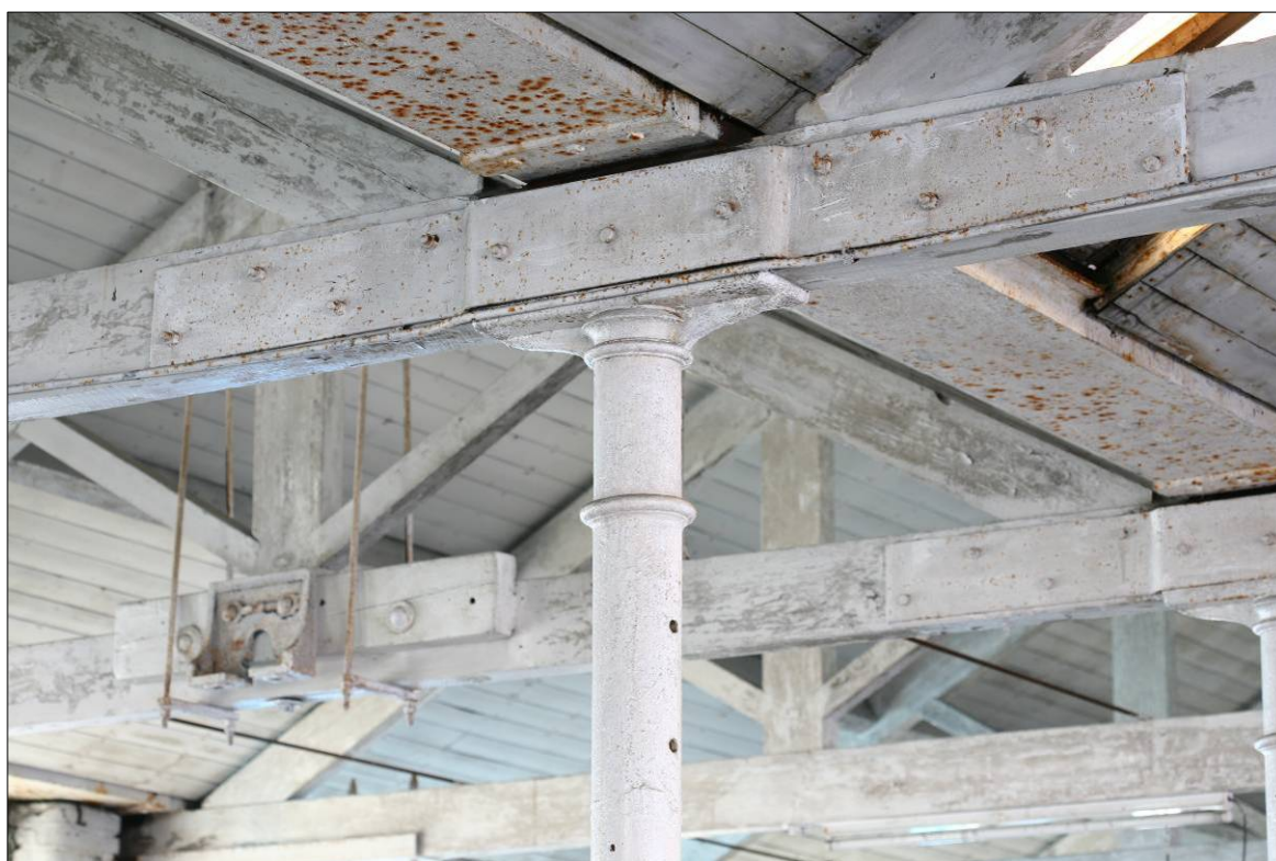
Figure 89. Detail of flanged column capitals.
