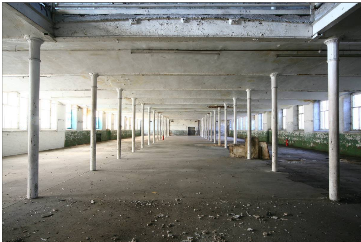
Figure 70. General view of Room F-1.
