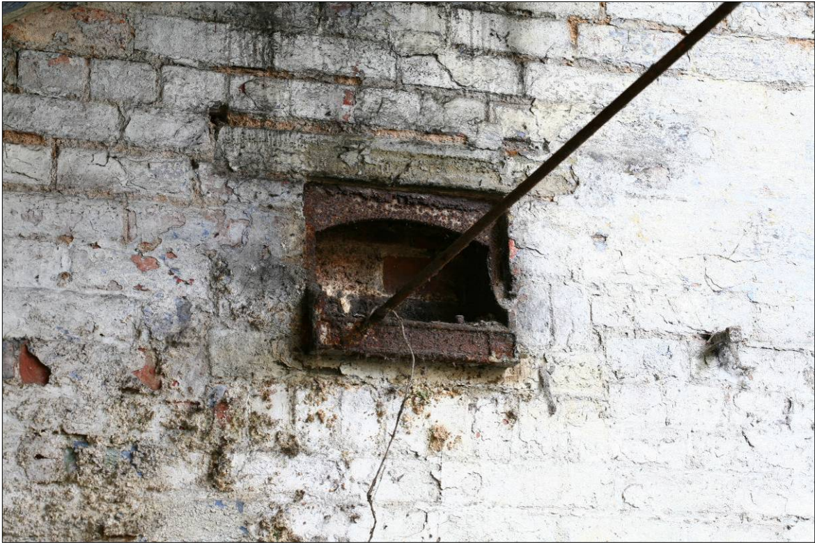
Figure 60. Bearing box in the west wall.
