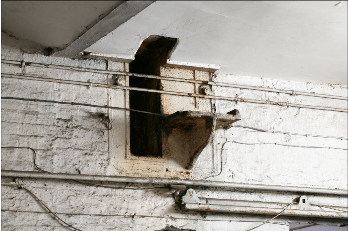
Figure 46. Detail of bearing box with bracket in the east wall.
