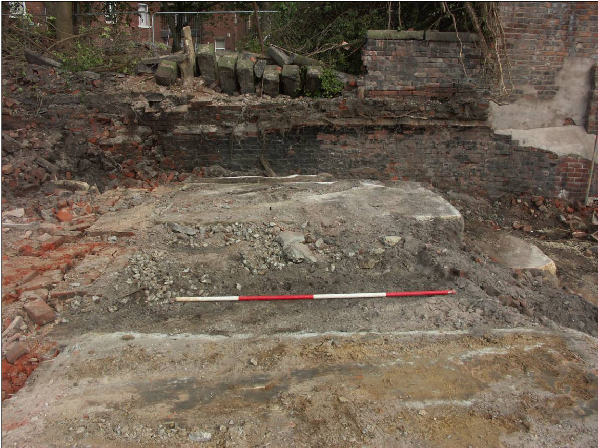
Figure 36. The engine-bed and piston-pit at the north end of the east wall.
