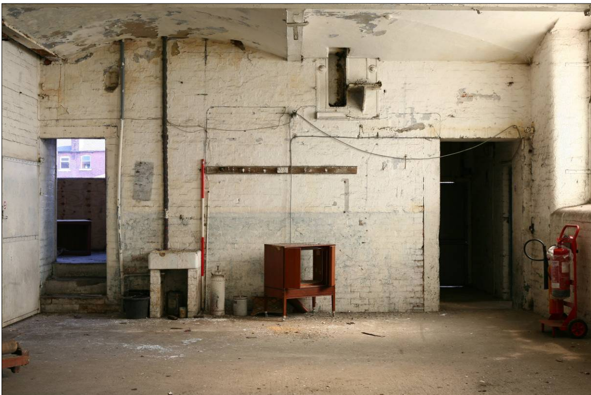
Figure 73. South end of the east wall showing the location of bearing boxes.
