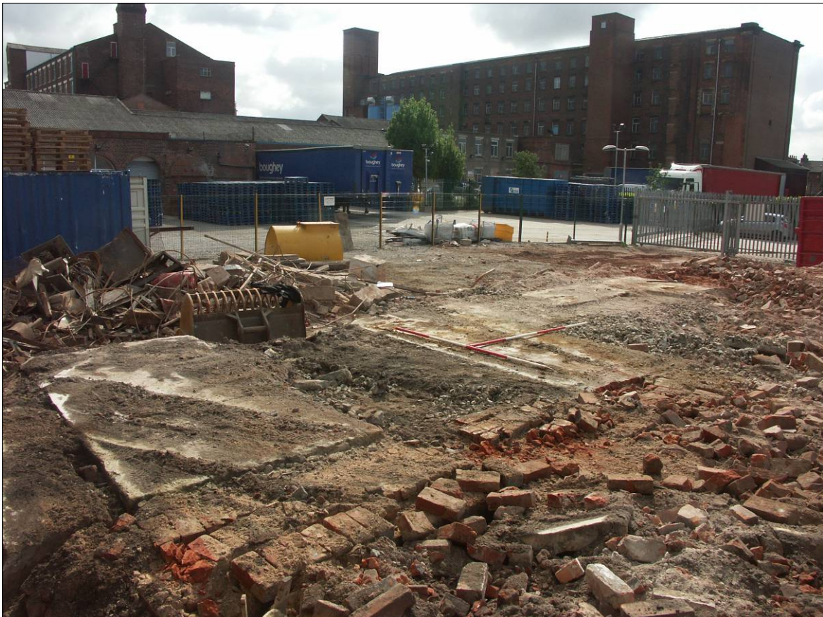
Figure 35. The extent of the engine bed facing southeast.
