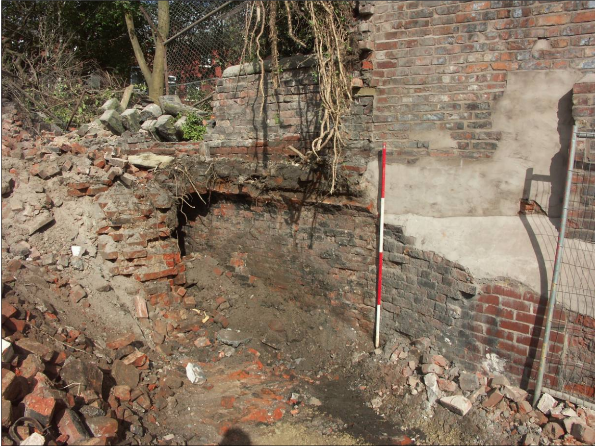
Figure 38. Brick-built flue from the southeast.
