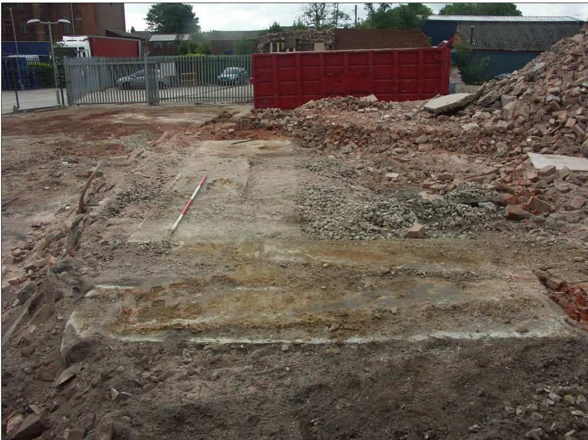
Figure 37. The engine bed facing south, with wheel-pit to the west.
