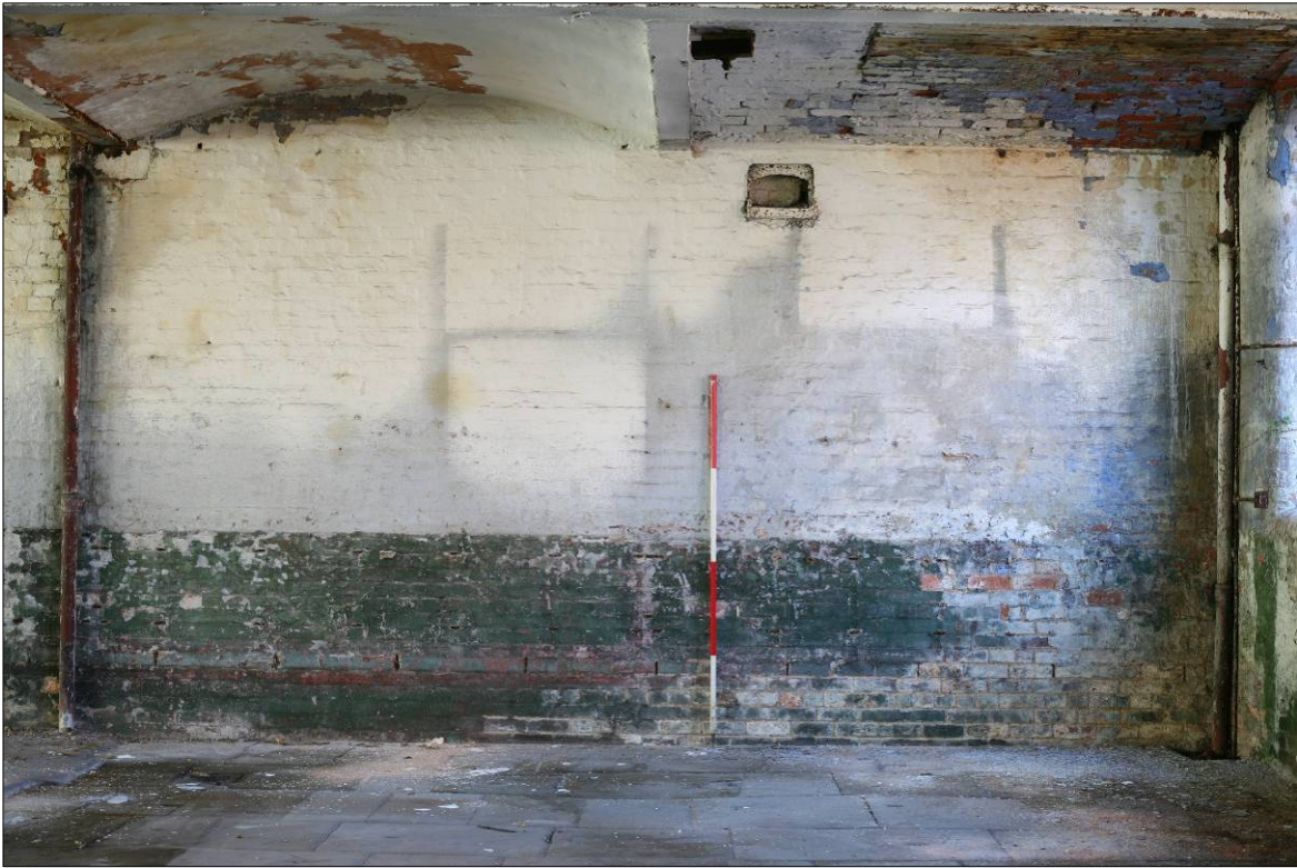
Figure 78. Bearing box in the west wall.
