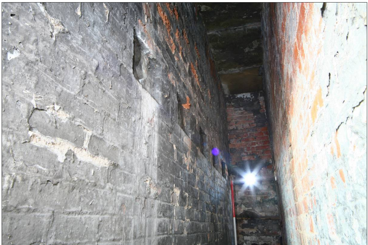
Figure 87. General view of Room F-6.
