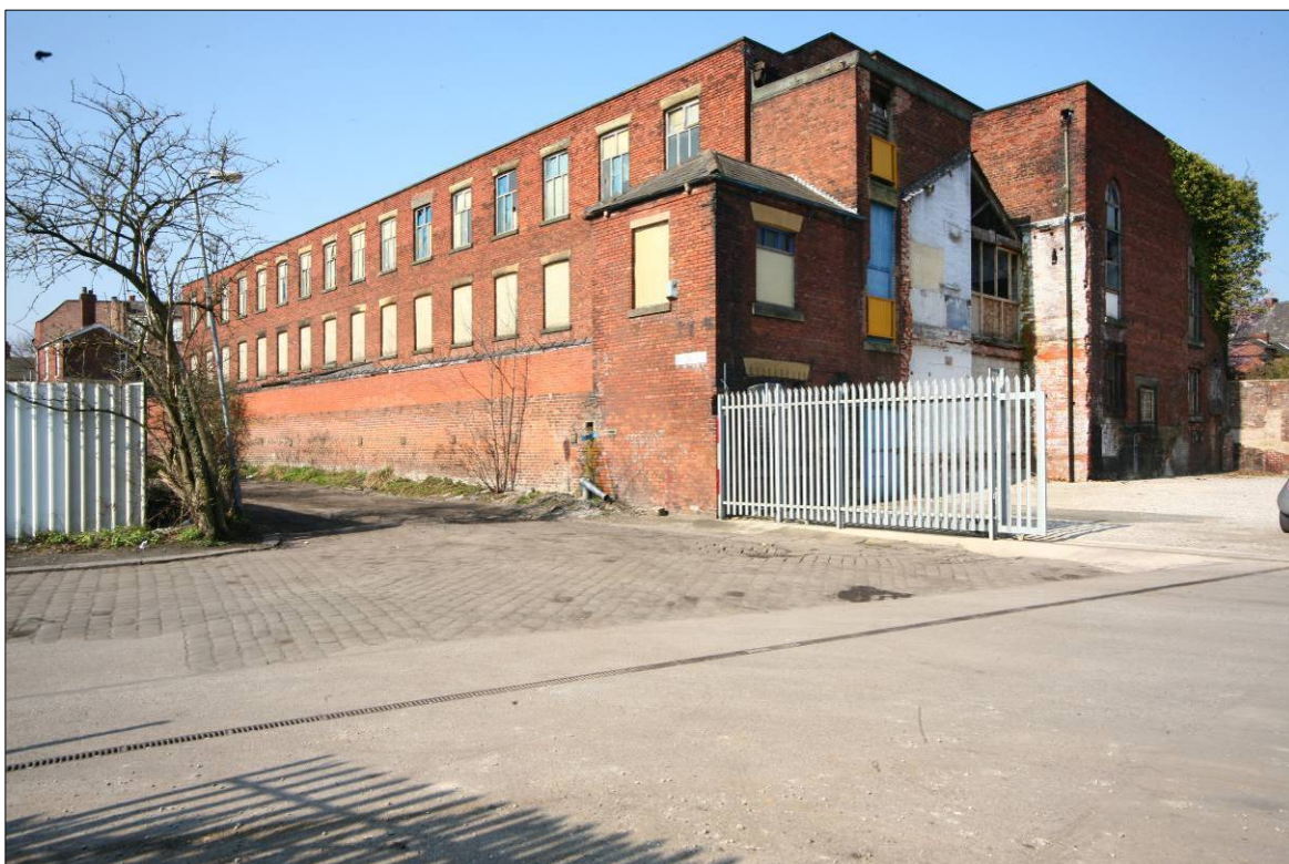
Figure 19. Site from the southeast.
