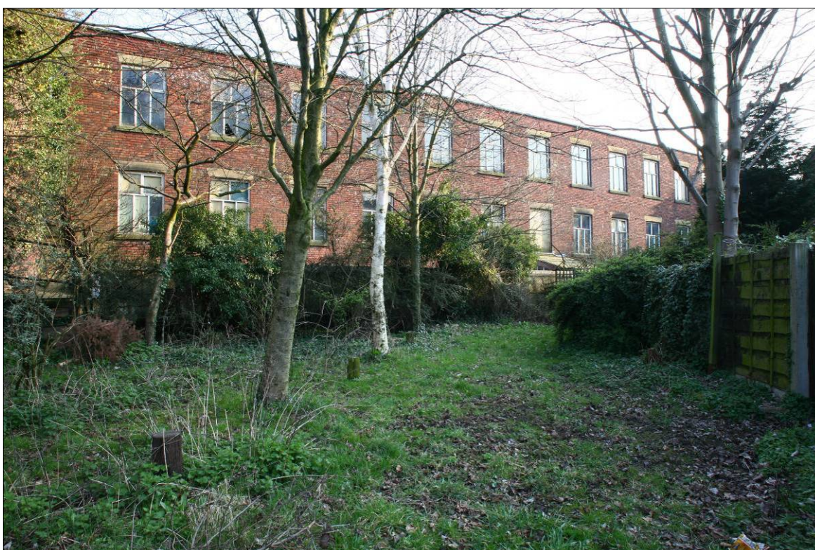
Figure 28. North elevation of the main mill.
