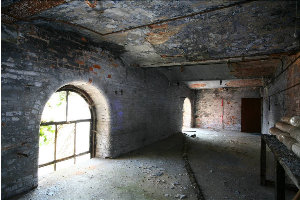
Figure 95. General view of Room S-3
