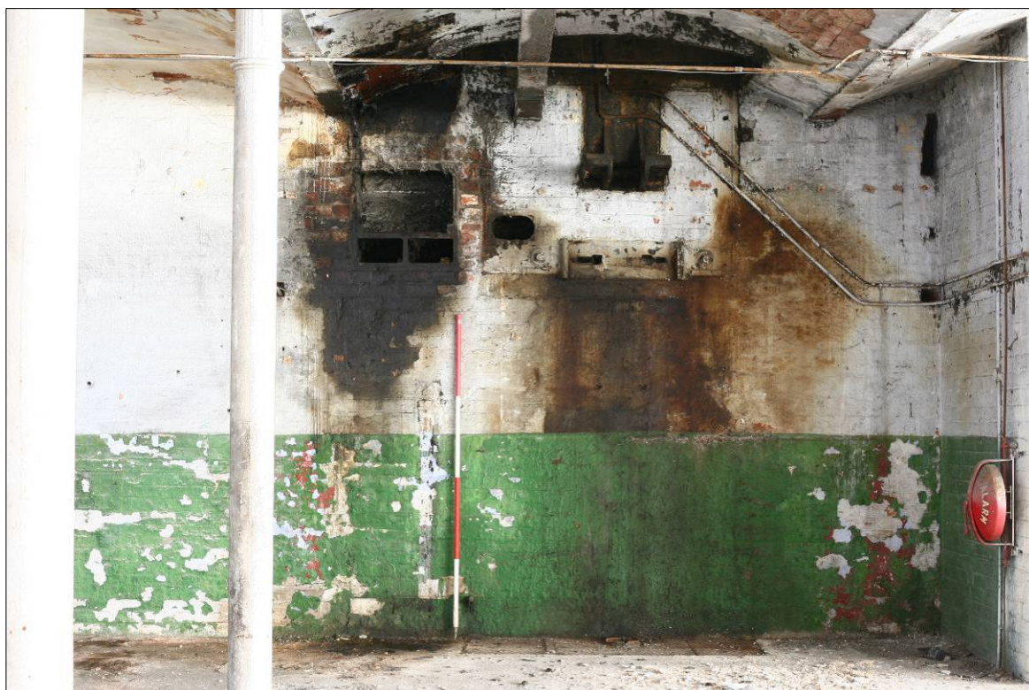
Figure 74. Centre of the east wall showing the location of bearing boxes.
