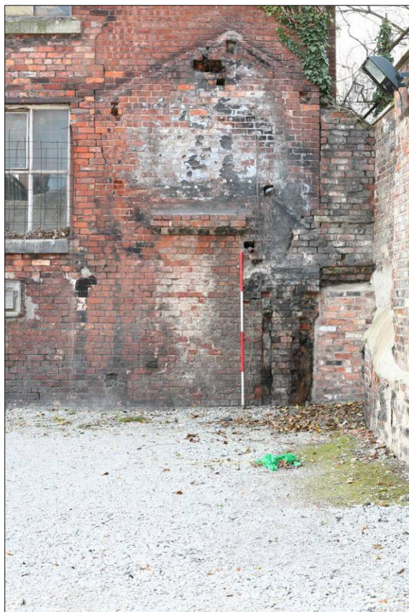
Figure 33. Detail of the demolished boiler house.
