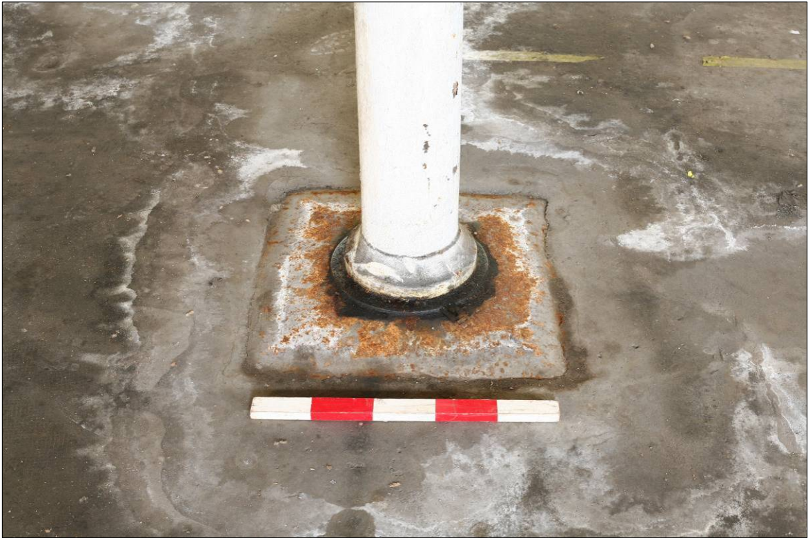
Figure 44. Concrete base of supporting cast iron columns.
