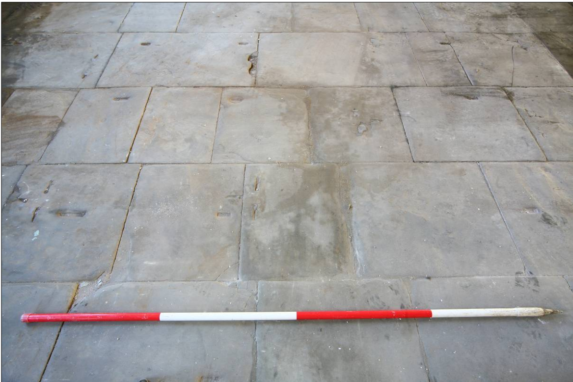
Figure 79. Detail of notches in the flagged stone floor marking the location of mill machinery
