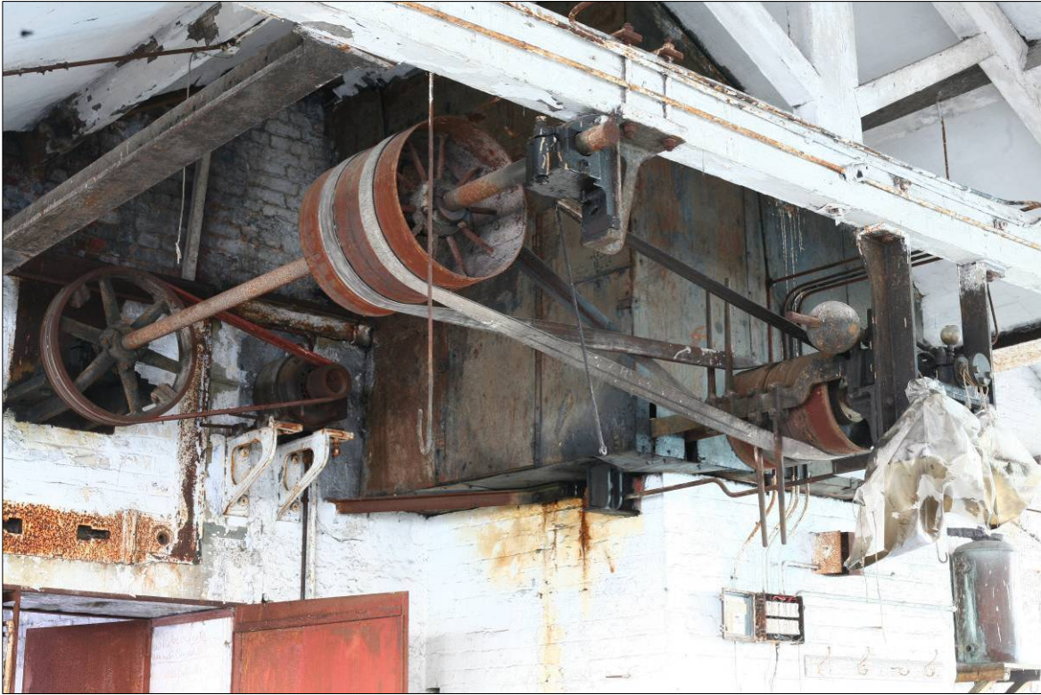
Figure 92. Detail of surviving gearing powering the inserted lift in the centre of the east wall.
