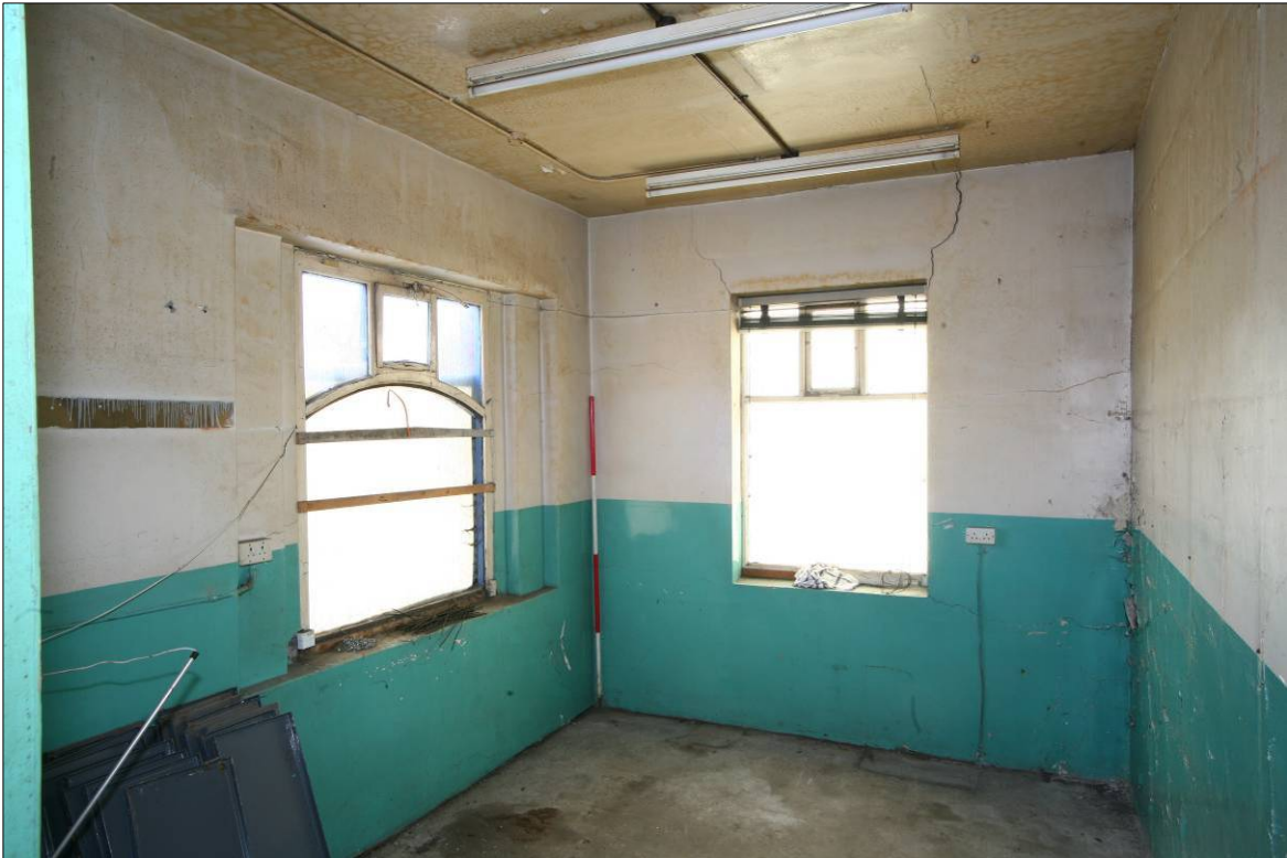
Figure 81. General view of Room F-2.
