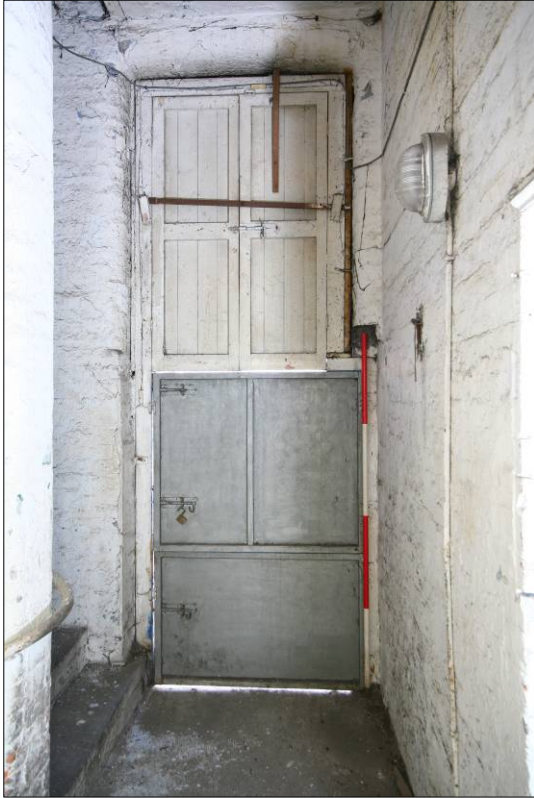
Figure 82. General view of Room F-3.
