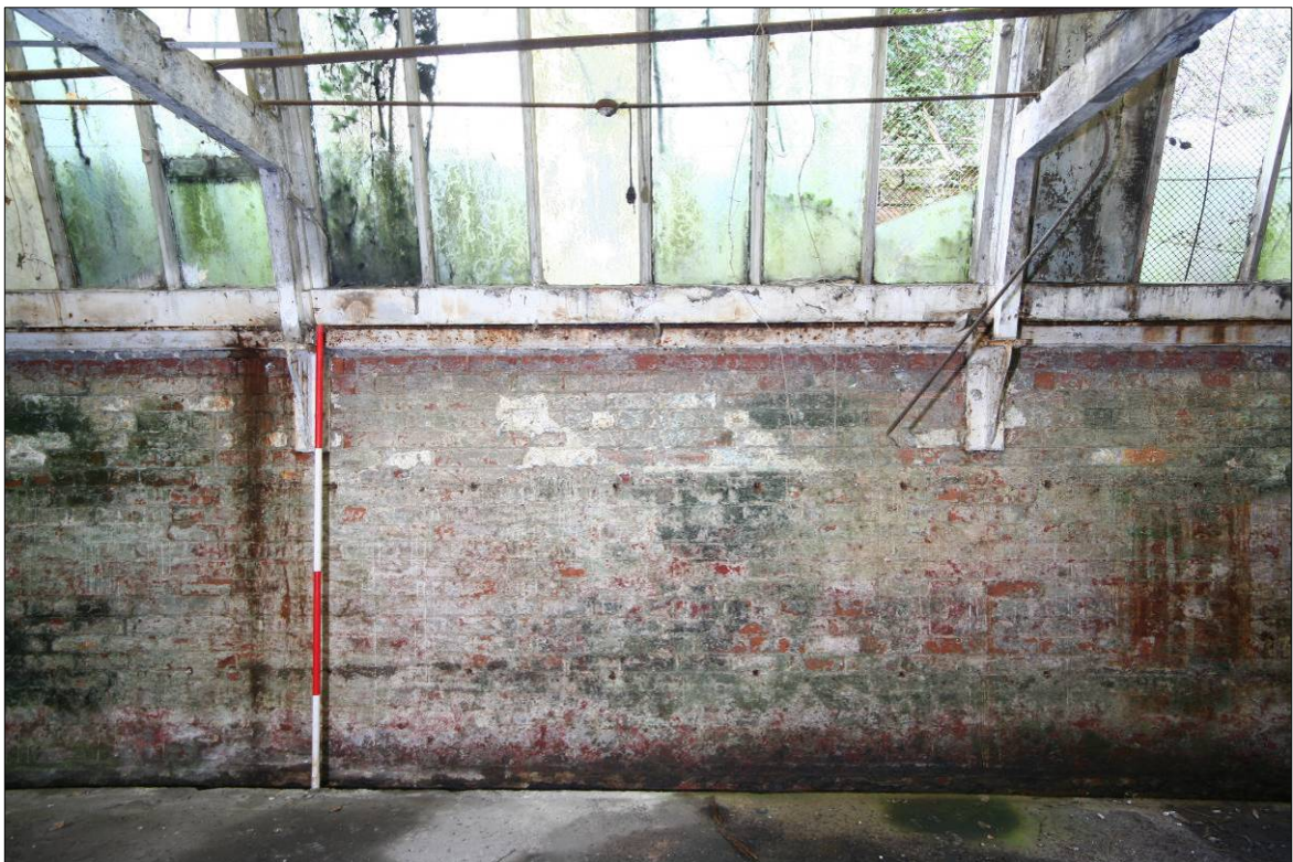
Figure 57. Evidence for a frame attached to the north wall.
