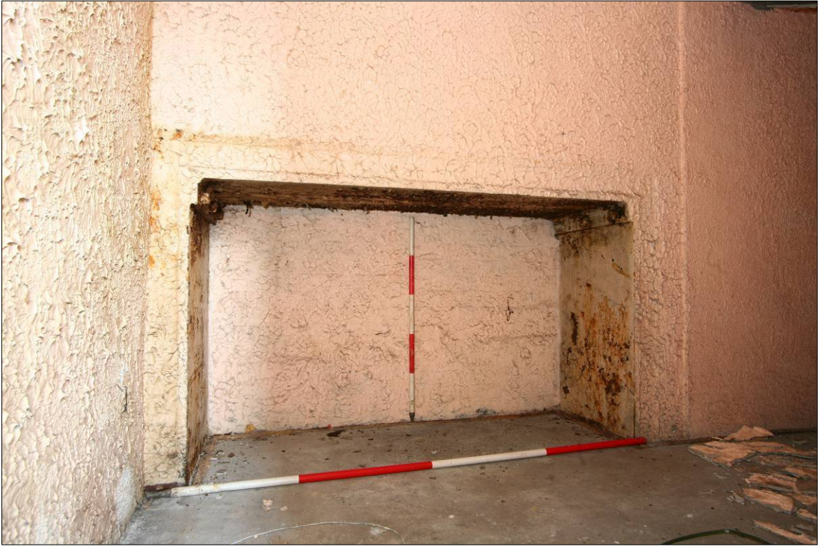
Figure 65. Blocked opening through to Room G-1 in the west wall.
