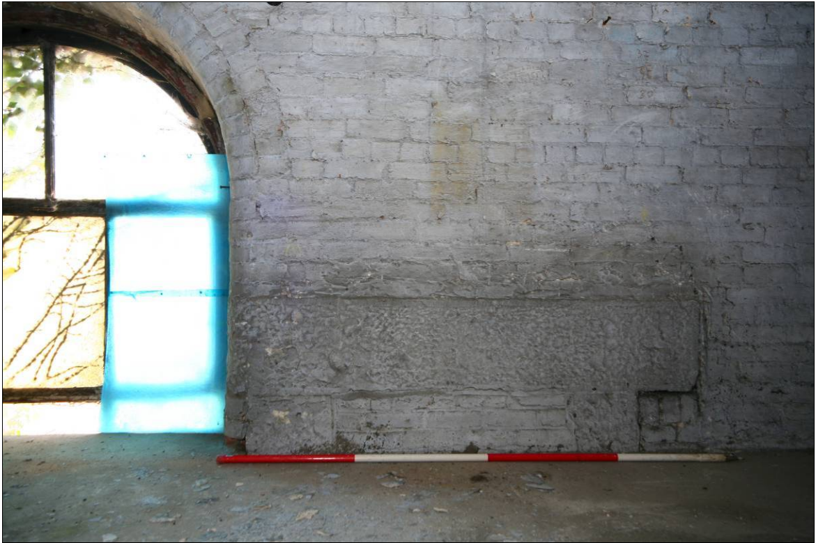
Figure 96. Detail of sandstone inclusion in the east wall.
