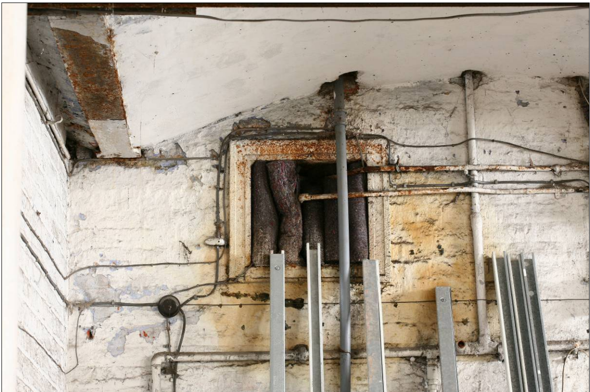
Figure 46. Detail of bearing box with bracket in the east wall.
