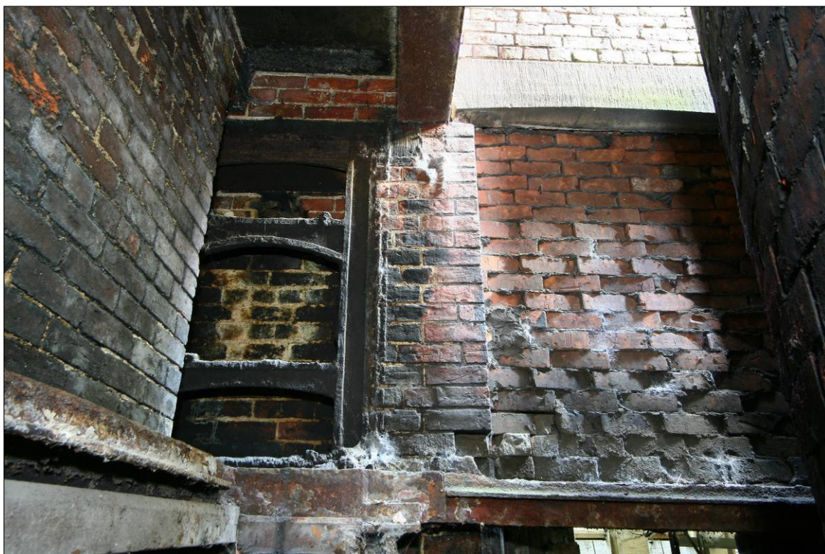
Figure 69. Detail of bearing box and blocked window in the south wall.
