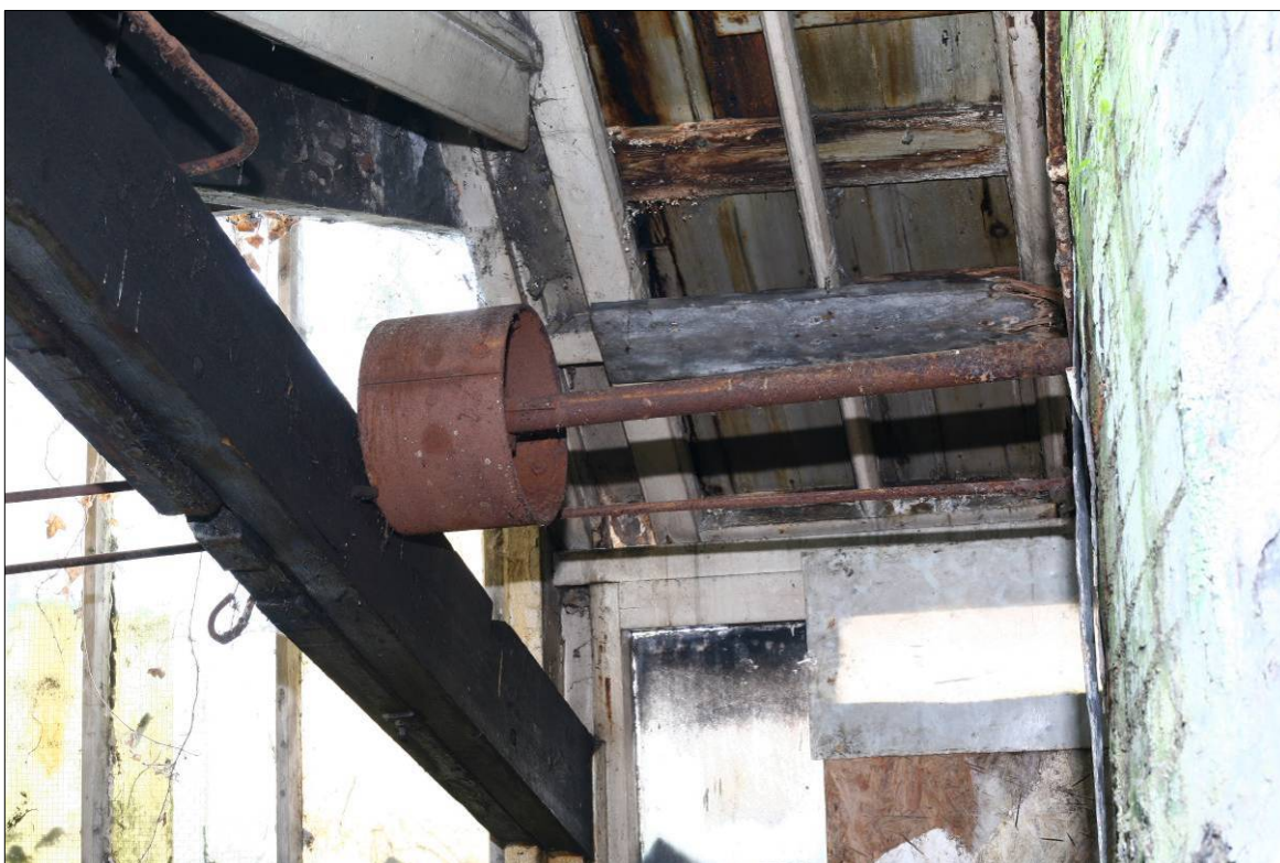
Figure 58. Detail of a surviving pulley on the east wall.
