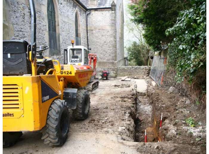
View of excavated trench
