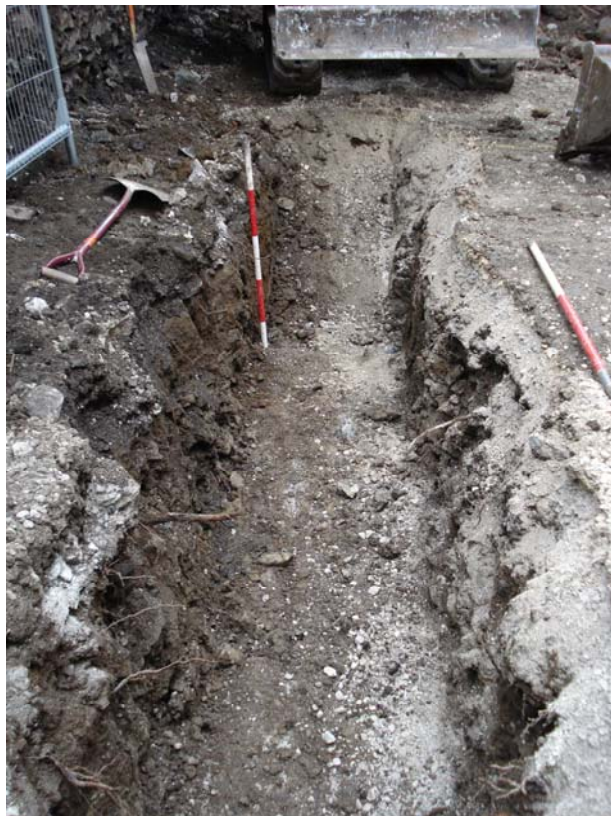
Figure 3: View of excavated trench
