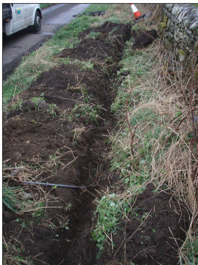
Figure 4. Trench with armoured copper cable installed.
