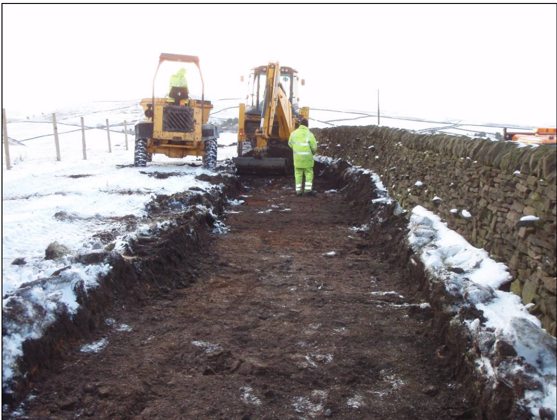
Figure 6: Excavation of the northern section of the bridleway, looking south
