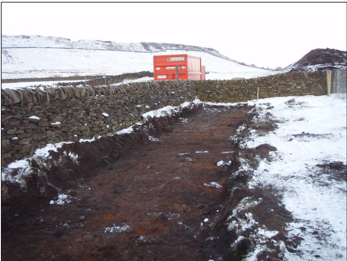
Figure 8: Northernmost end of the new bridleway section, looking north
