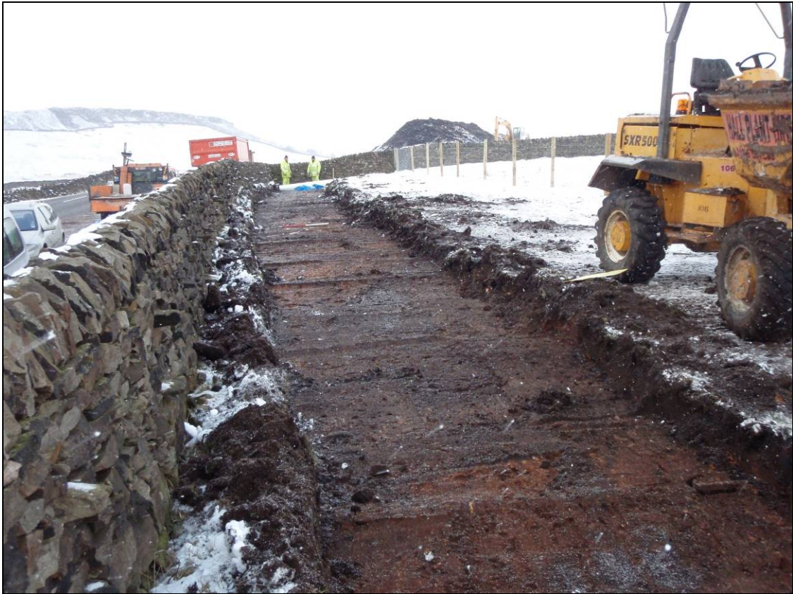
Figure 7: Excavation of the northernmost section of the bridleway, looking north (scale 1m)
