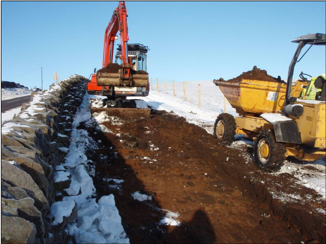
Figure 3: Excavation of the southern section of the bridleway, looking north
