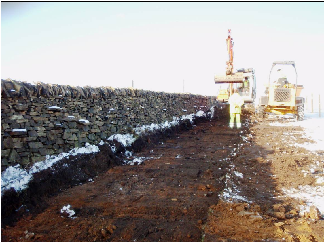
Figure 4: Excavation of the central section of the new bridleway, looking north
