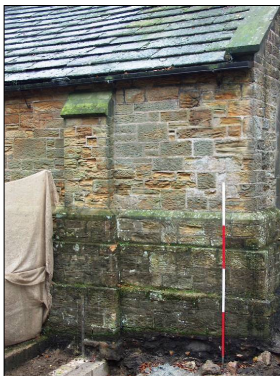
Fig. 7 North wall of the vestry prior to demolition (scale 2m)
