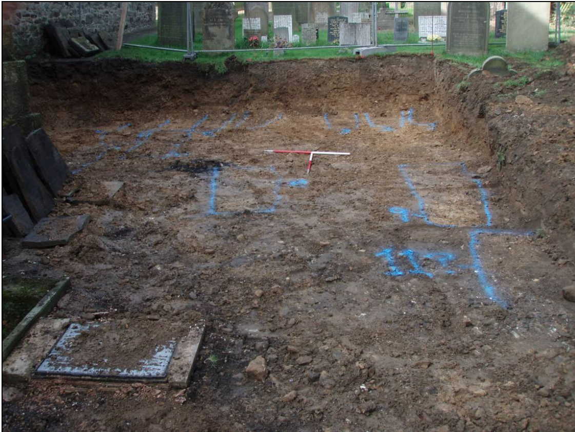
Fig. 4 Excavated area of the proposed building, looking west. Scale = 1m x 2
