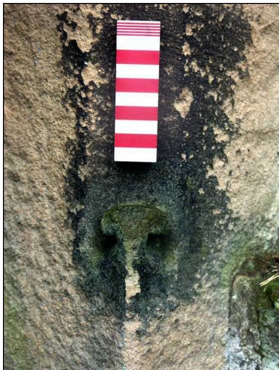
Fig. 10 Detail of chamfer stop (scale 100mm).
