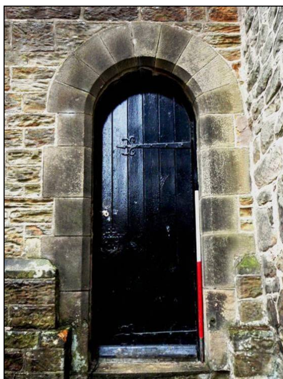
Fig. 9 Detail of doorway (scale 1m).
