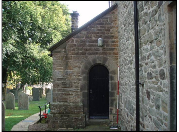
Western elevation of the vestry of the Church of St Lawrence
