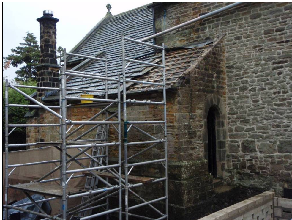
Fig. 16 South-western corner of vestry during demolition, looking south-east.
