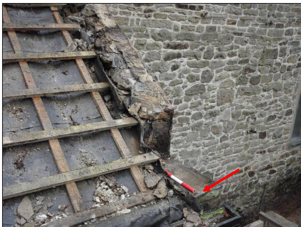
Fig. 17 Grave stone fragment used as masonry indicated with red arrow, looking south-west (scale 300mm).
