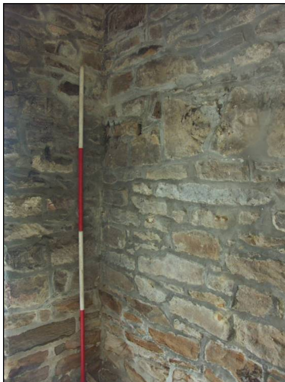
Fig. 14 Sandstone internal wall of the vestry, looking north-west (scale 2m)
