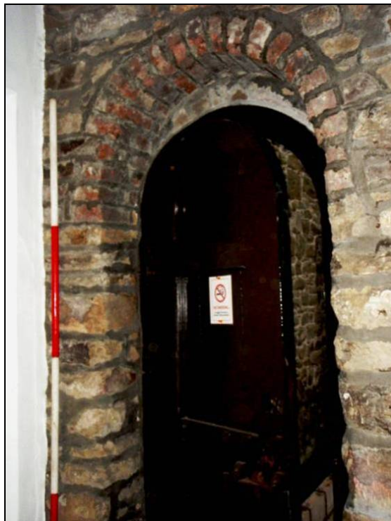
Fig. 15 Doorway with internal brick arched head, looking west (scale 2m).
