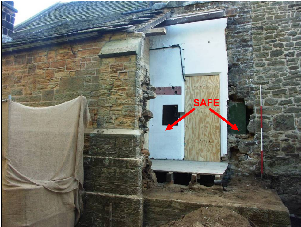
Fig. 24 Completed demolition showing the inserted safes, looking south (scale 2m).
