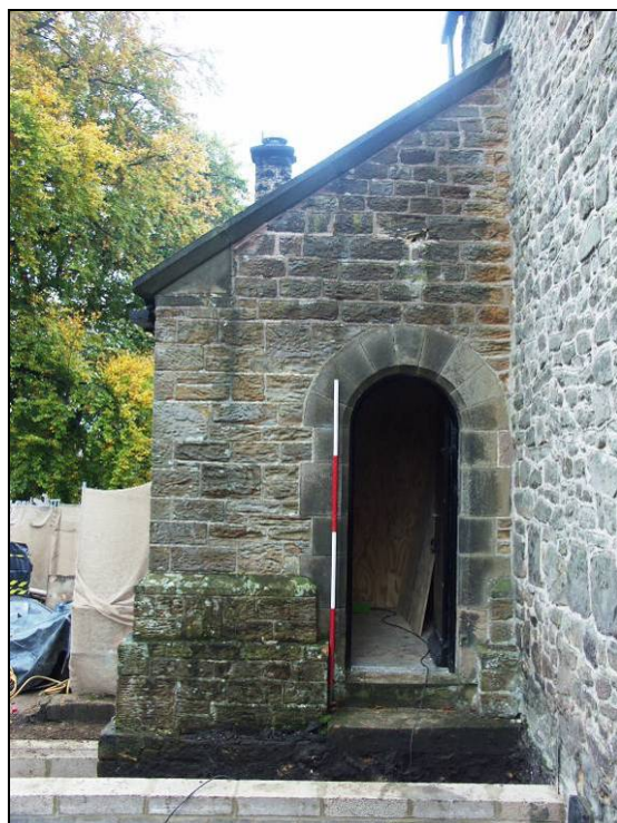
Fig. 8 West wall of the vestry prior to demolition (scale 2m).
