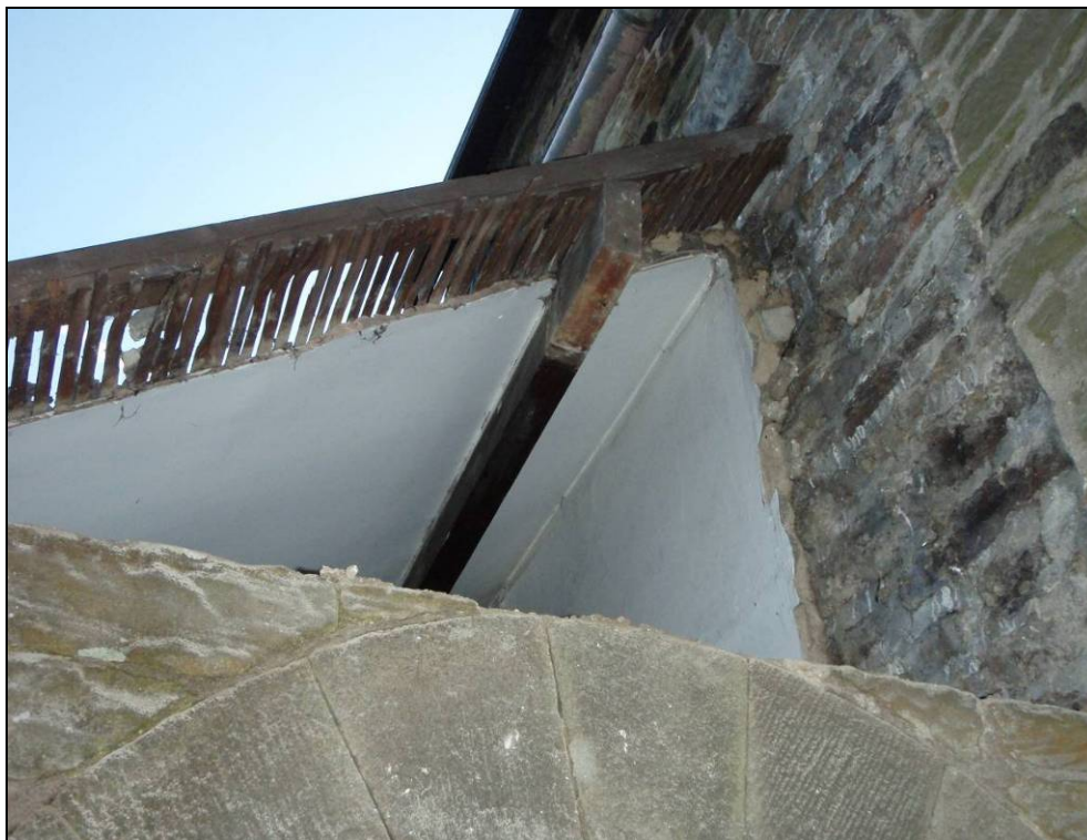
Fig. 20 Detail of ceiling structure during demolition, looking east.
