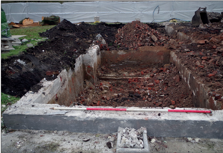
Plate 1: View of foundation walls from the north-east, 2 m scale
