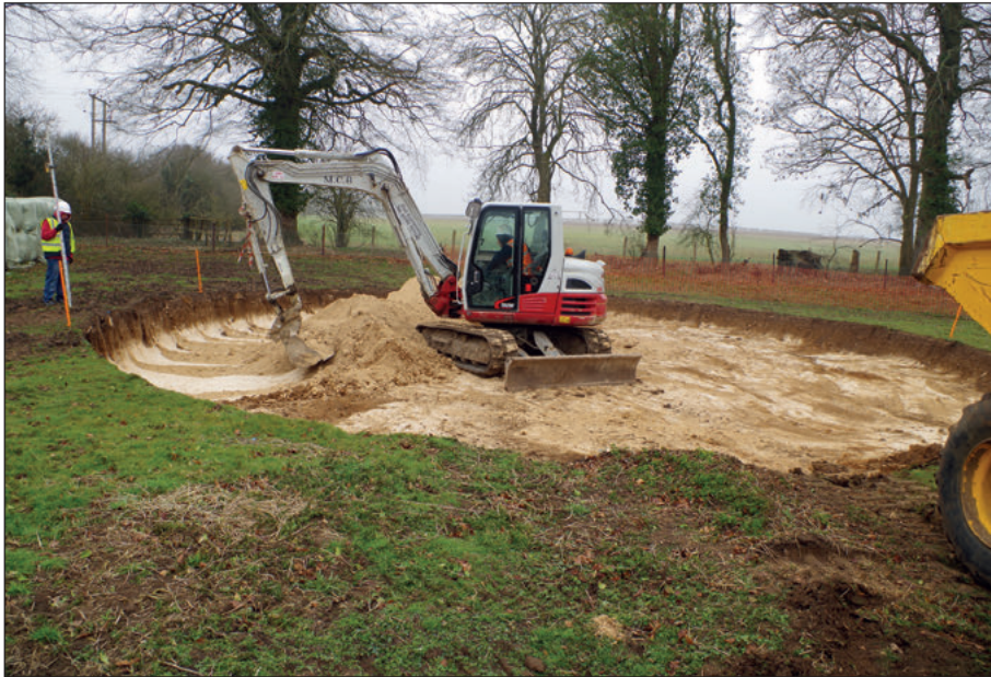
Plate 5: Working shot of TR7, viewed from east
