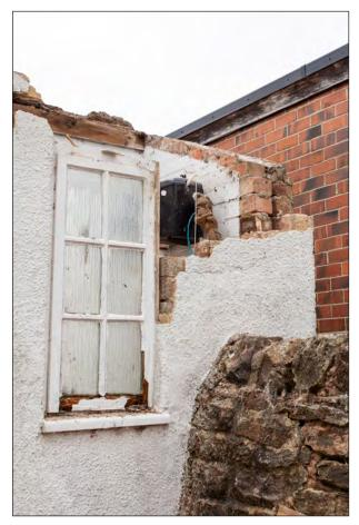
Plate 46 - Outbuilding 1: exposed brickwork of the W.C. extension
