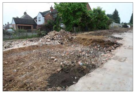
Plate 10 - Area of Whitehouse Farmhouse and stables following demolition to ground level; note the variation in levelling deposits / makeup between the main range (left) and southwest range (yellow sand, centre right)
