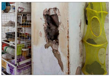
Plate 41 - Outbuilding 1: brick rubble partition wall revealed within the tack room
