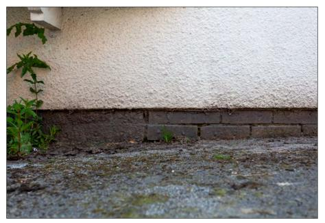
Plate 7 - Detail of the brickwork (and damp proofing) visible at low level around the farmhouse
