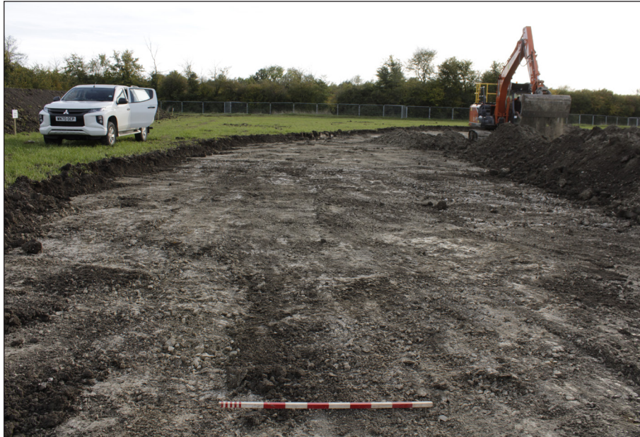
Figure 4: Working shot – subsoil stripping within Area 3 viewed from the north
