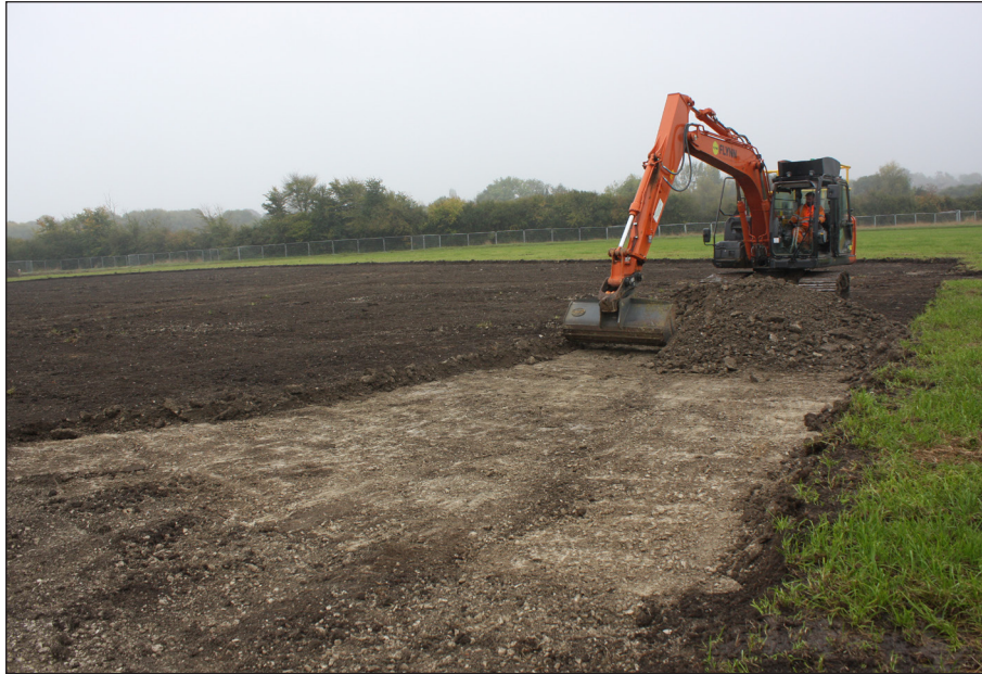
Figure 3: Working shot – subsoil stripping within Area 3 viewed from the north-west
