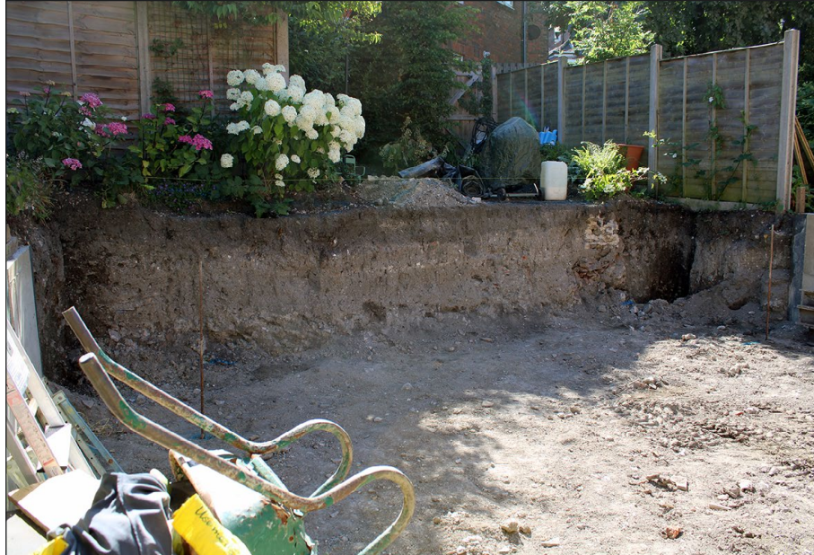
Figure 5: Fully excavated area, view from the north-west
