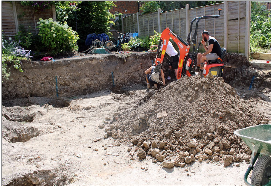
Figure 6: Excavation of beam holes, view from the north-west
