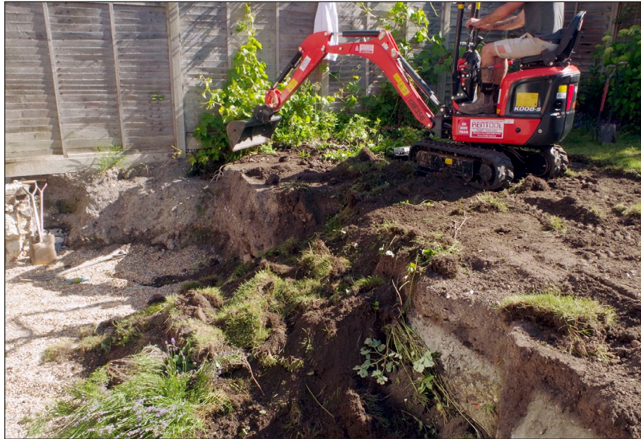
Figure 4: Initial excavations, view from the south
