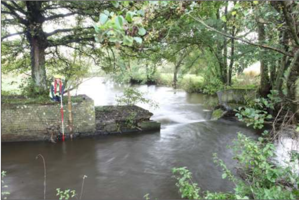
Plate 1: The weir structure viewed from the north-west prior to demolition
