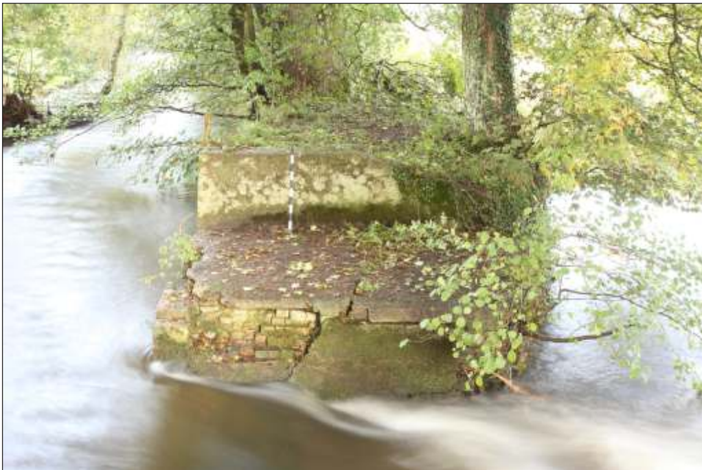
Plate 2: The east bank of the weir structure prior to demolition
