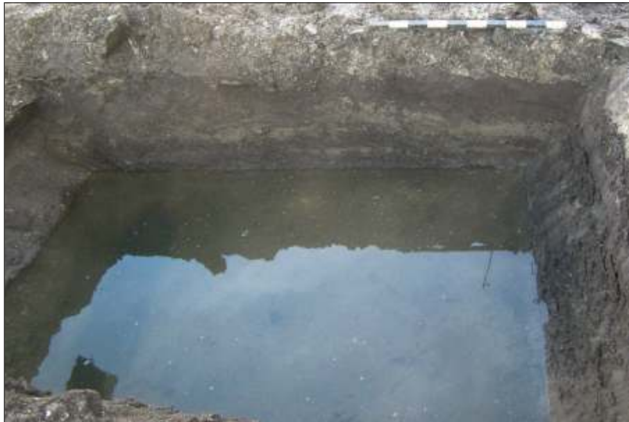
Plate 21: Representative levee construction section trench with submerged culvert to the left
