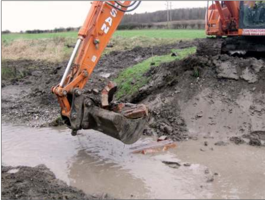
Plate 23: Culvert removal in progress and brick construction detail
