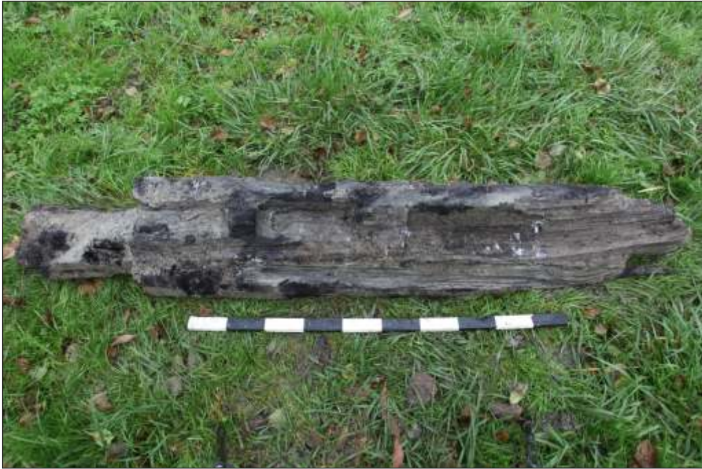
Plate 11: Timber 1 recovered from beneath the east bank, west wall of the weir structure with several carpentry joints including mortises and tenons and a groove along its length
