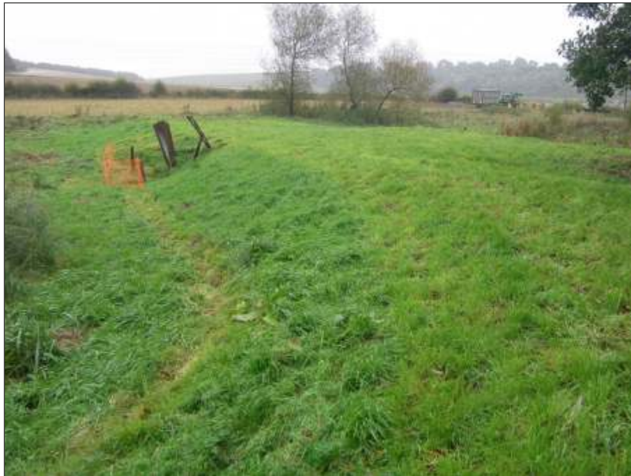
Plate 17: Entrance of culvert viewed from the south
