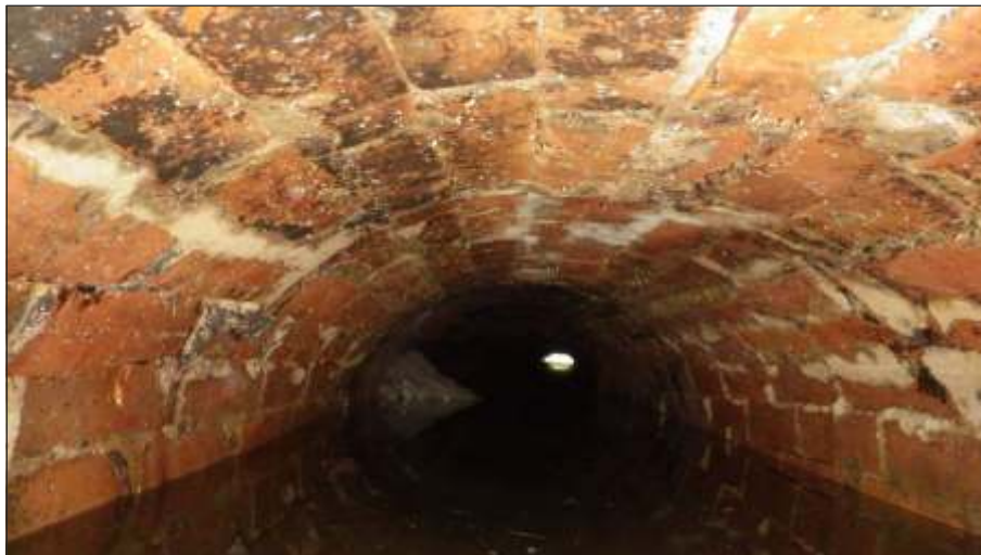
Plate 19: Interior of the culvert showing brick vault
