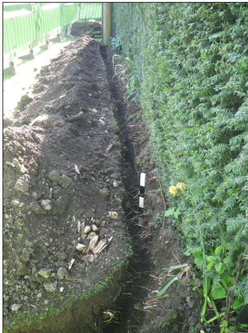
Plate 2: Southern section of trench from support pole to road; garden soil (03)
