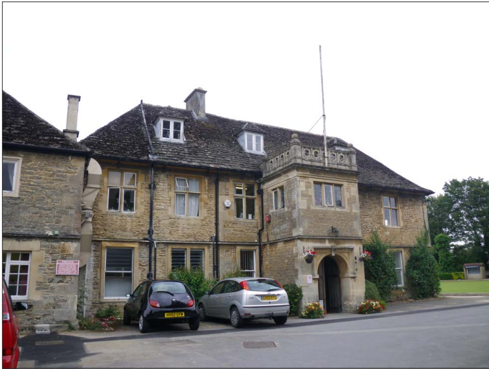
Plate 1: Melksham House, view from south-east
