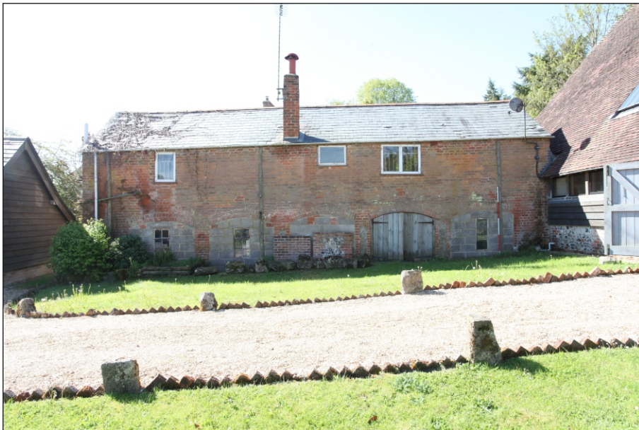
Plate 12: Drax Cottage north elevation showing blocked pigsty entrances and inserted first floor windows
