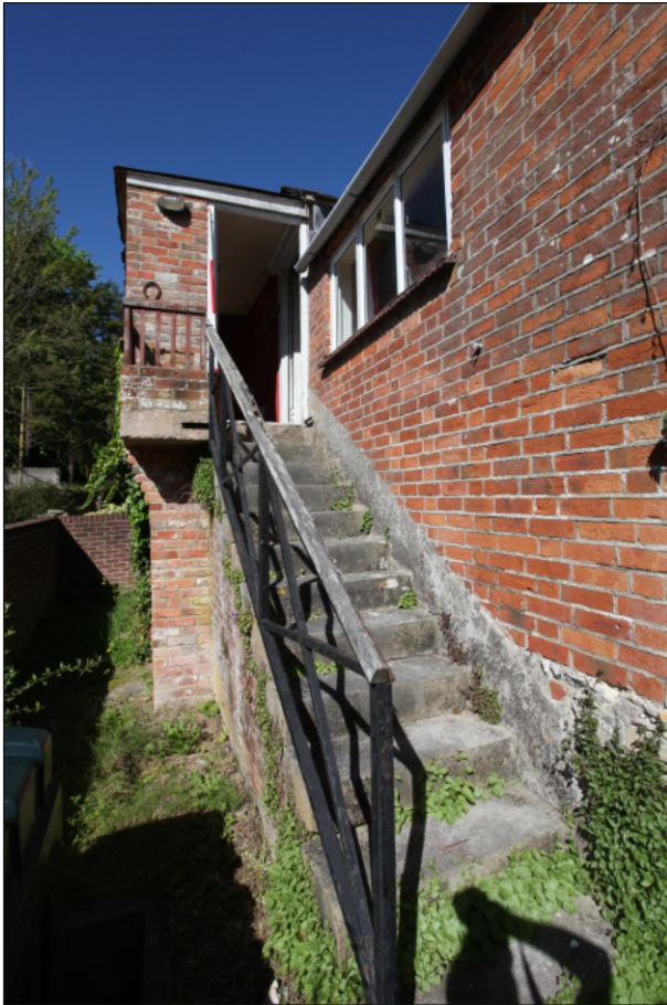
Plate 15: Drax Cottage south elevation showing access stairs and first floor porch
