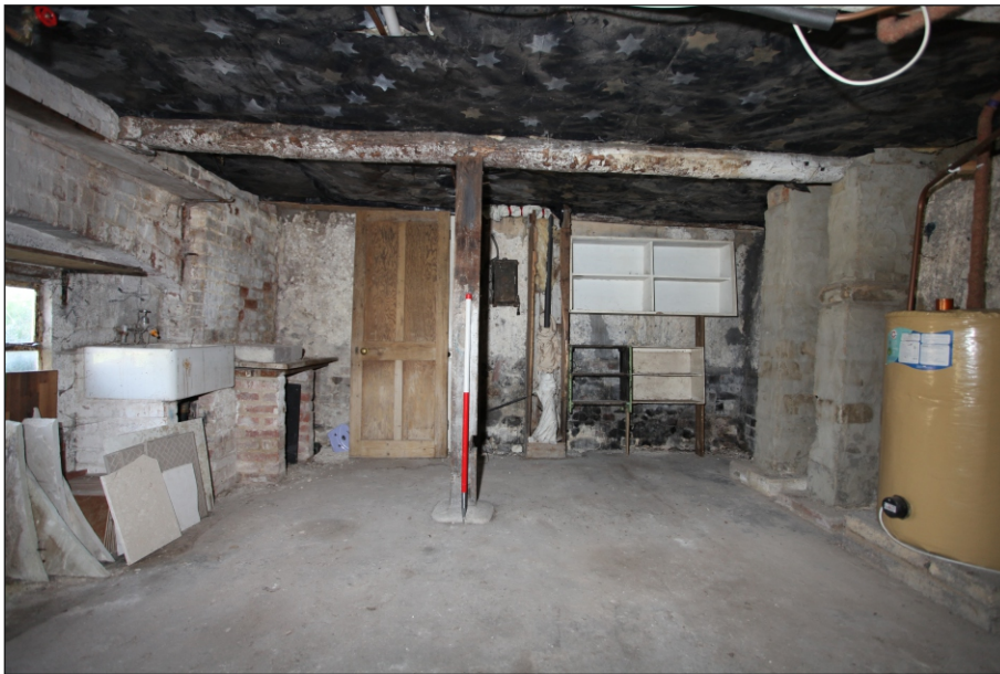
Plate 24: Drax Cottage east wall showing cob walling
