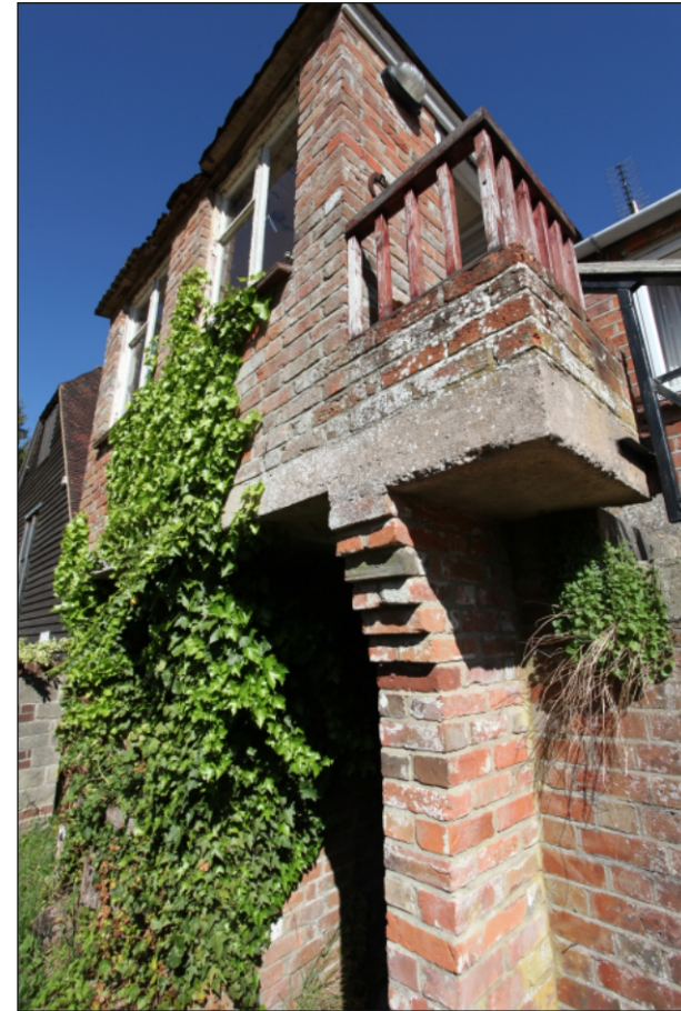
Plate 16: Drax Cottage south porch platform and supports
