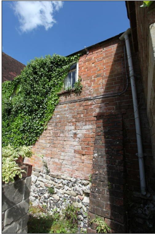
Plate 17: Drax Cottage south wall west end showing brickwork and applied buttress
