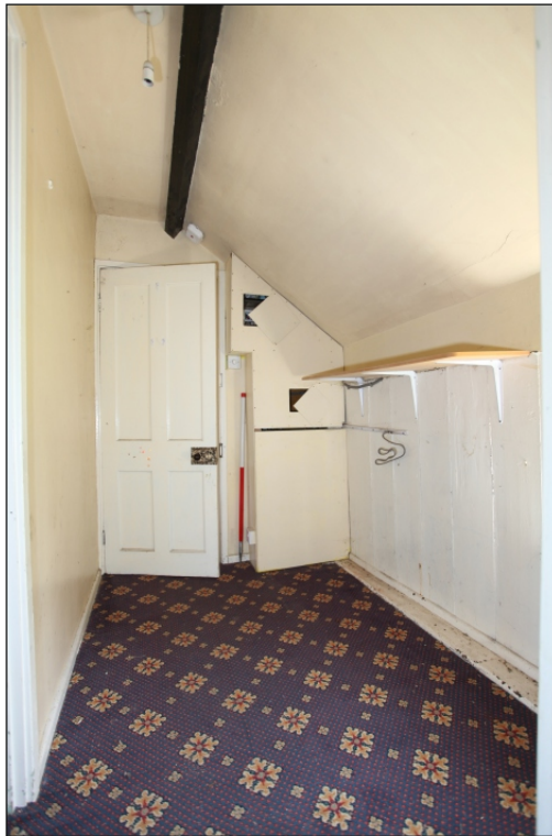
Plate 29: Drax Cottage first floor lobby showing wainscoting along south wall
