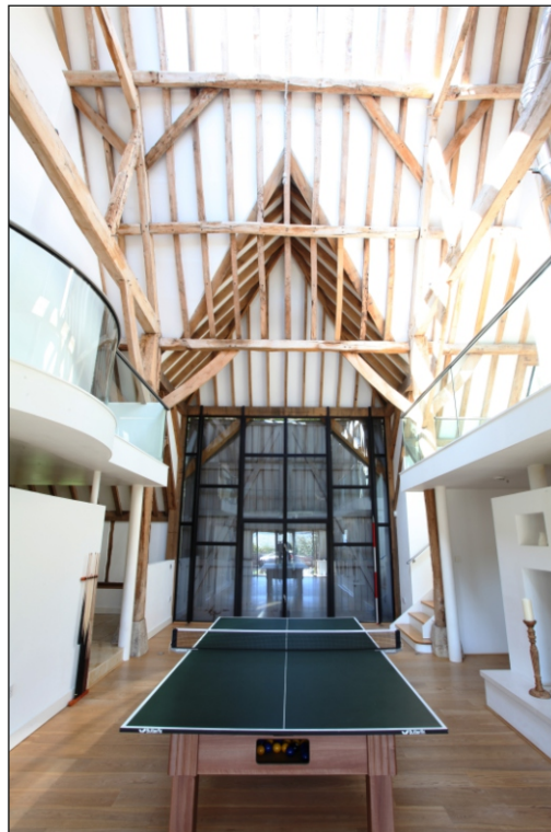
Plate 4: Drax Barn general view of ground floor center
