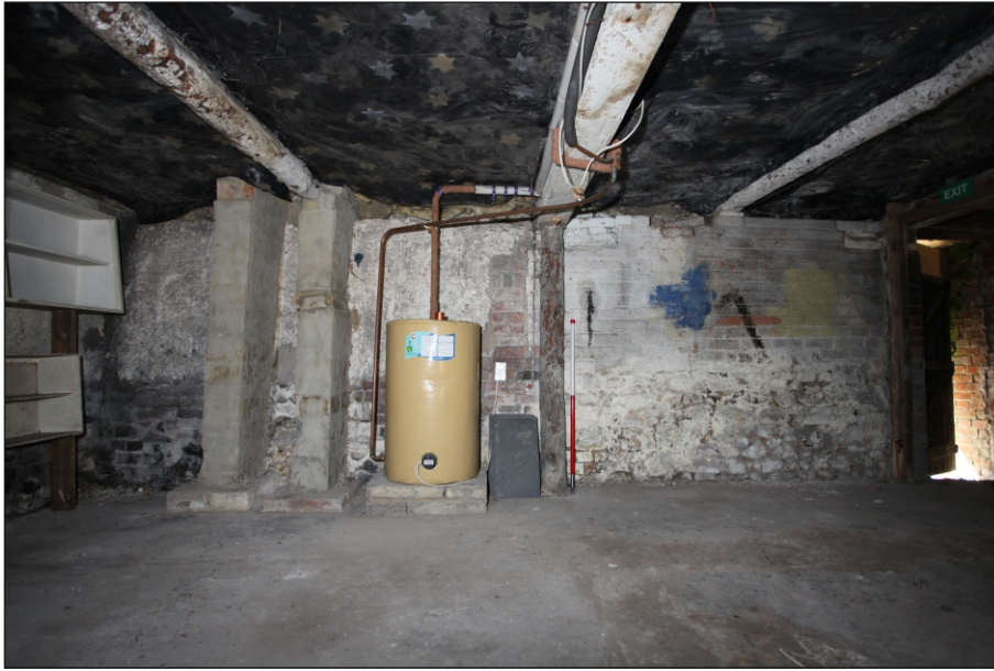
Plate 25: Drax Cottage south wall showing cob walling
