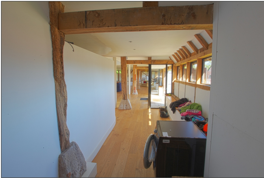
Plate 7: View along east aisle showing aisle posts and aisle ties
