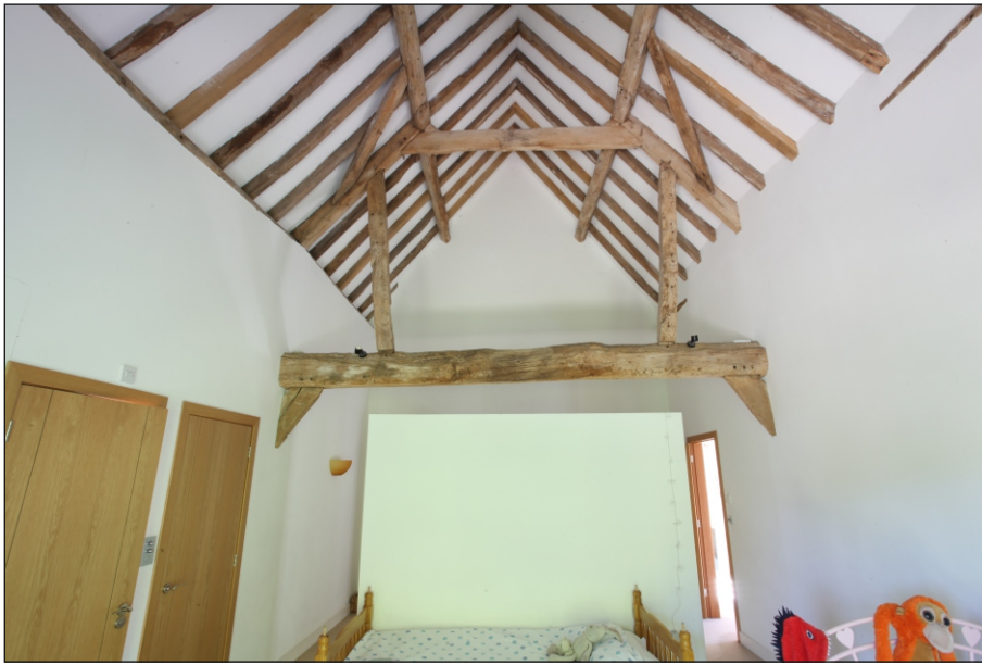
Plate 11: Drax Barn north end roof viewed from north
