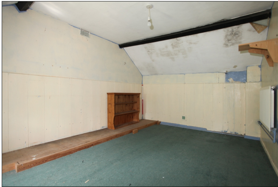
Plate 31: Drax Cottage first floor west bedroom showing wainscoting along north and west walls
