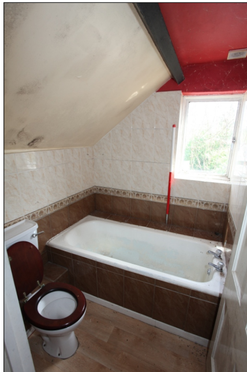
Plate 28: Drax Cottage first floor bathroom east end
