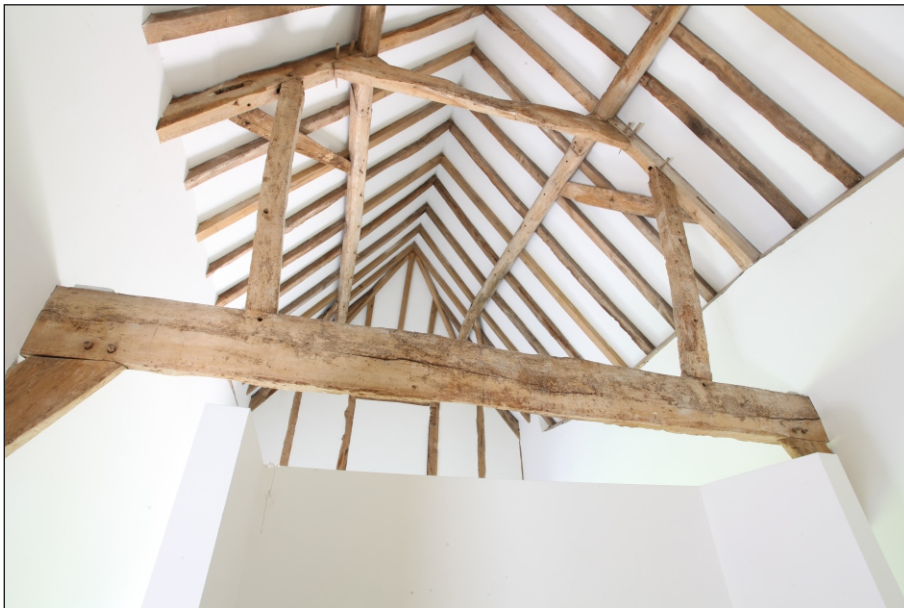
Plate 10: Drax Barn north end roof viewed from south
