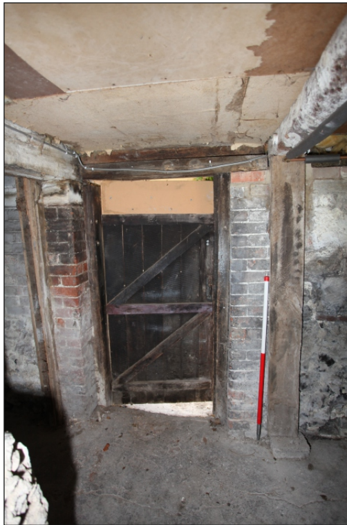
Plate 21: Drax Cottage south door entrance viewed from interior
