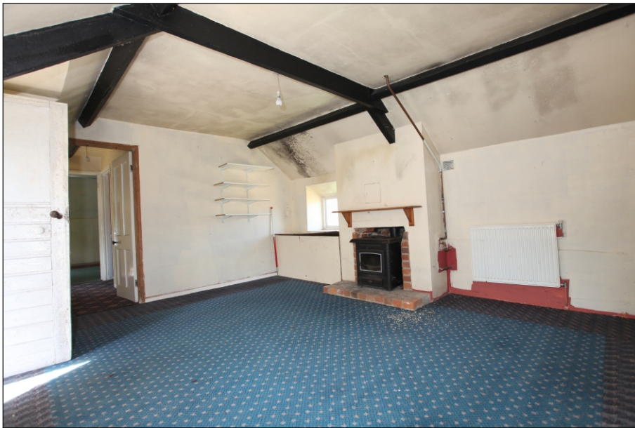
Plate 26: Drax Cottage first floor living room also showing exposed roof timbers
