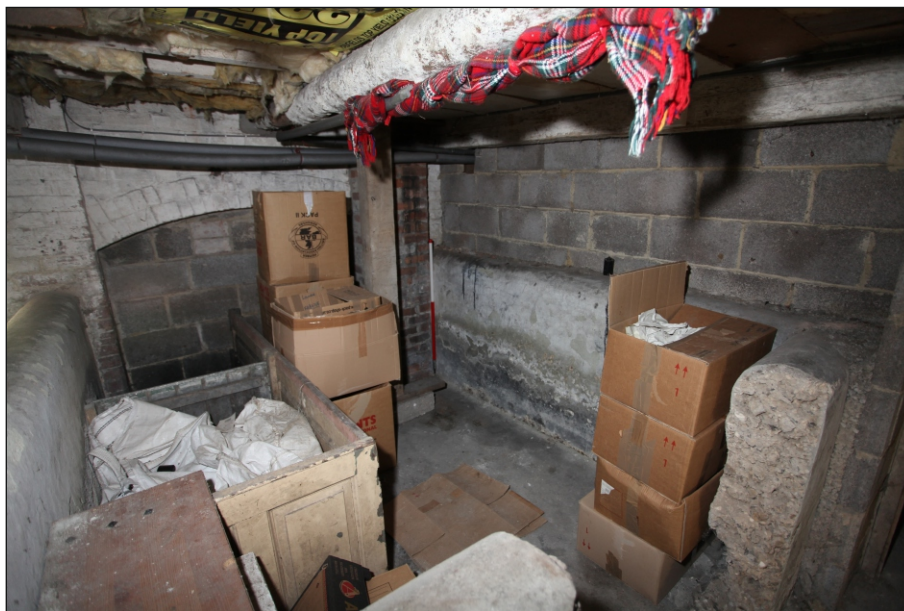
Plate 22: Drax Cottage concrete block dividing wall
