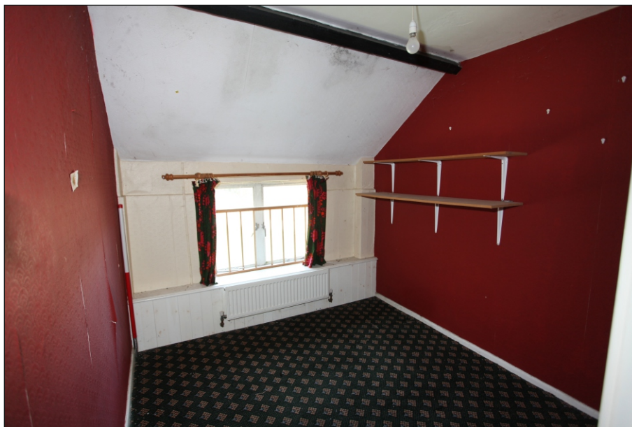
Plate 30: Drax Cottage first floor north bedroom showing wainscoting along north wall
