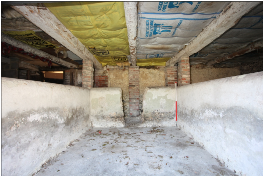
Plate 20: Drax Cottage typical pigsty and supporting beams to first floor
