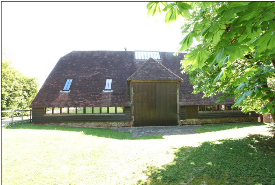
Plate 2: Drax Barn viewed from west showing mid-strey porch
