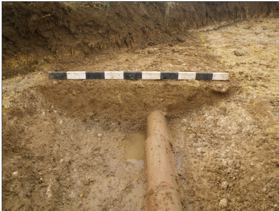
Plate 6: North-east facing section of land drain bearing ditch 504
