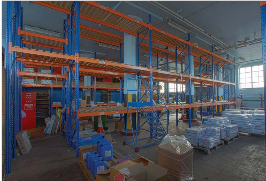
Plate 6: WD 0 040 ground floor storage space with concrete column framework viewed from the north.
