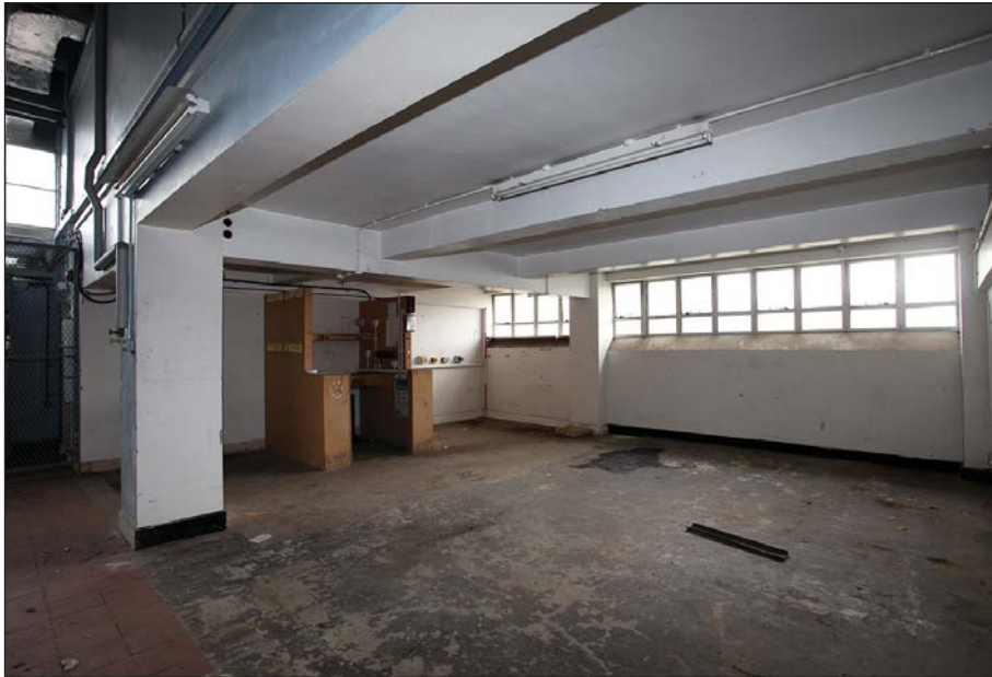
Plate 11: WD 0 040 ground floor. Workshop area after clearance.
