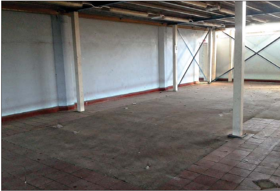
Plate 13: WD 0 040 ground floor. Oven room untiled floor surface that marks the location of the oven.
