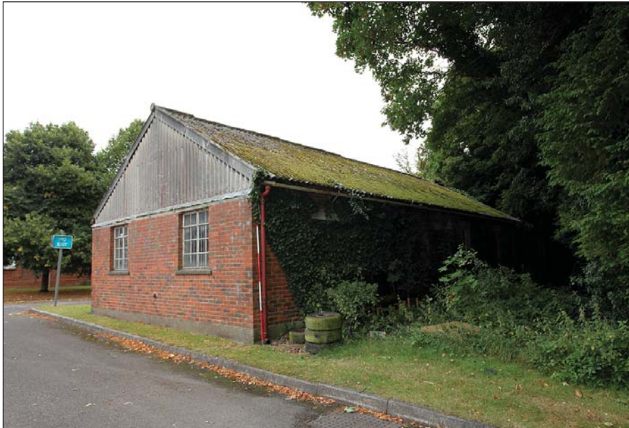
Plate 86: WI 0 218 viewed from the north.
