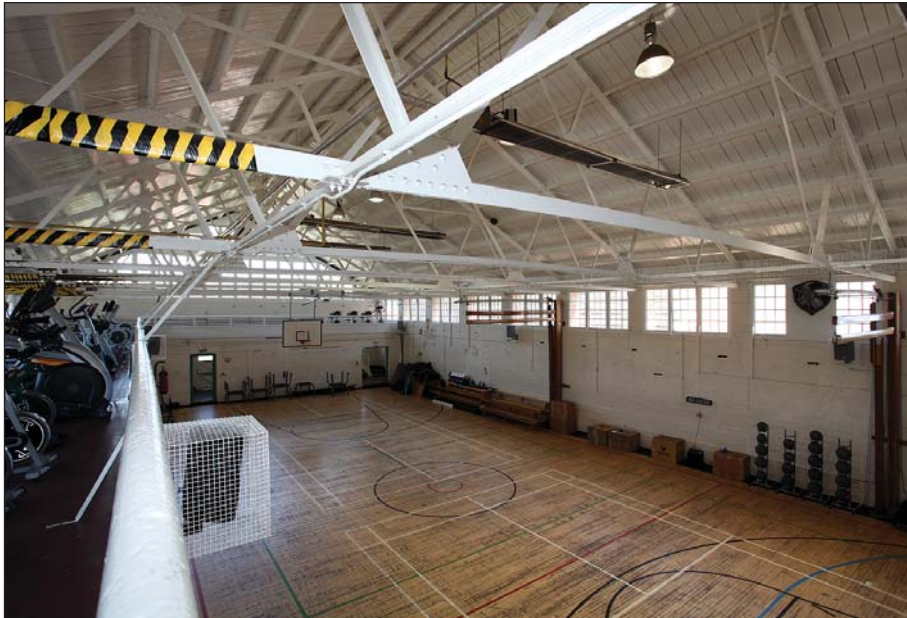
Plate 116: First floor gallery overlooking the sports hall, viewed from the west.
