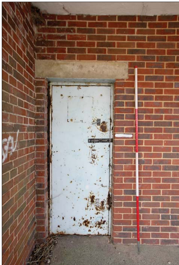
Plate 98: WI 0 235 metal security door at the north end of the building.
