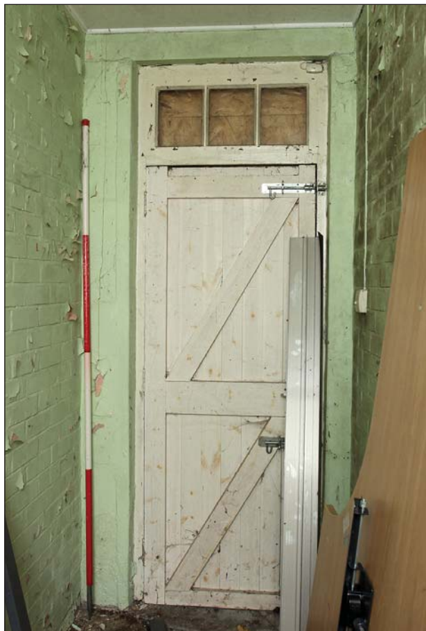
Plate 88: WI 0 218 internal face of the rear access door.
