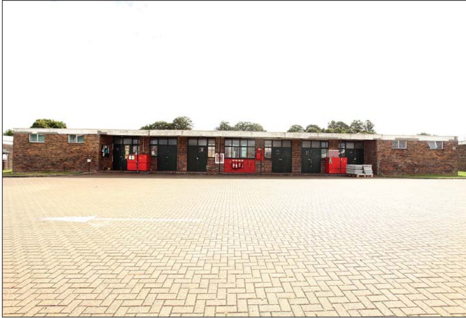
Plate 57: WI 0 207 viewed from the north-west.
