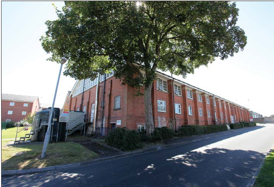
Plate 106: KW 0 415 viewed from the north.
