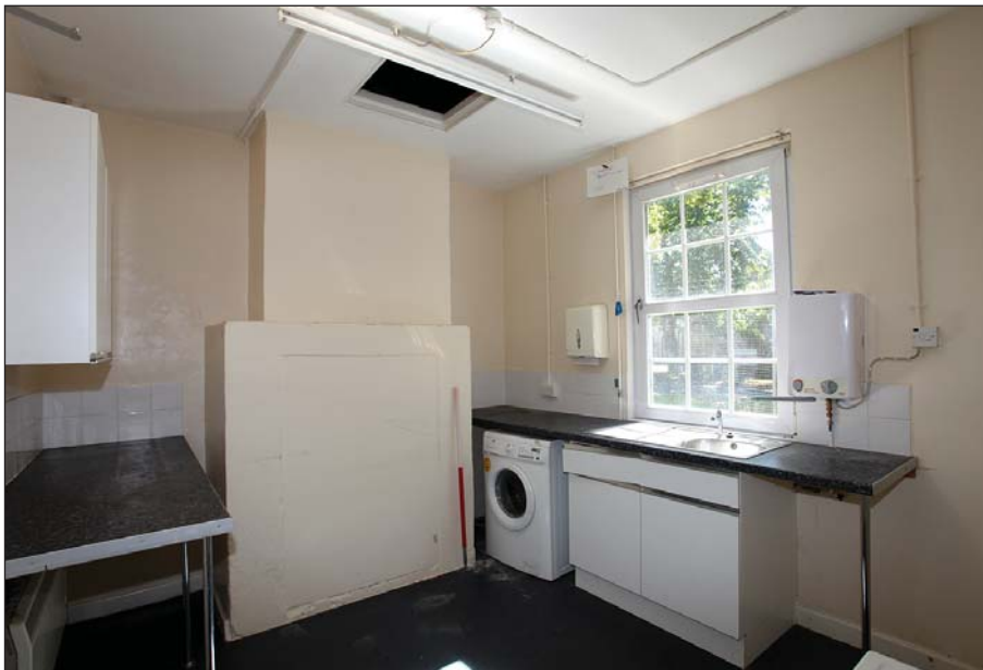
Plate 130: PC 0 707 kitchen viewed from the north.
