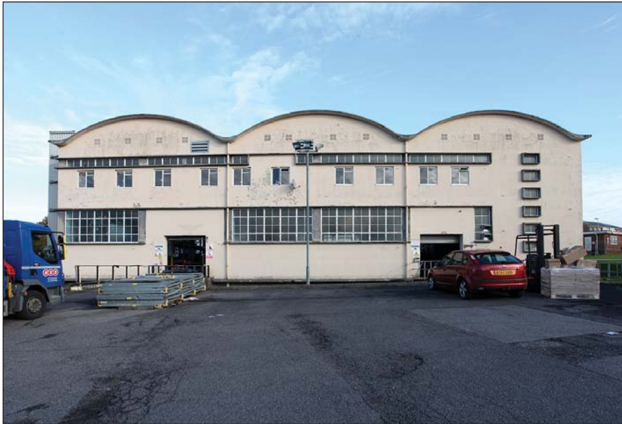
Plate 3: WD 0 040 south-west (rear) elevation.
