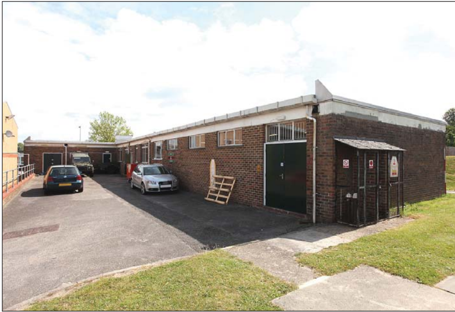
Plate 51: WI 0 206 and WI 0 830 viewed from the south-west.
