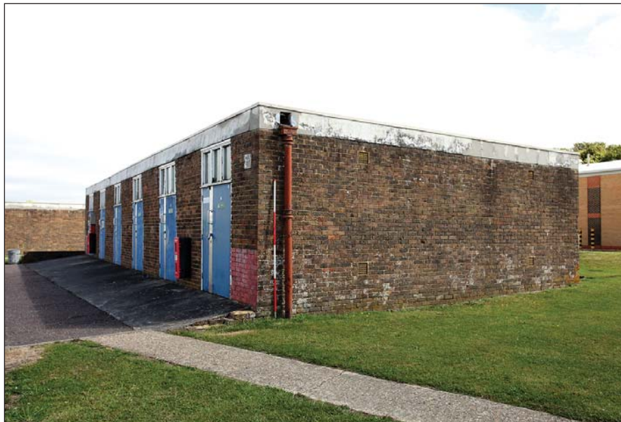
Plate 68: WI 0 209 viewed from the west.
