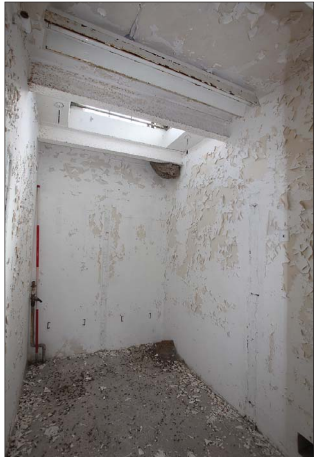
Plate 104: WI 0 235 smallest store room in the south area. Note the vertical scars on the walls that mark the position of removed shelving partitions.
