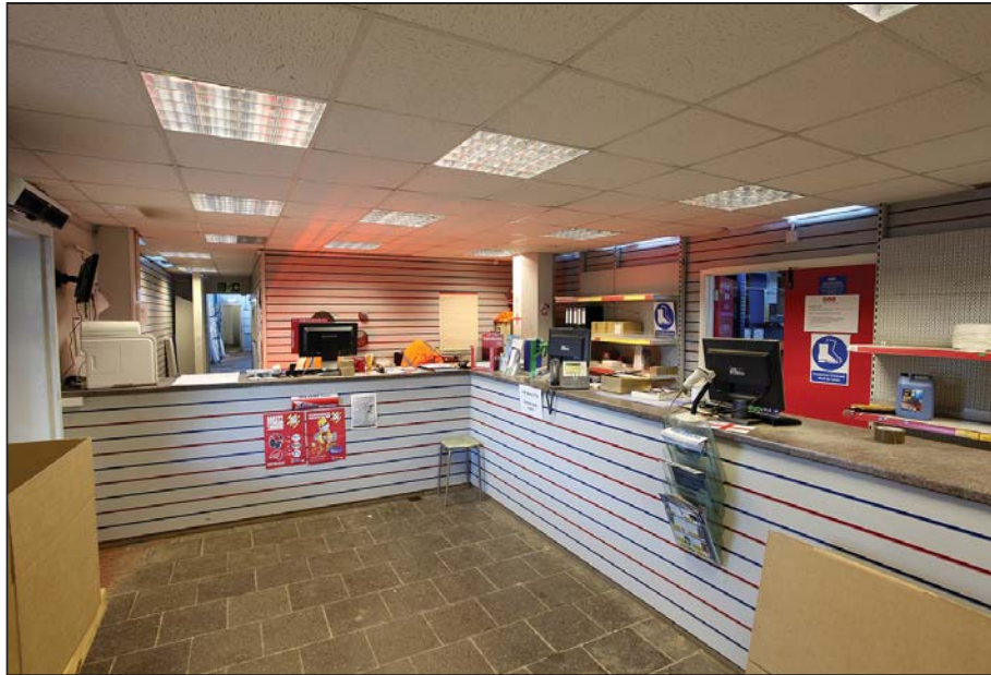
Plate 5: WD 0 040 ground floor reception area viewed from the north showing the later partition walls and ceiling around the original concrete column framework.
