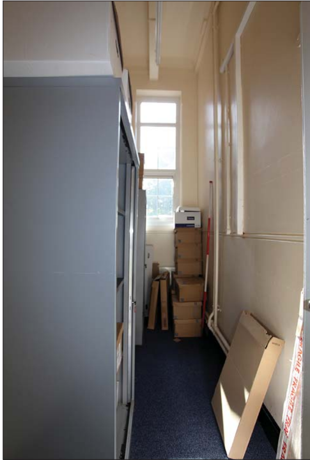
Plate 47: WI 0 082 archives (0.3), former Coats and Hats room. Note the chamfered window opening and flushed bead at dado level.
