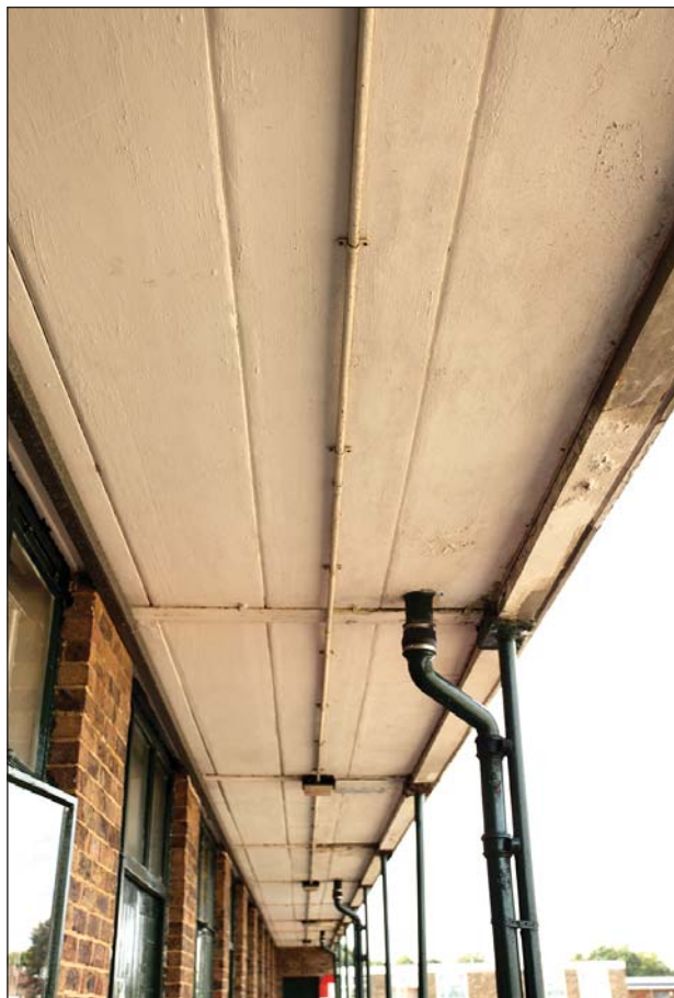
Plate 62: WI 0 208 verandah ceiling.
