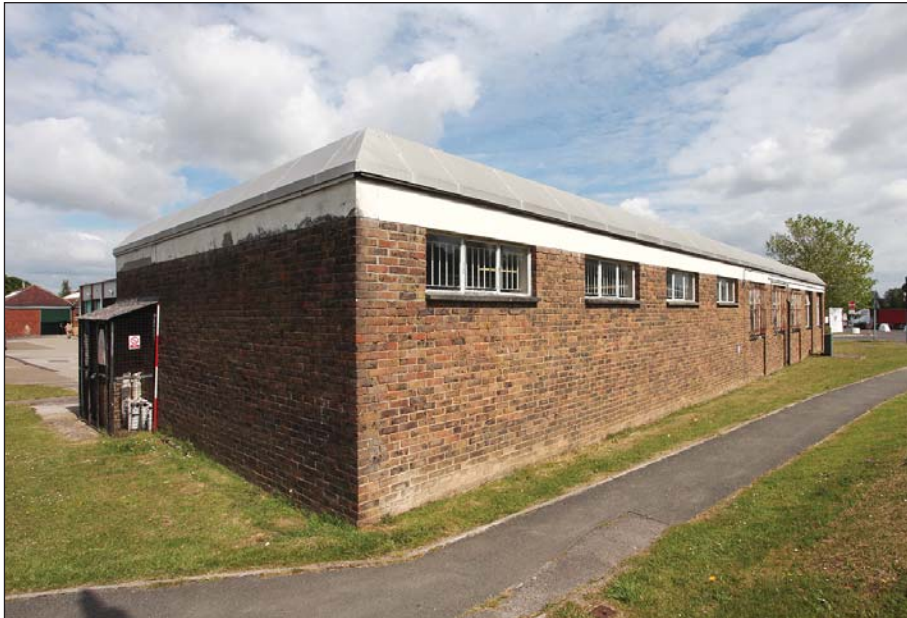
Plate 52: WI 0 206 and WI 0 830 viewed from the south.
