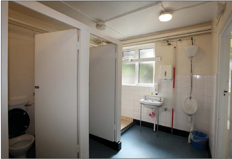
Plate 81: WI 0 216 ablutions room viewed from the north.
