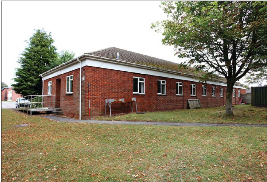
Plate 72: WI 0 216 viewed from the west.
