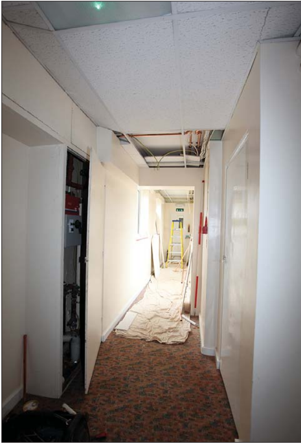
Plate 76: WI 0 216 secondary and link corridor viewed from the south-west.
