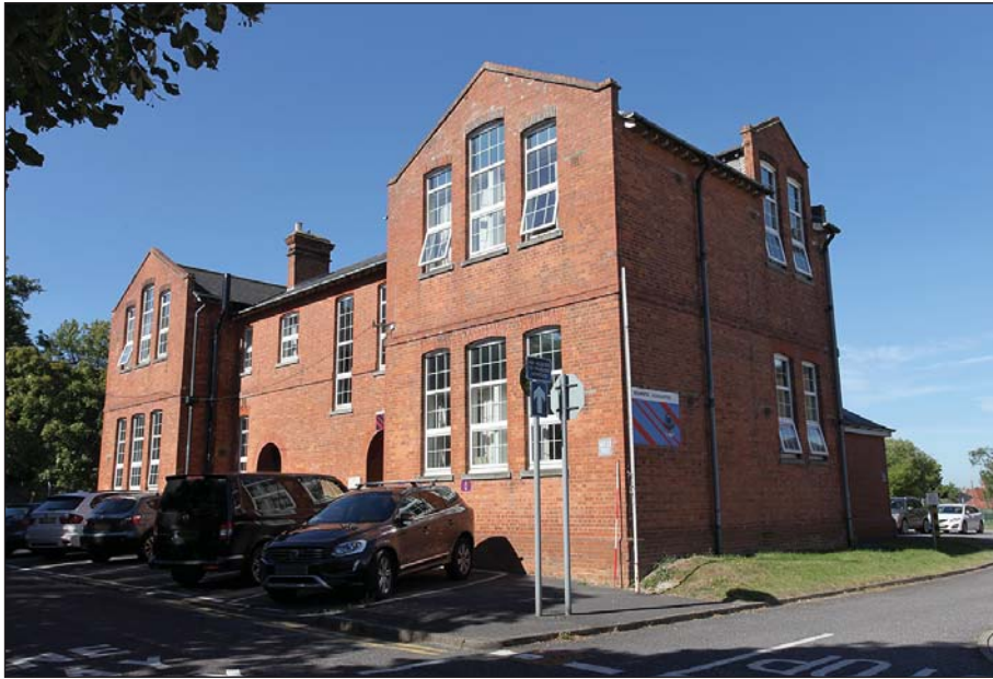
Plate 27: WI 0 082 RMP HQ viewed from the east.
