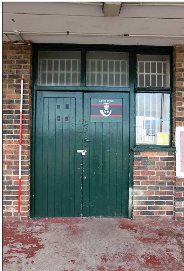
Plate 58: WI 0 207 door and windows detail.
