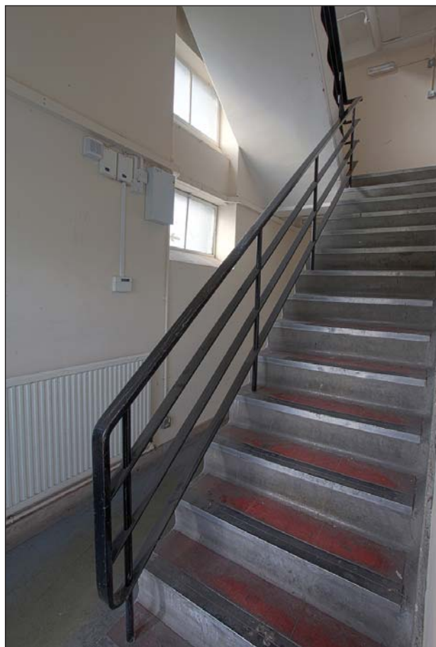
Plate 10: WD 0 040 ground floor. South corner stairwell. It contains its original staircase and column of windows.
