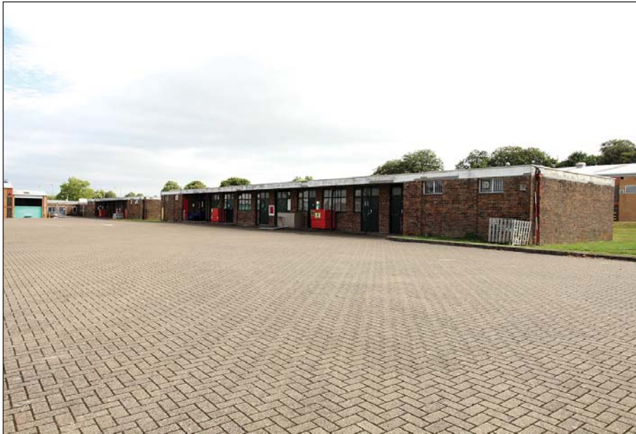
Plate 64: WI 0 208 viewed from the south-west. WI 0 207, WI 0 206 and WI 0 830 are in the background.
