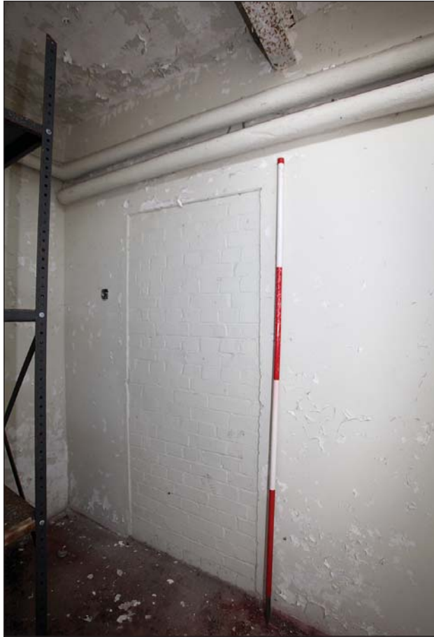
Plate 101: WI 0 235 the blocked door opening between the north and south areas
