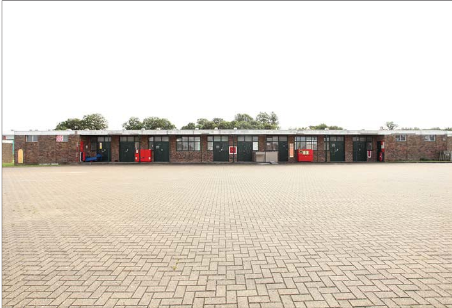
Plate 61: WI 0 208 viewed from the north-west.
