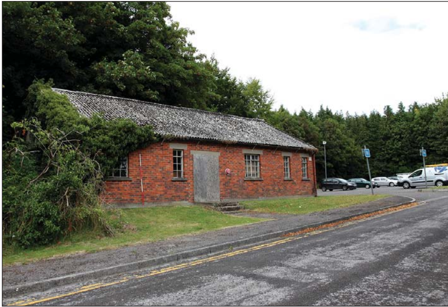
Plate 85: WI 0 218 and car park viewed from the south.
