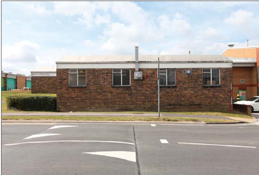
Plate 54: WI 0 206 and WI 0 830 north-east elevation viewed from the north-east.
