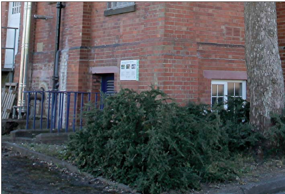
Plate 110: KW 0 415 north corner showing the basement stairs and window.
