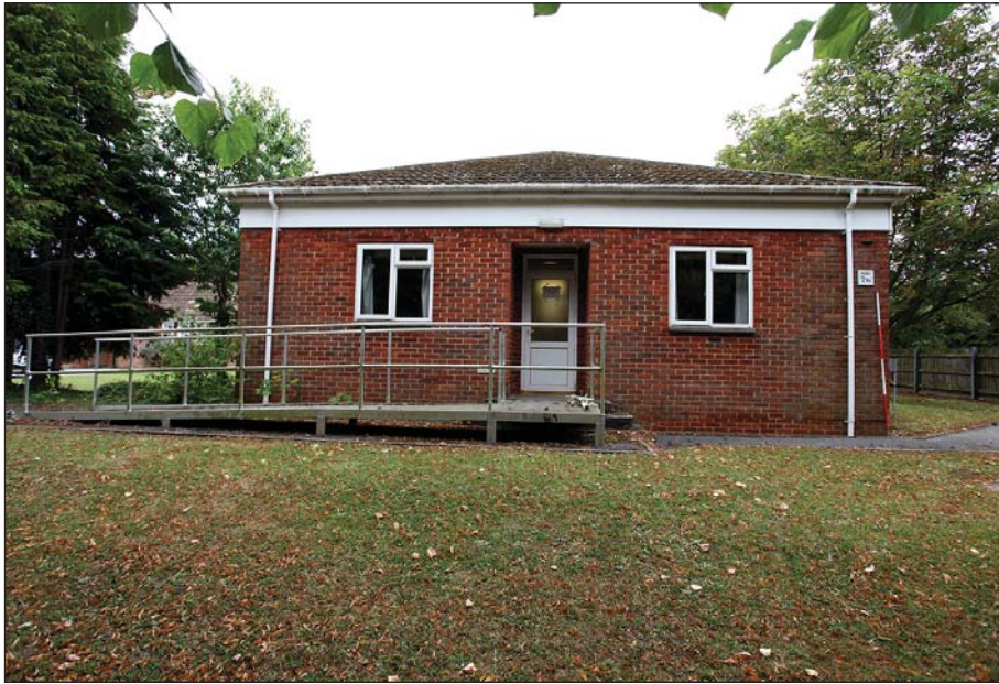
Plate 71: WI 0 216 viewed from the north-west.
