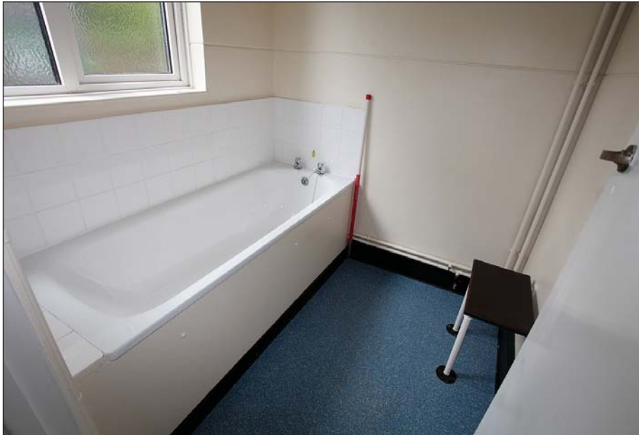
Plate 82: WI 0 216 bath in ablutions room 10 viewed from the east. The incised line at dado level and seat appear to be original.
