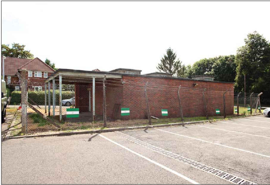
Plate 95: WI 0 235 viewed from the north-west.
