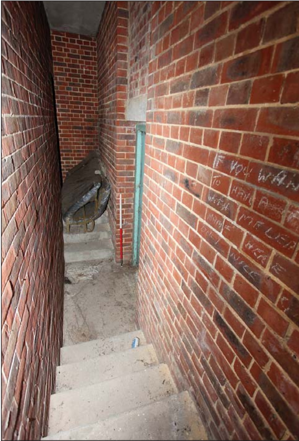
Plate 103: WI 0 235 rear entrance block viewed from the north-west.
