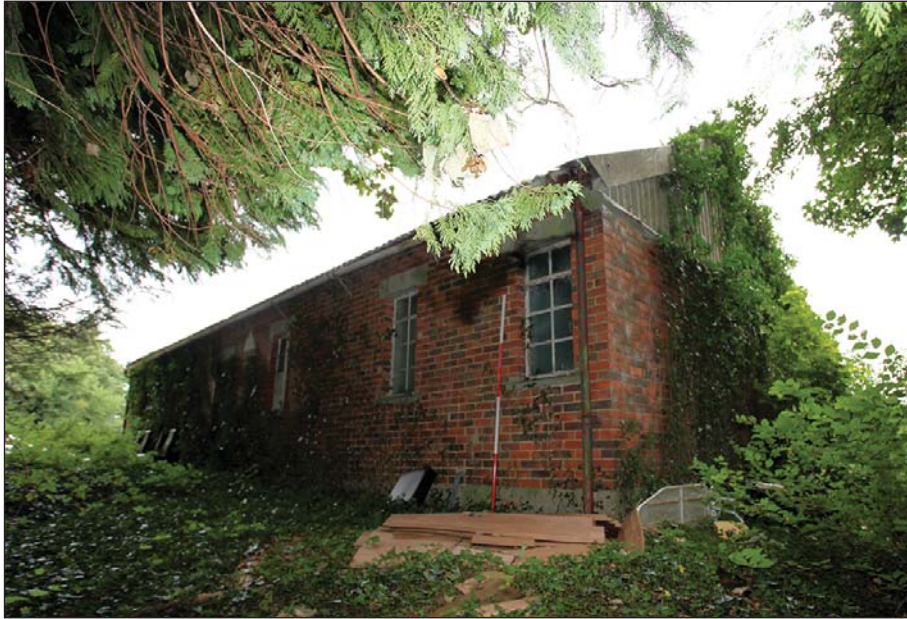
Plate 87: WI 0 218 viewed from the west.
