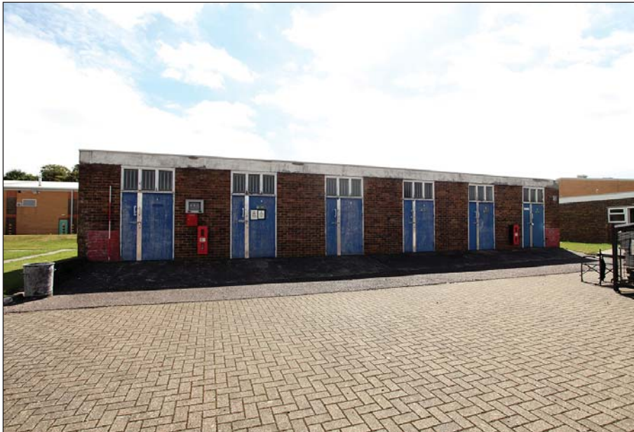
Plate 66: WI 0 209 viewed from the north-west.
