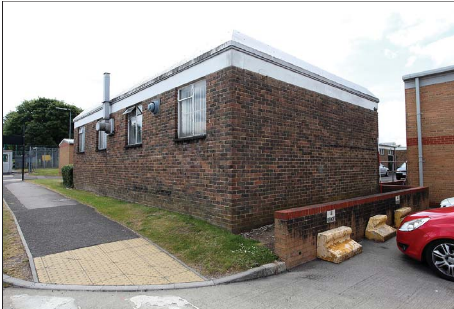
Plate 55: WI 0 206 and WI 0 830 viewed from the north-west.
