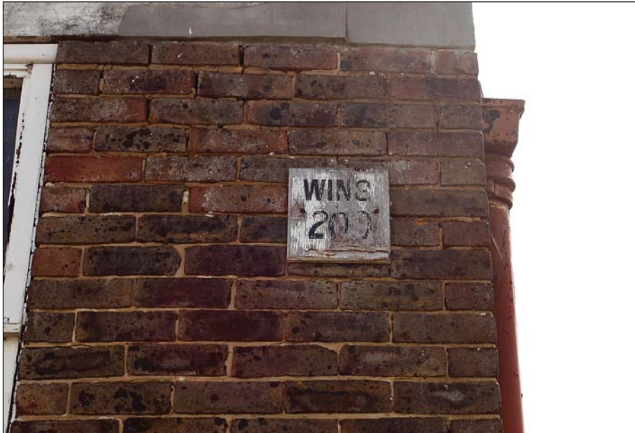
Plate 70: WI 0 209 sign 'WING 209' fixed to the west corner of the building.
