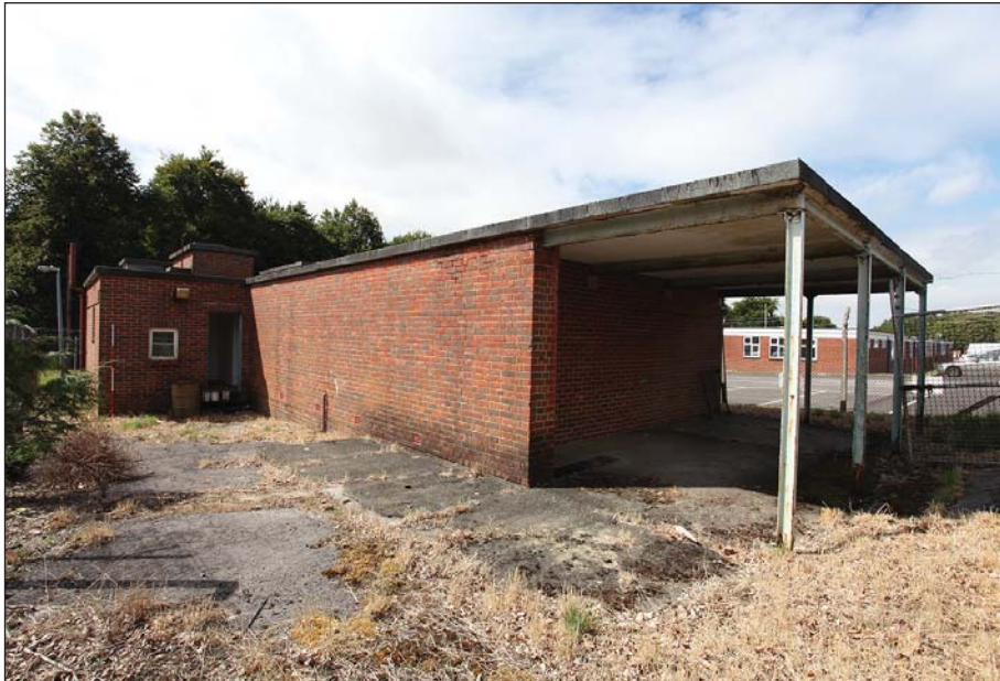
Plate 96: WI 0 235 viewed from the north-east.
