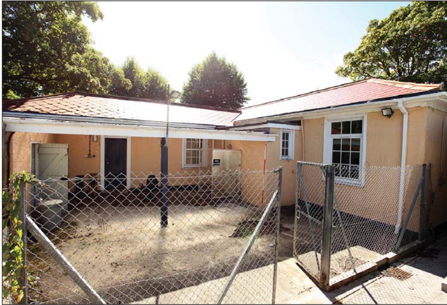
Plate 121: PC 0 707 viewed from the east. The north-east side of the building and south end of the yard are shown.
