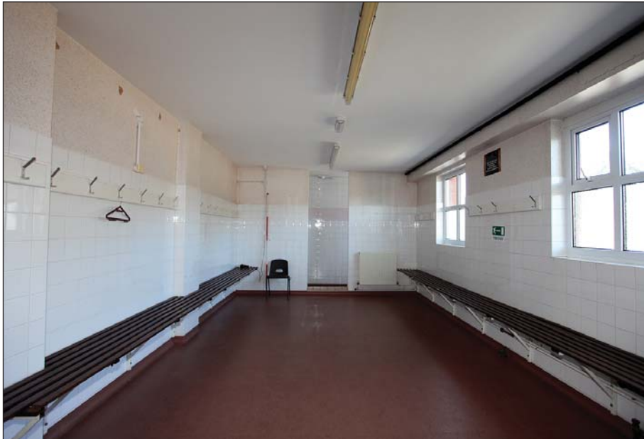
Plate 114: KW 0 415 changing room viewed from the north-east.
