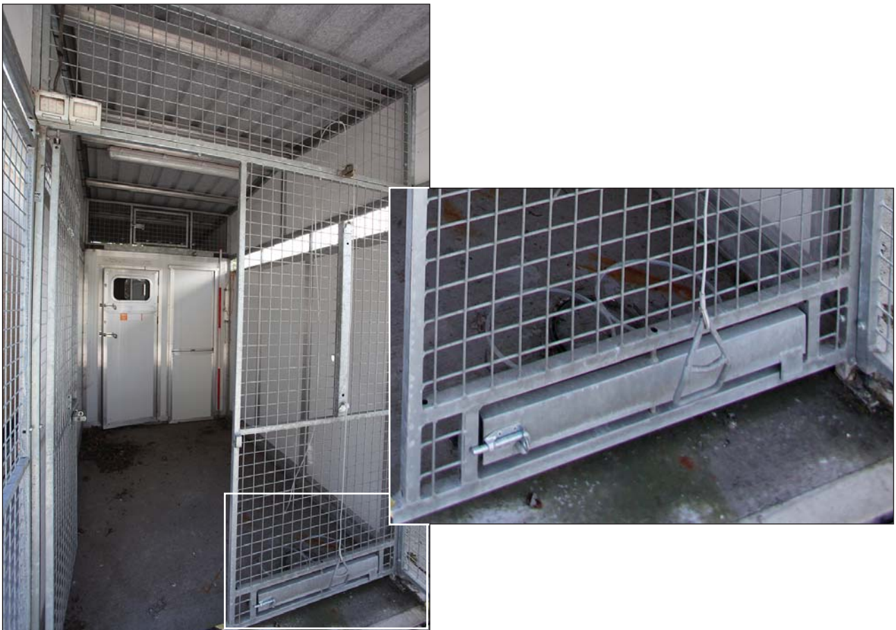
Plate 124: PC A 707 kennel bay. Note the rotating food hatch (inset) and pulley system for the sleeping enclosure hatch (right).
