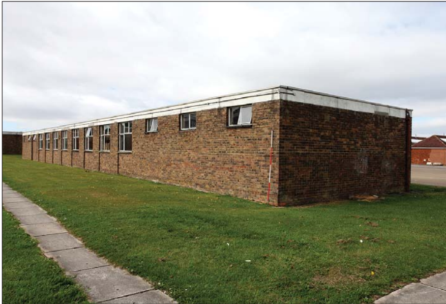
Plate 63: WI 0 208 viewed from the north-east.
