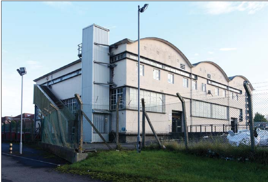
Plate 4: WD 0 040 viewed from the west showing the external lift and stair towers on the north-west elevation.
