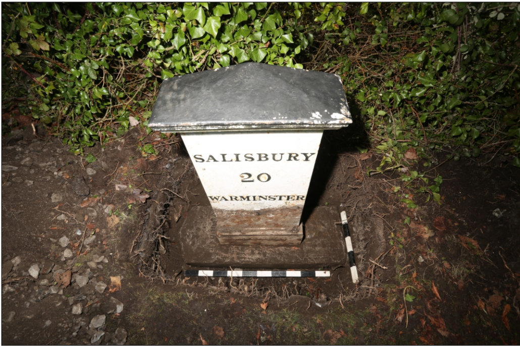
Plate 3: The milepost and milestone beneath it fully exposed prior to lifting
