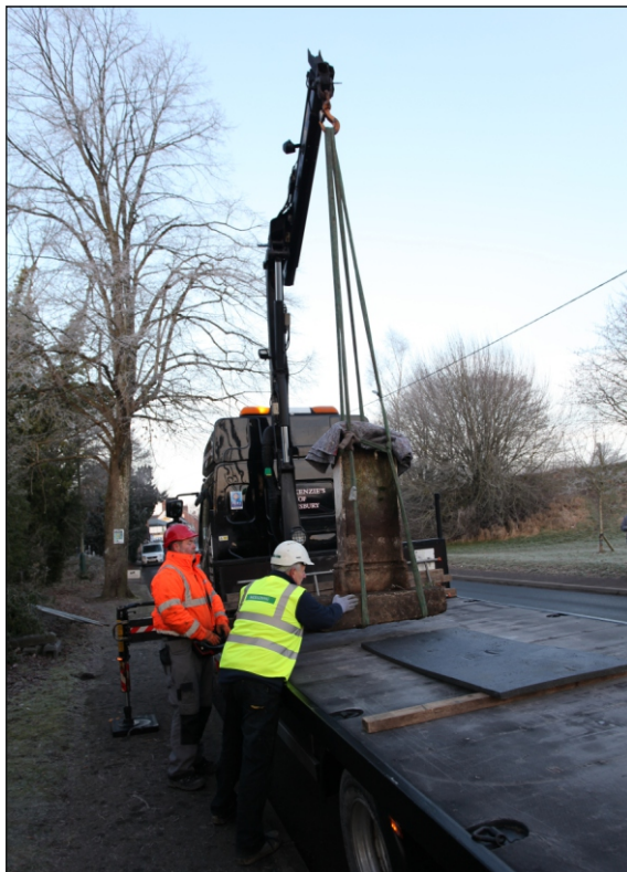
Plate 5: Lifting of the milepost and milestone
