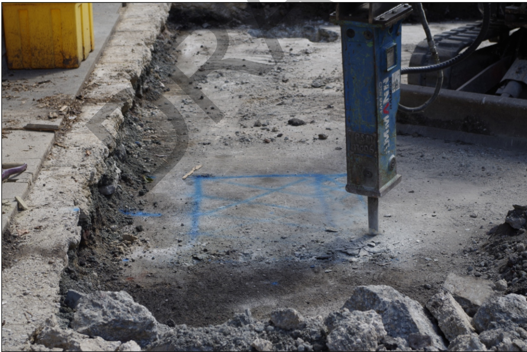
Plate 4: Breaking out concrete slab in piling locations
