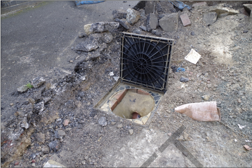
Plate 3: Modern drainage in concrete slab
