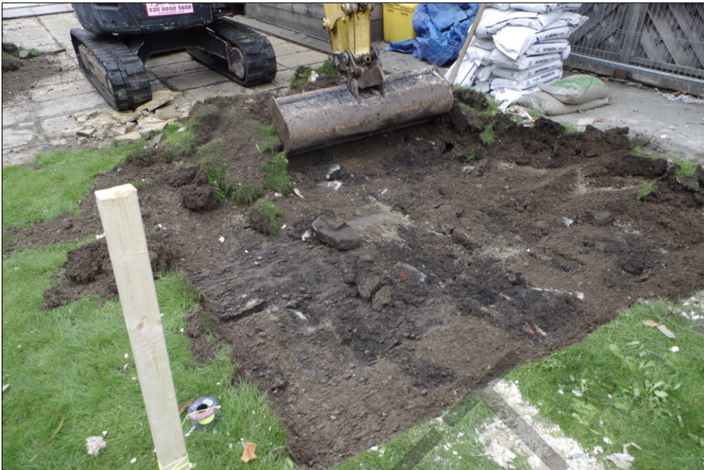
Plate 1: Made ground under grassed picnic area
