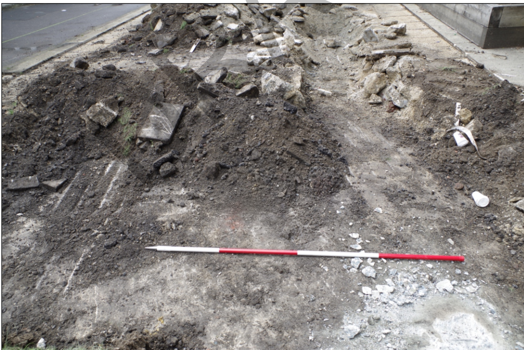
Plate 2: Made ground above concrete slab
