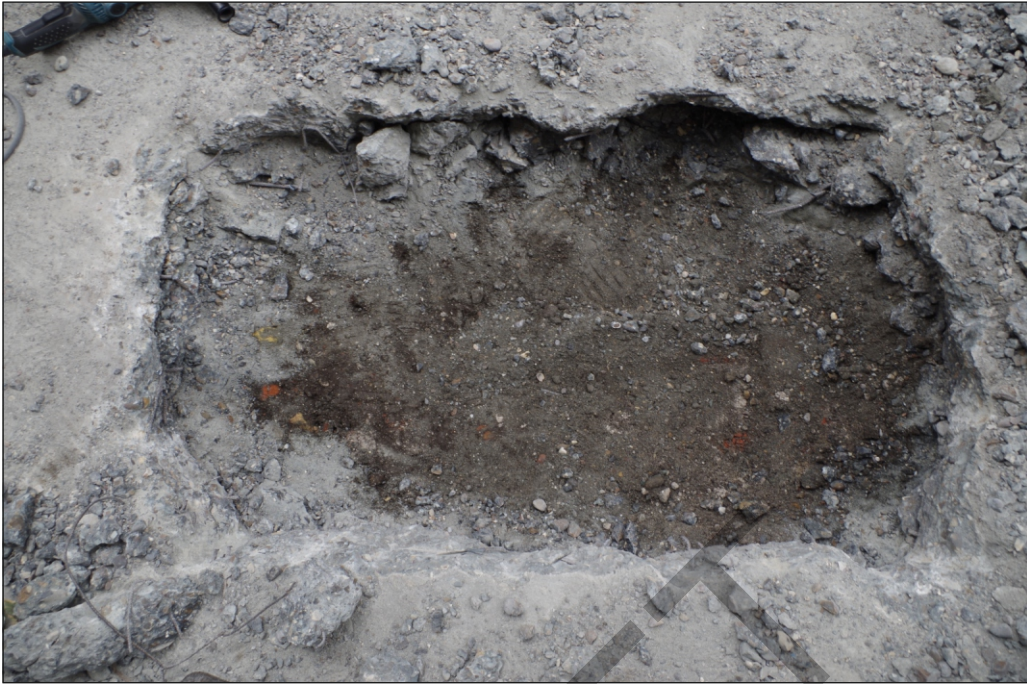
Plate 5: Made ground under concrete slab
