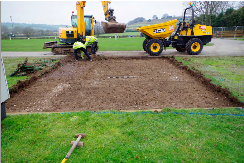
Plate 4: Topsoil strip for caravan hardstanding
