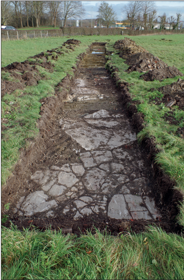
Plate 1: General shot of Trench 1, looking east-north-east
