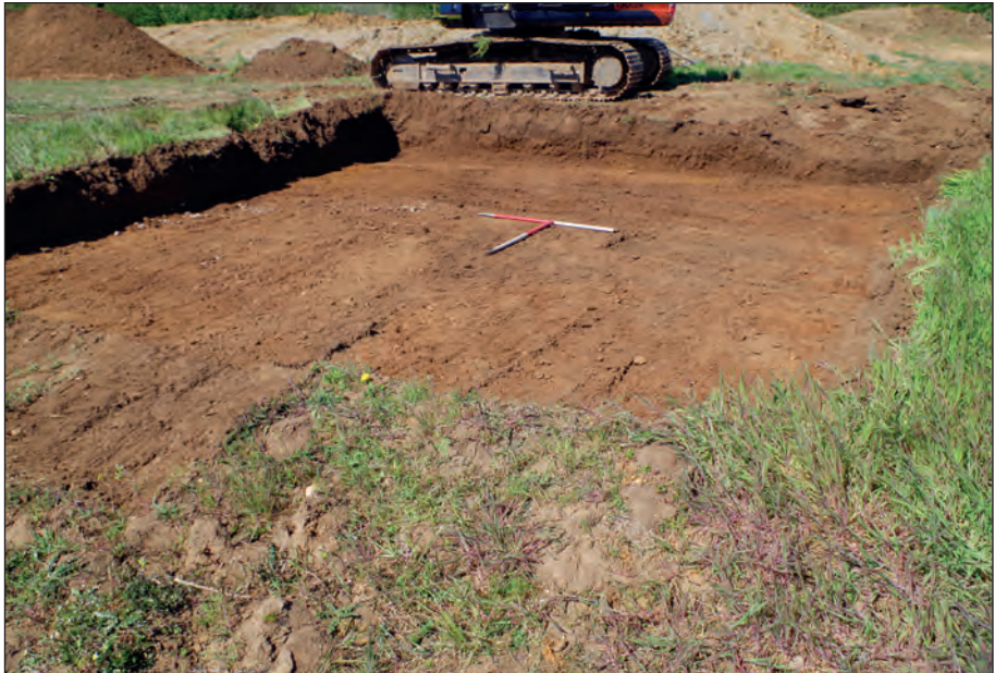
Plate 2: Smaller extension to the pumping station, viewed from the east
