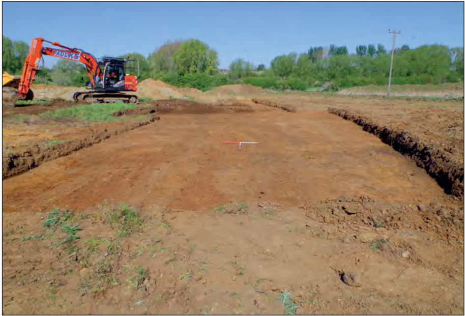
Plate 1: Larger extension to the pumping station, viewed from the south-west
