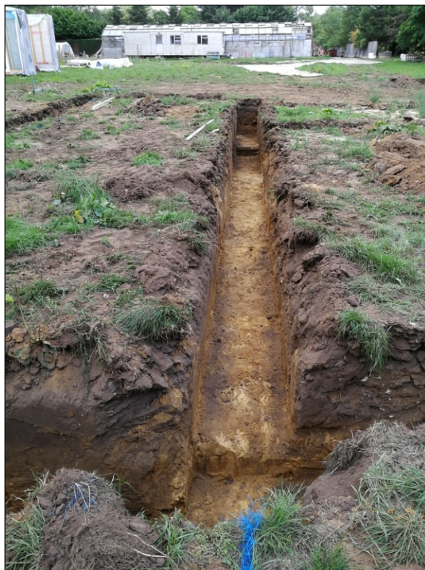
Plate 6: Excavated footing for Plot 3, view from the north
