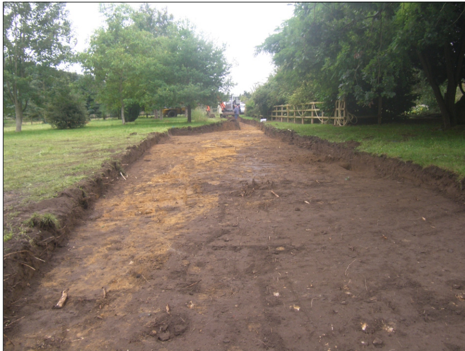
Plate 1: Access road excavation, view from the west
