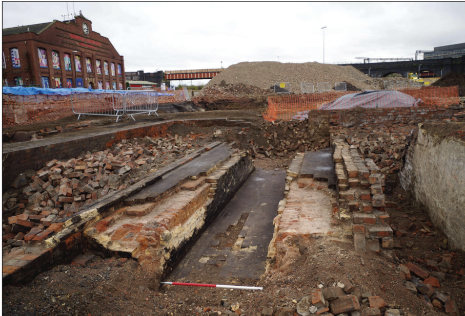
Plate 6: Firebrick steam boiler base 1128 – 1131 from North East
