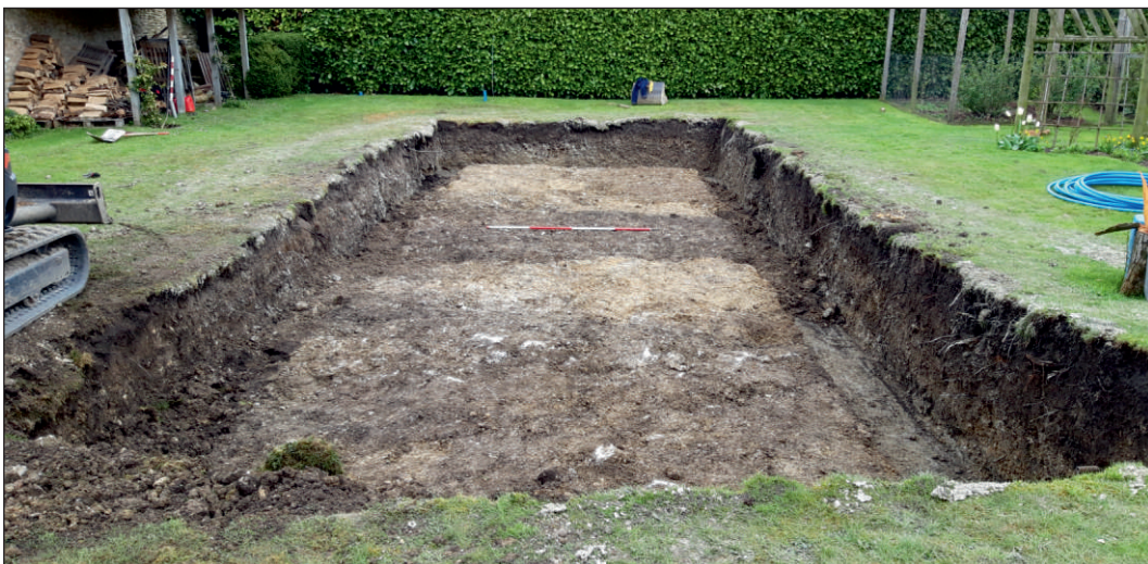
Plate 5: The monitored area down to the depth of the archaeological horizon showing ditch 104 (in the foreground), and ditch 106. The North facing Section 1 is on the right of the image. Scale 2 metres
