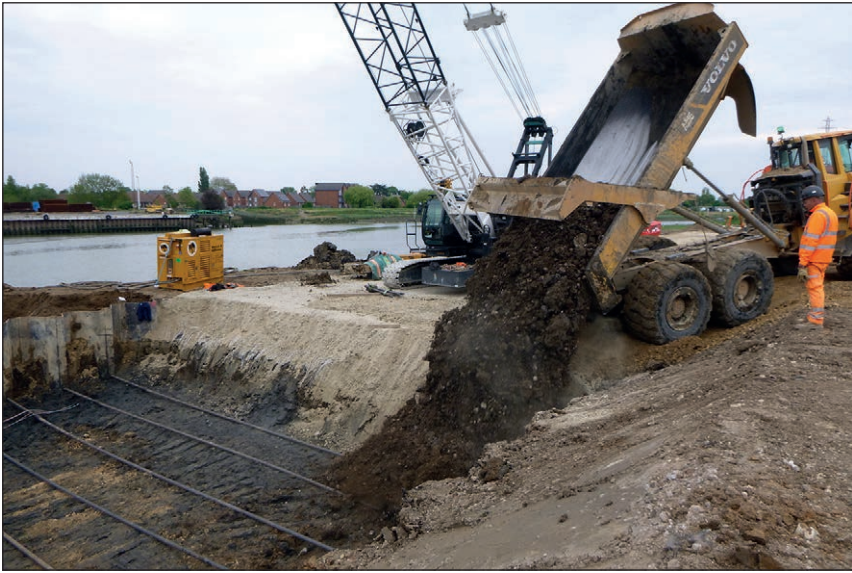
Plate 22: Backfilling the trench once the tie rods have been installed
