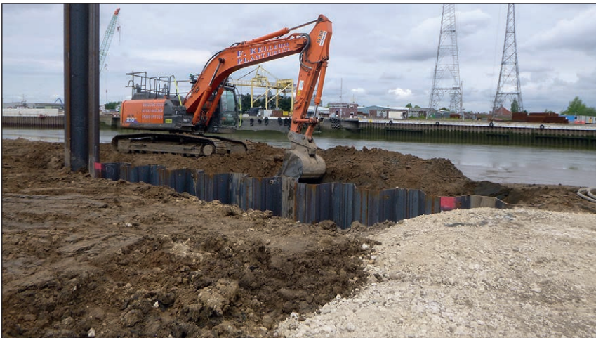
Plate 20: Removing sediment from outside of the piling
