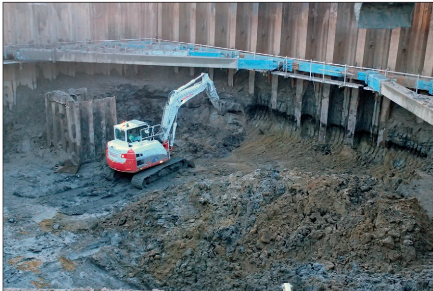
Plate 7: Excavating within the cofferdam. The horizon of peat is visible as a black line against the cofferdam wall
