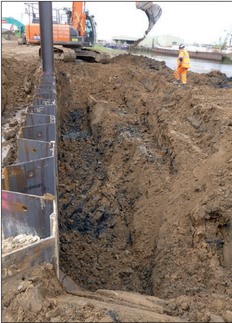
Plate 18: Removing sediment from outside of the piling
