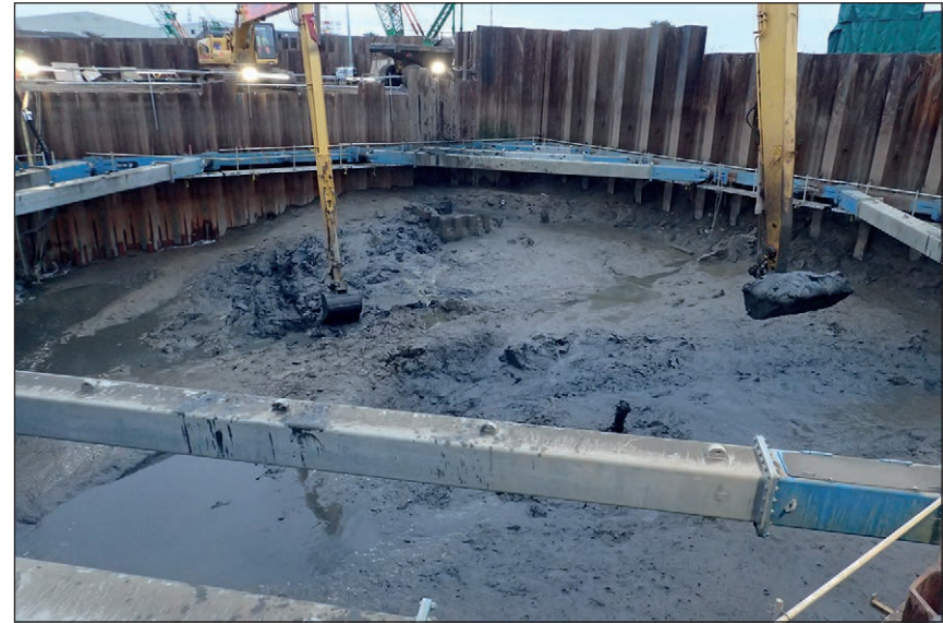
Plate 6: Excavating within the cofferdam
