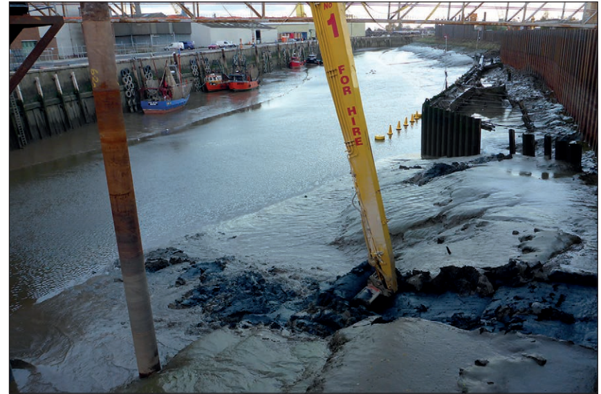
Plate 2: Dredging river to the east of the cofferdam from riverbank
