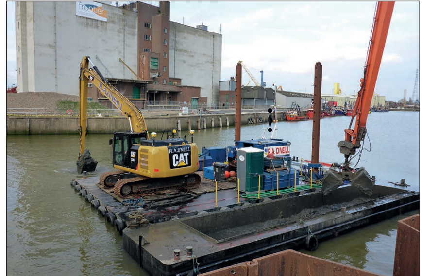
Plate 4: Dredging river to the east of the cofferdam from pontoon
