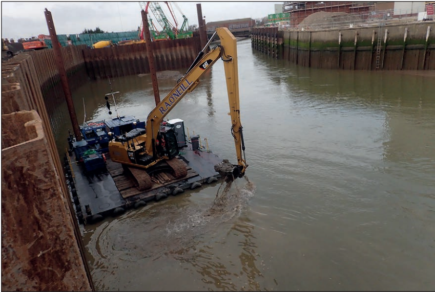
Plate 1: Dredging river to the east of the cofferdam from pontoon
