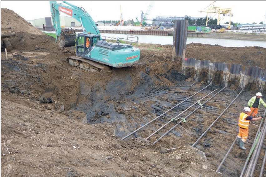
Plate 24: Installation of the tie rods in the trench while excavation is still ongoing
