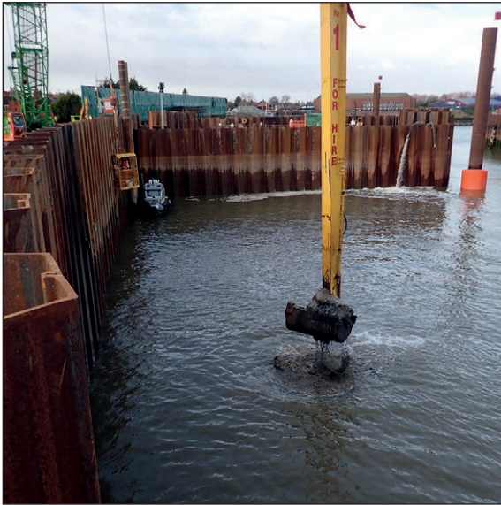
Plate 5: Dredging river to the east of the cofferdam from riverbank
