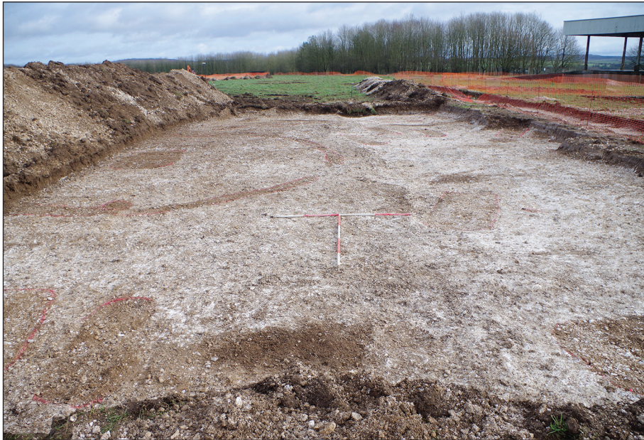
Plate 11: Trench 31 taken from the west. Scales are 2m
