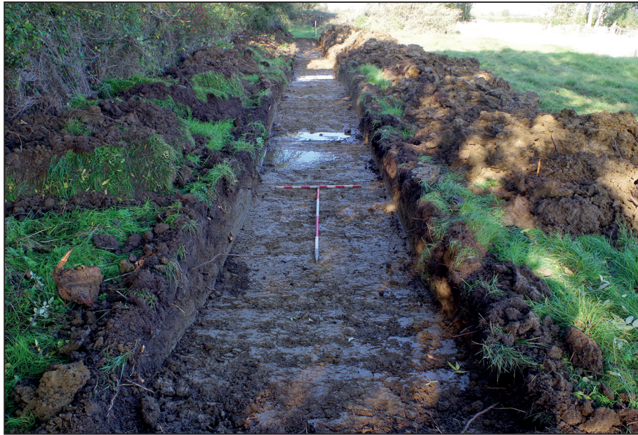
Plate 5: Shot of trench 59. View from south-east, 2.0m and 1.0 m scales.
