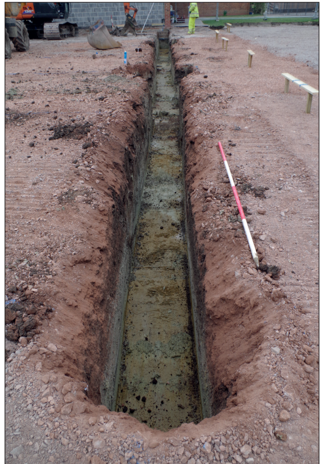
Plate 6: Footings in Trench 7 from the NW. Scales: 1 and 2 metre.
