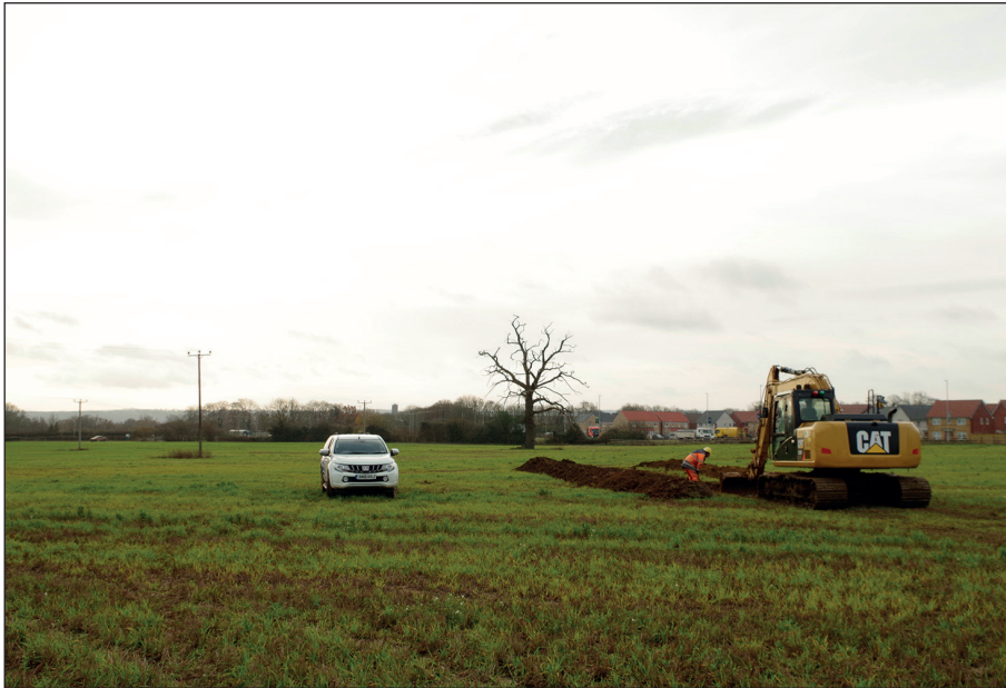
Plate 1: General view of the site showing trench 51, looking south-east.
