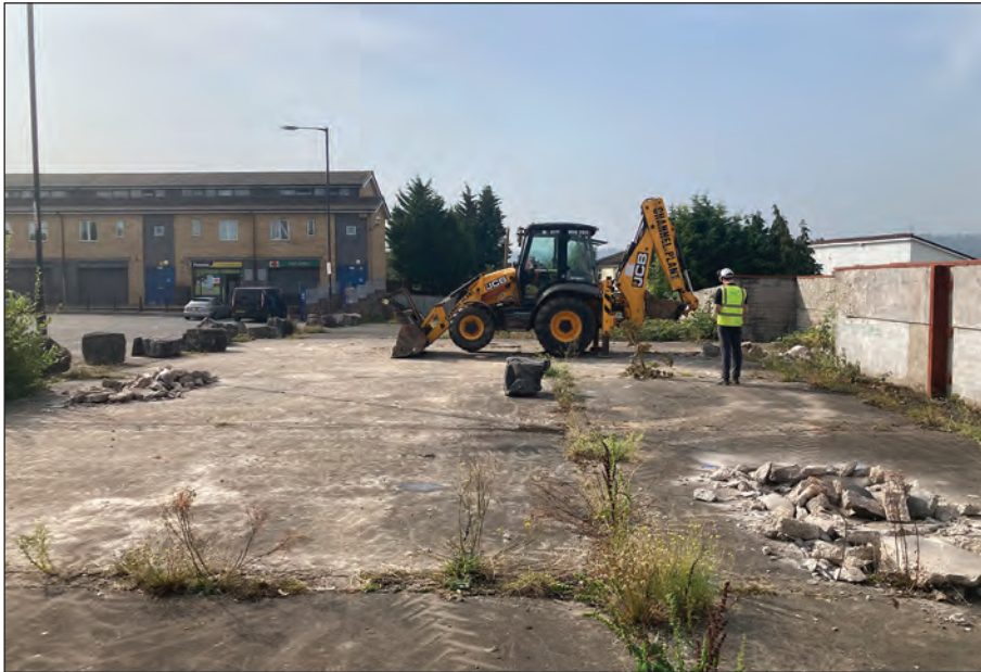
Plate 1: General view of the site, looking south
