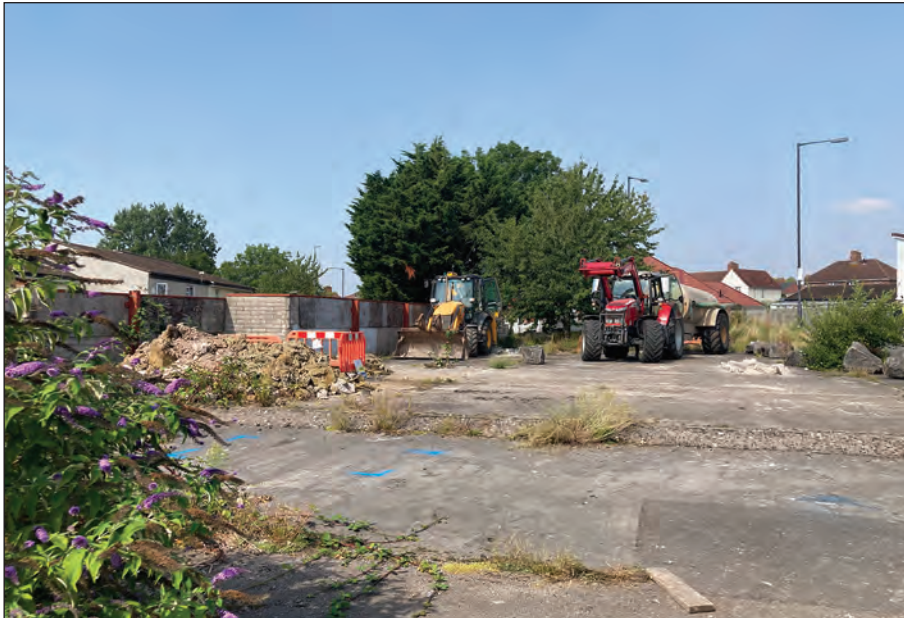
Plate 2: General view of the site, looking north
