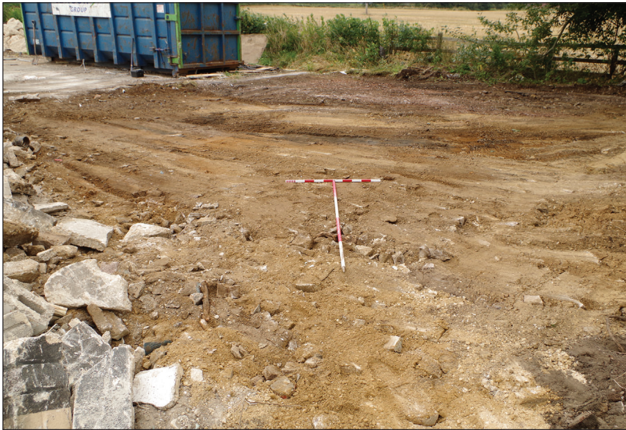
Plate 1: View of area 1 after removal of the concrete slab
