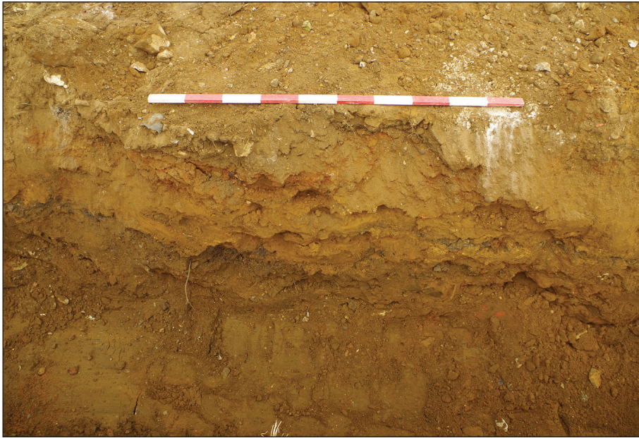
Plate 3: East facing view of section through a footings trench in area 3
