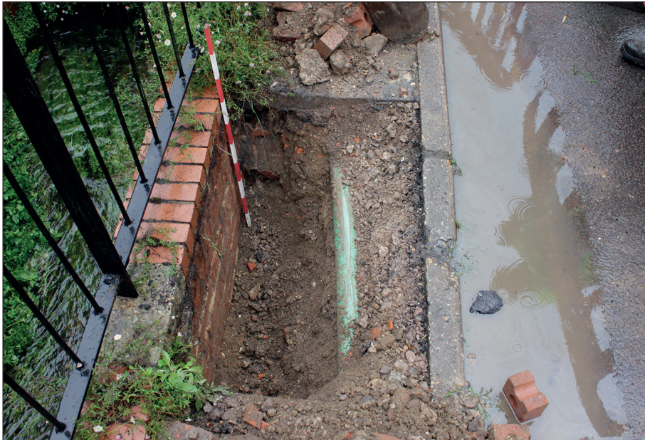
Plate 6: Northeast facing section of Trial Pit 6, with 1 m scale
