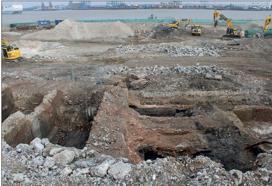
Plate 2: Overview of site conditions and works
