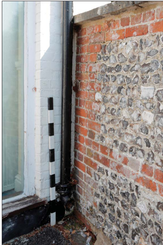
Plate 19: Join between the stable block and yard wall
