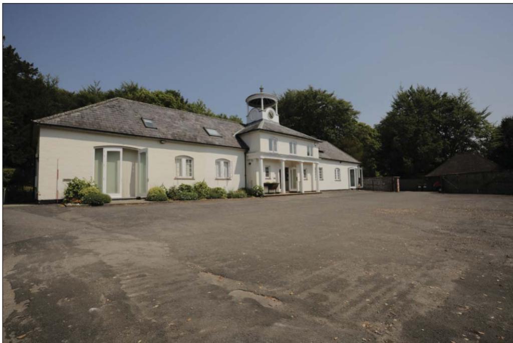
Plate 16: The listed (former) stable block
