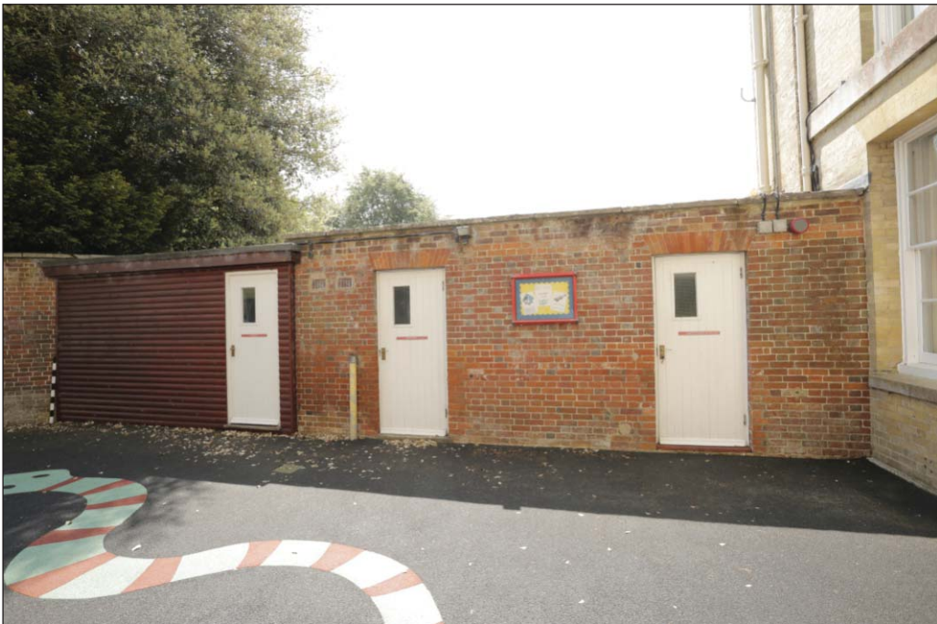
Plate 24: The music rooms north elevation
