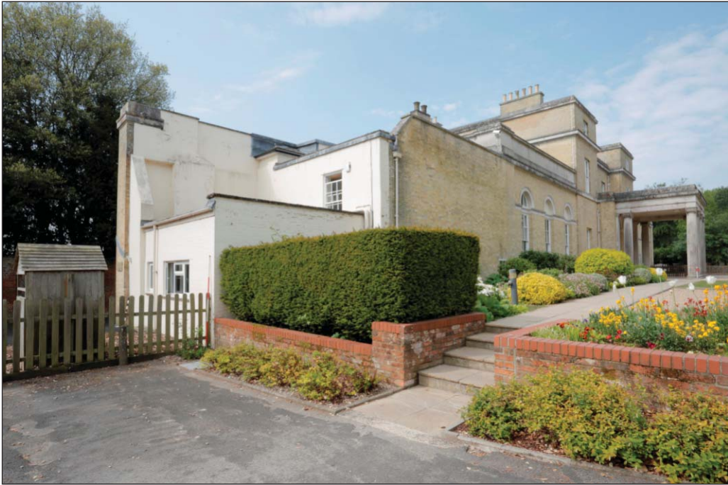
Plate 3: East end of Worthy Park House viewed from the north-east
