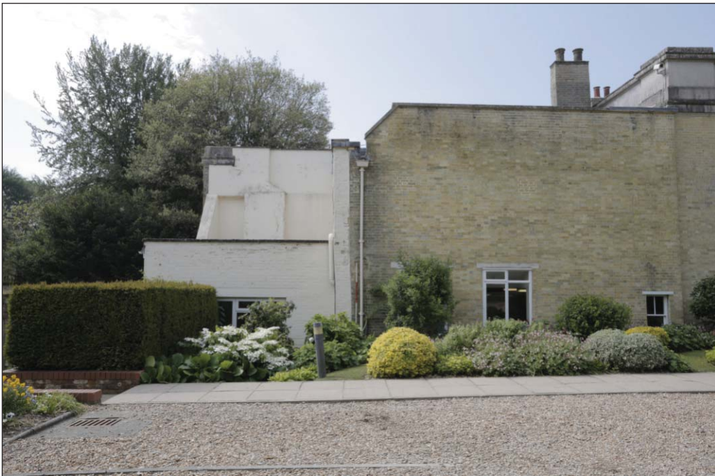
Plate 4: East end of Worthy Park House viewed from the north
