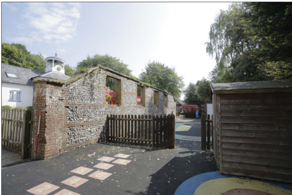
Plate 20: The former stable yard wall south elevation (outside the yard)
