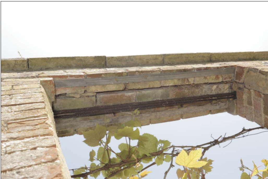
Plate 22: Detail of a window lintel within the former stable yard wall
