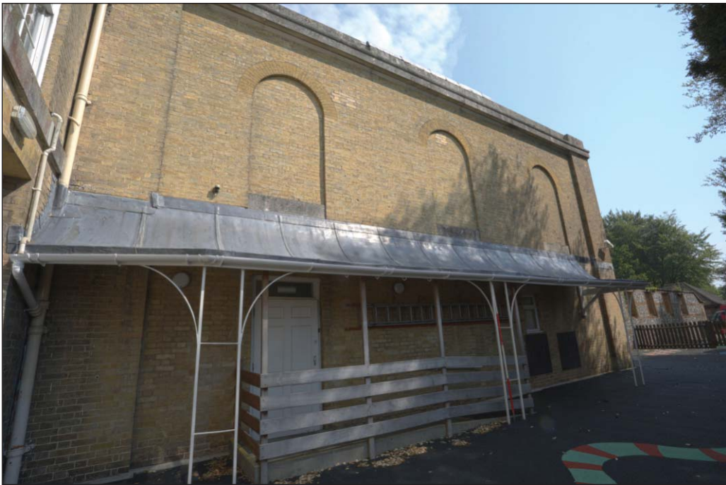
Plate 6: South elevation of the east end of Worthy Park House
