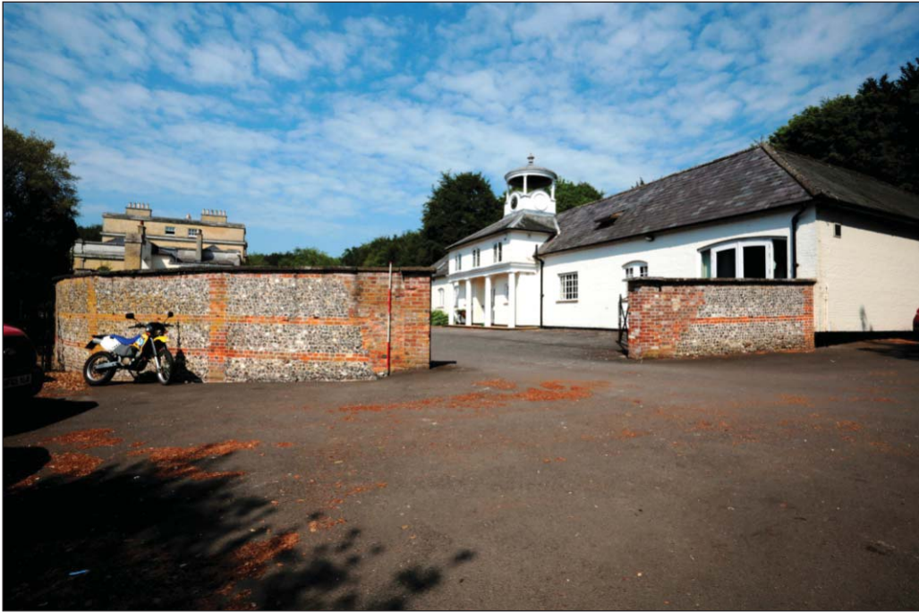
Plate 23: The east elevation and opening in the former stable yard wall plus the listed stable block in the background
