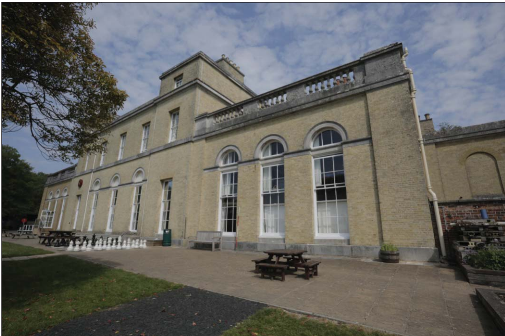
Plate 2: Worthy Park House south (rear) elevation viewed from the south-east
