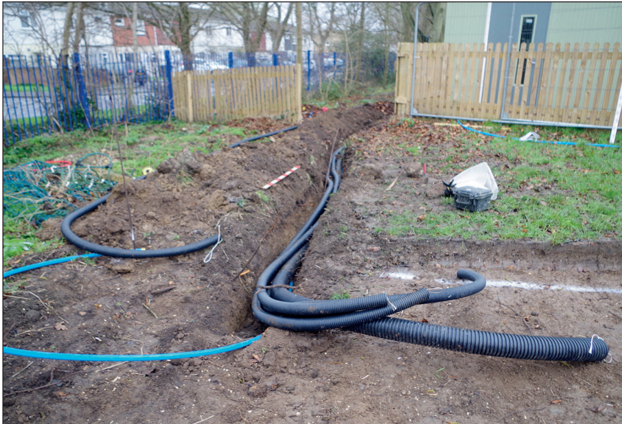
Figure 7: View through trench 2 from the north (1 m scale)
