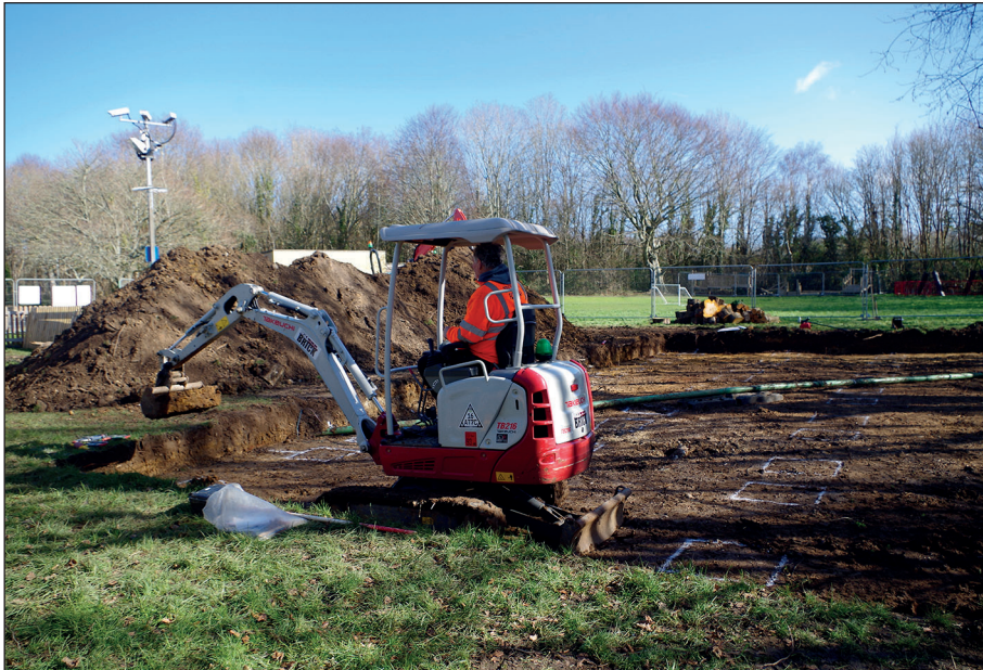
Figure 5: View from west of pad locations prior to excavation
