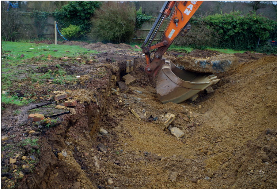
Figure 4: Excavation of the footings in Trench 1, view from East
