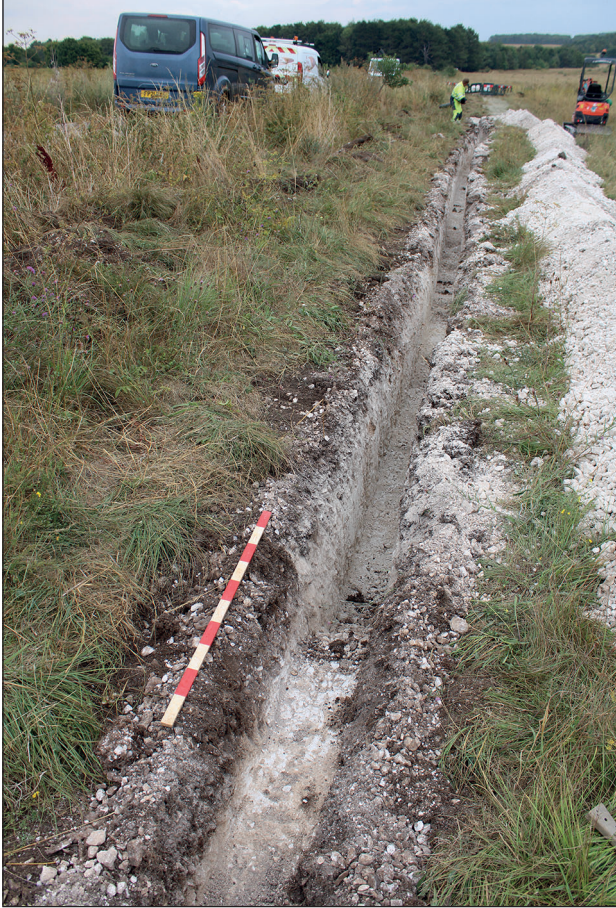
Figure 5: Cable trench from the south-west
