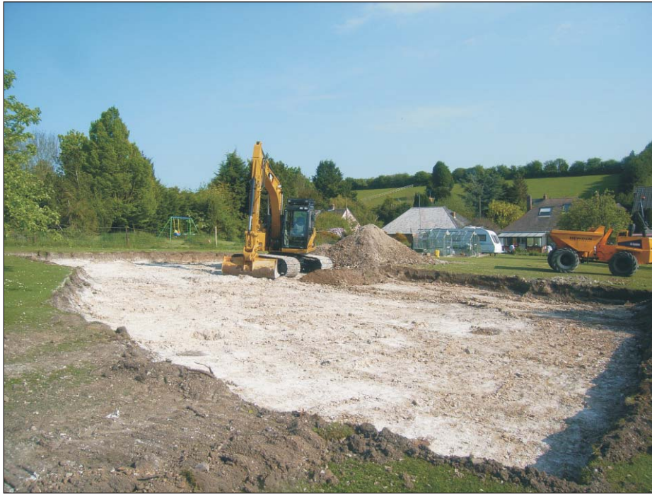
Plate 1: Site strip looking south-east
