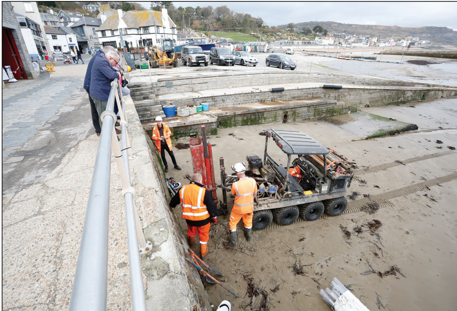
Plate 18: Window sample 107, percussive technique.
