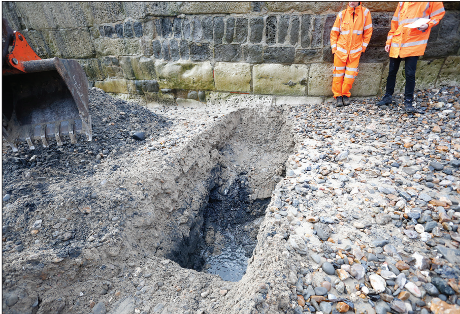
Plate 10: Excavation of Trial Pit 103.t
