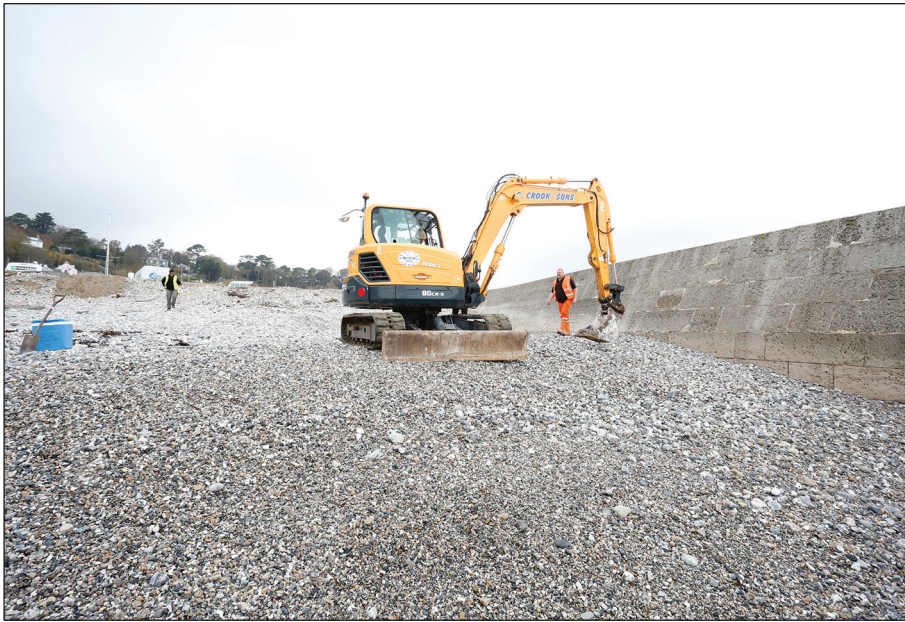
Plate 11: Location of Trial Pit 104.
