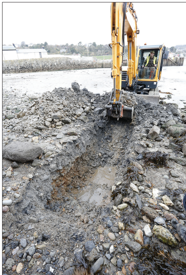
Plate 6: Excavation of Trial Pit 101.
