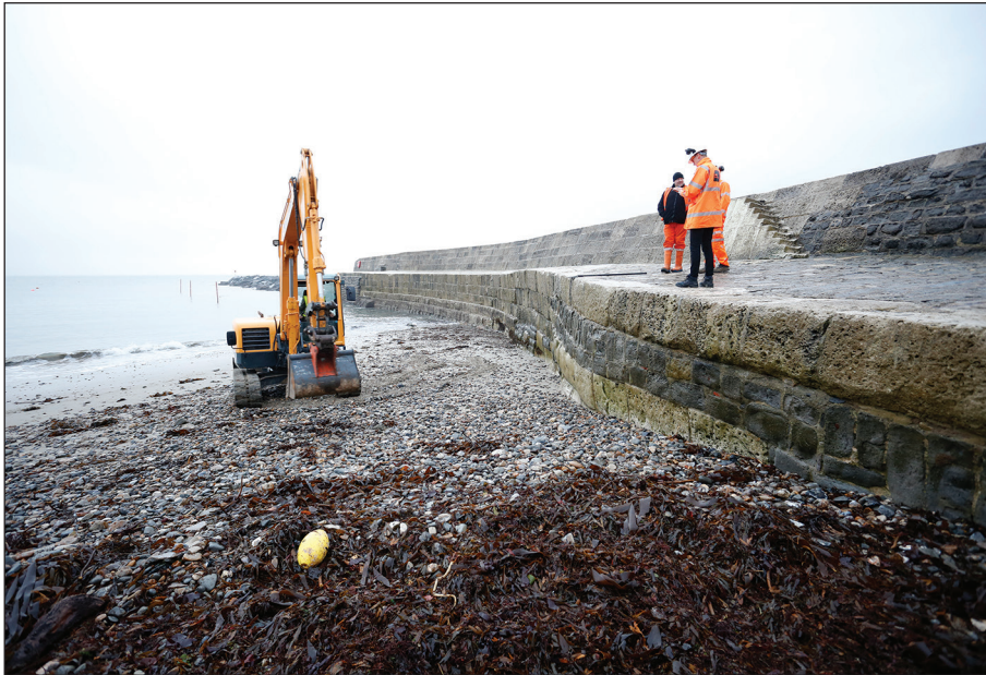
Plate 3: Southern Arm, west end, 1860's Biscuit Work below contractors.
