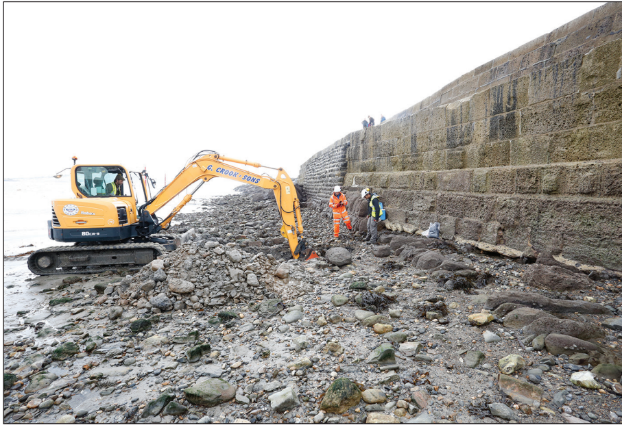
Plate 5: Location of Trial Pit 101.
