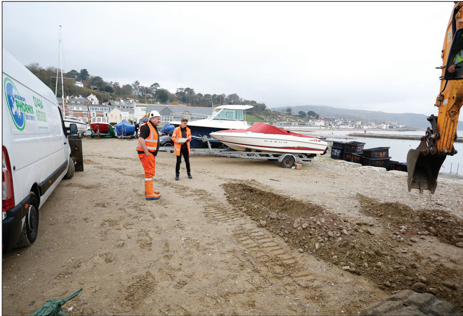
Plate 13: Location of Trial Pit 105.
