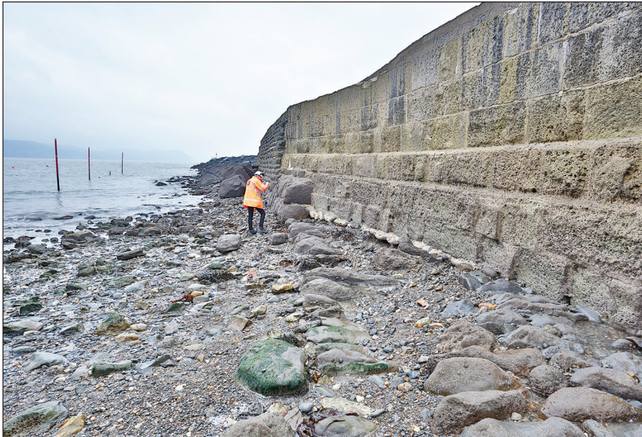
Plate 4: 16th century Cowstone foundation on earlier alignment, with later curving Ashlar Portland Stone above.
