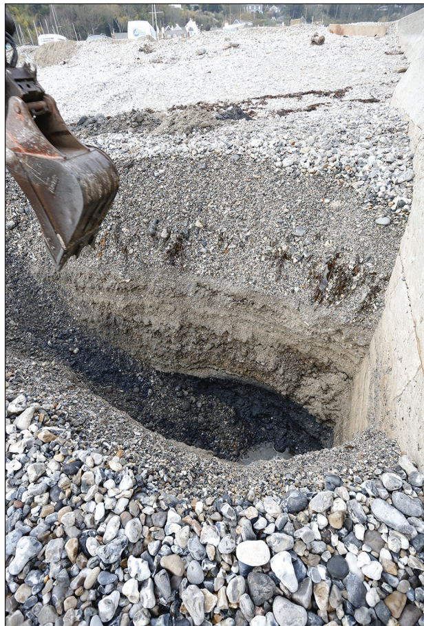
Plate 12: Excavation of Trial Pit 104.
