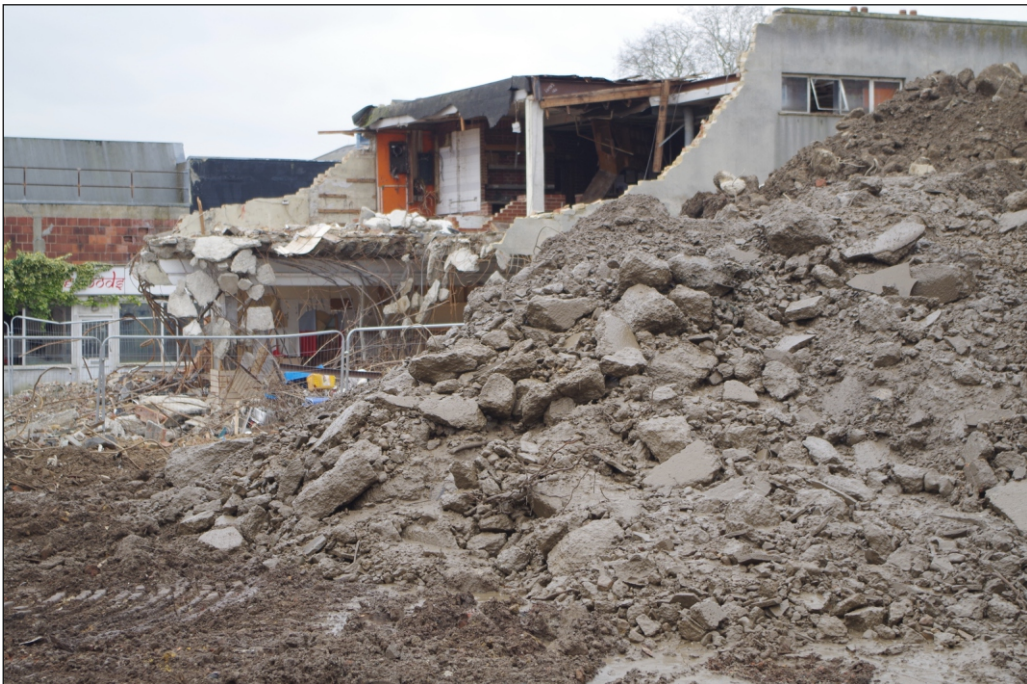
Plate 6: Partially demolished buildings in centre of site
