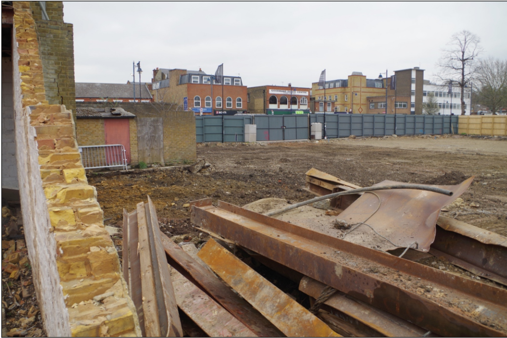
Plate 7: Area at north of site – madeground levelled ready for piling
