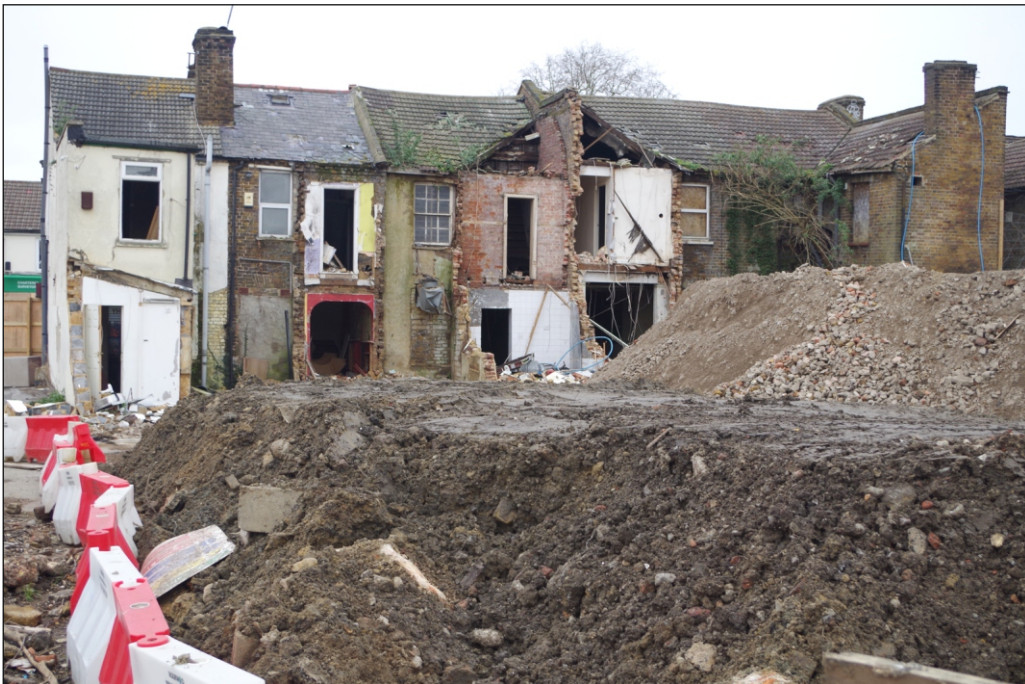
Plate 8: Partially demolished buildings fronting Lowfield Street
