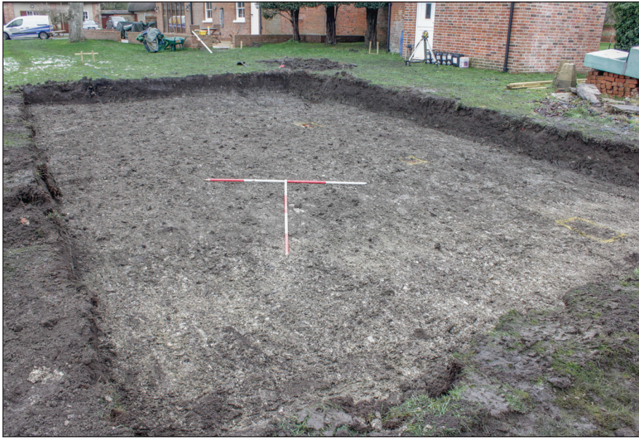
Plate 1: Excavated area from the south-east showing natural river terrace deposits
