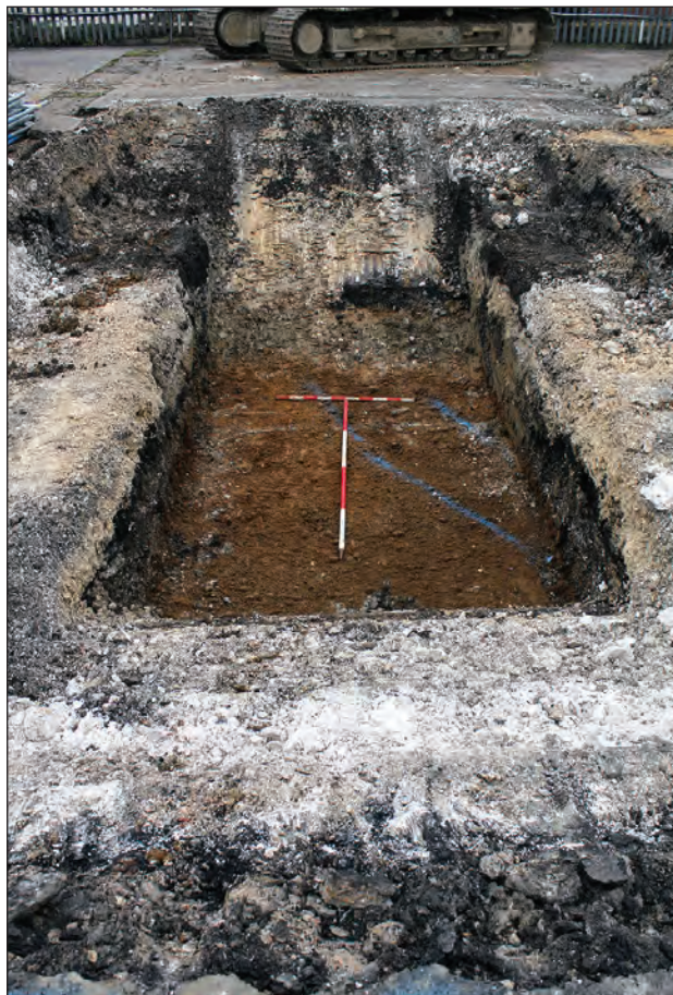
Plate 5: Trench 3, viewed from the south
