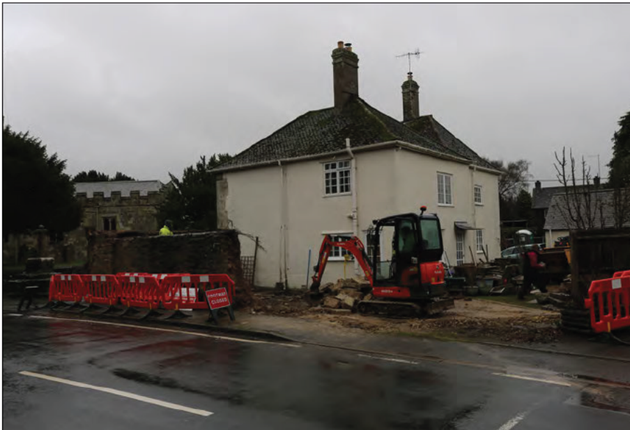
Photograph 20: The demolition of the walls in progress
