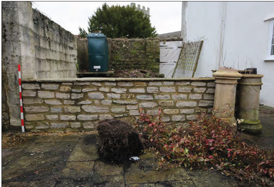
Photograph 14: The north-west side of the garden wall faced in stone
