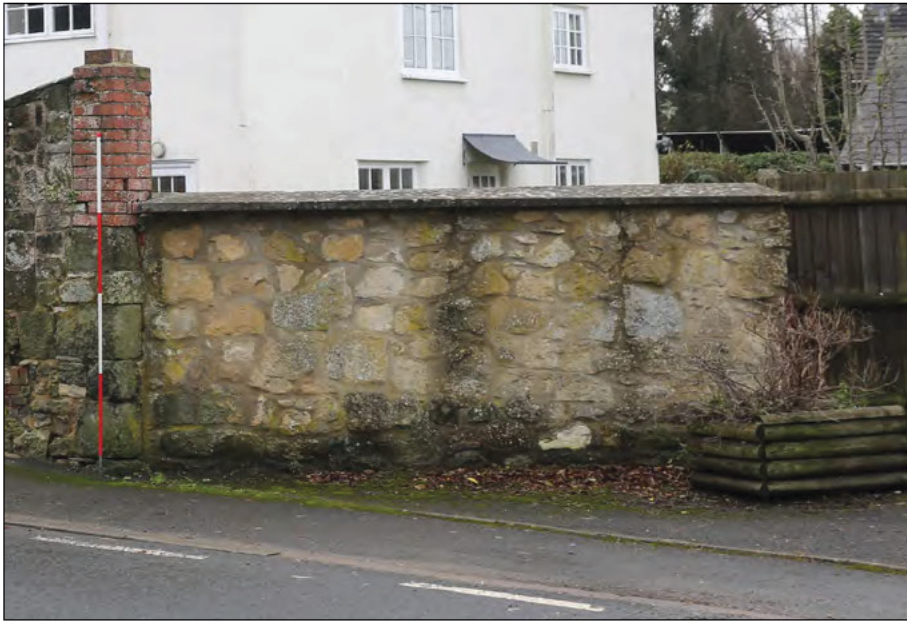
Photograph 3: The angled wall added as a later extension to the West Street boundary wall
