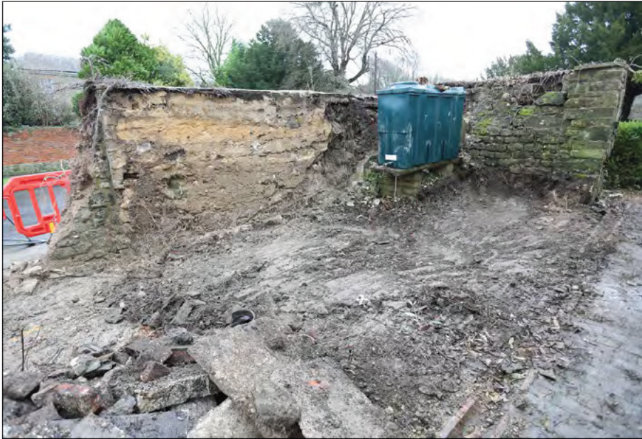
Photograph 21: The partially demolished walls viewed from the west
