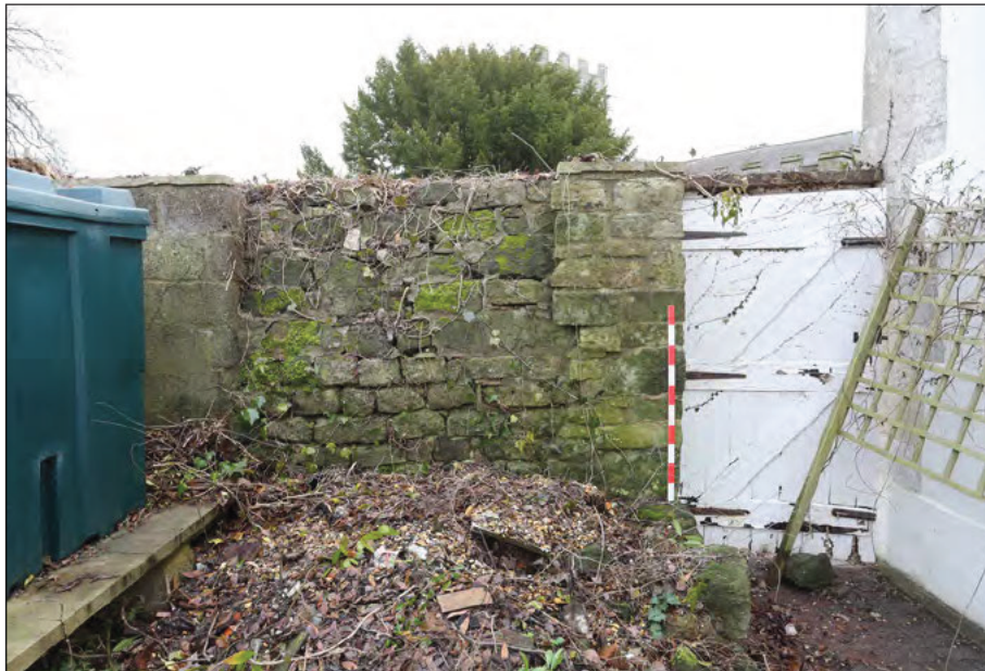
Photograph 18: The Duck Lane boundary wall north-west elevation
