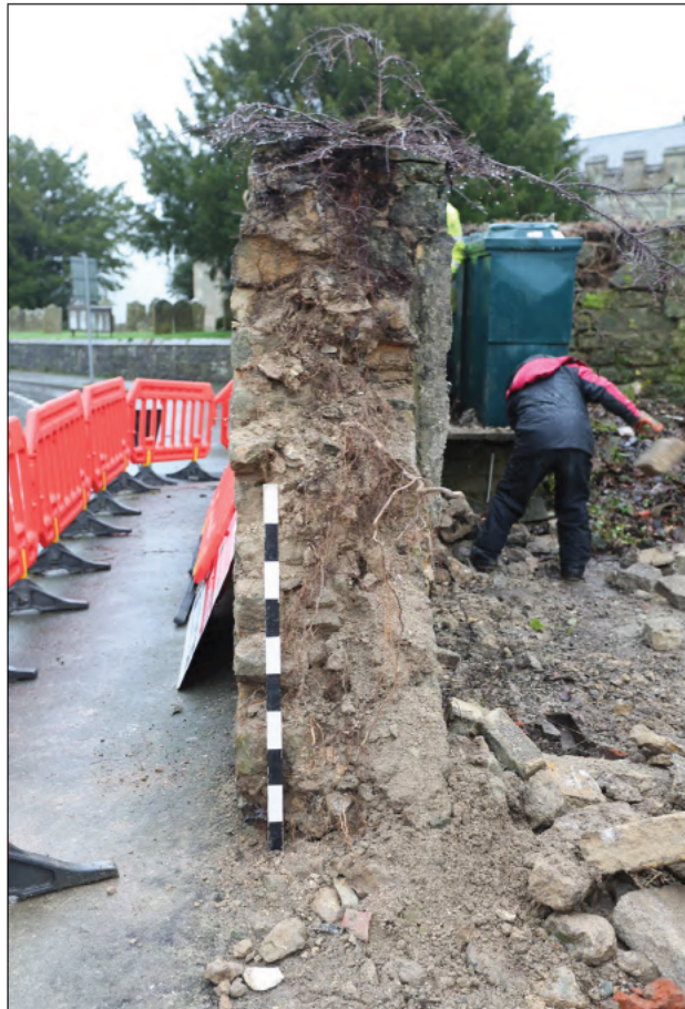
Photograph 22: Cross-section through the blocked doorway in the West Street boundary wall
