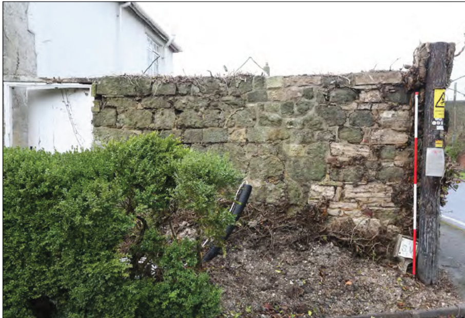
Photograph 17: The Duck Lane boundary wall south-east elevation
