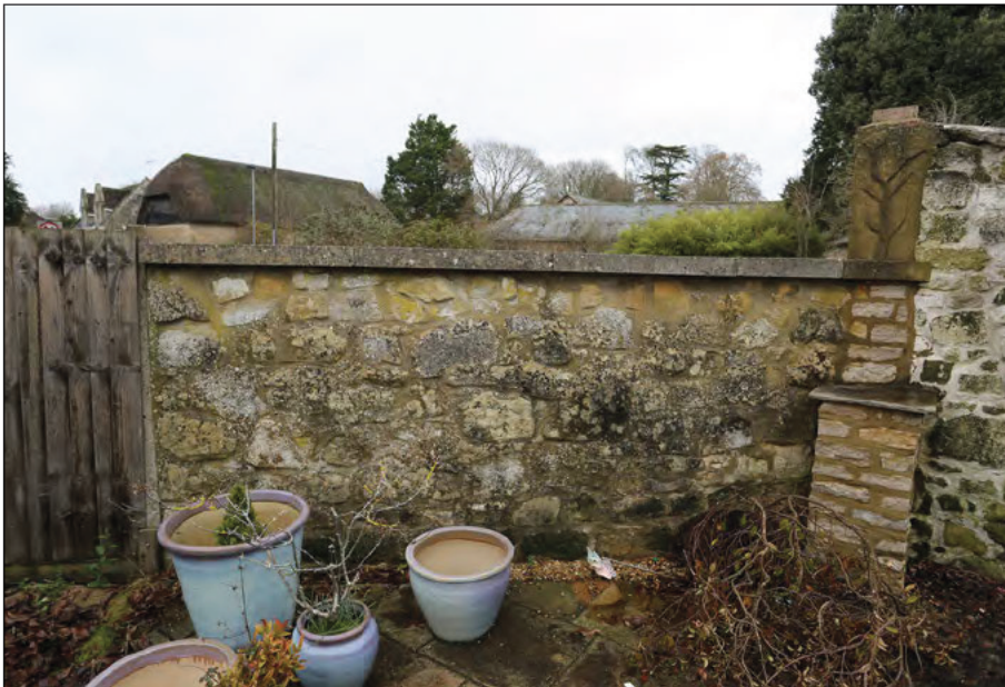
Photograph 16: The angled wall viewed from the south. Note the stone pier at the junction between the angled wall and the older West Street boundary wall
