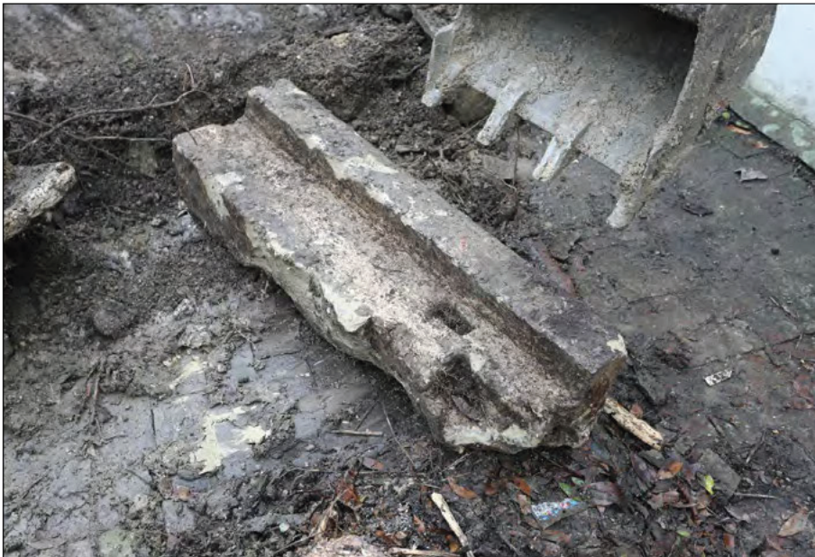
Photograph 26: The moulded L-profile limestone block interpreted as a lintel which was found during demolition
