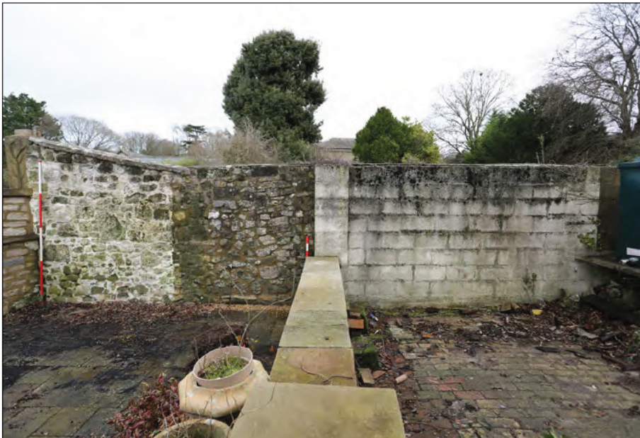
Photograph 12: The south-west elevation of the West Street boundary wall
