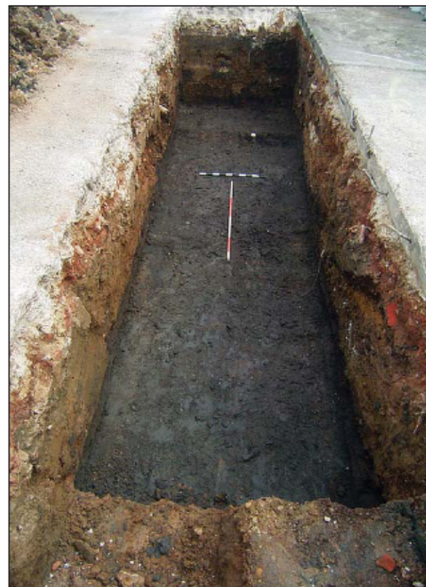
Plate 5: General shot of Trench 3, viewed from the west
