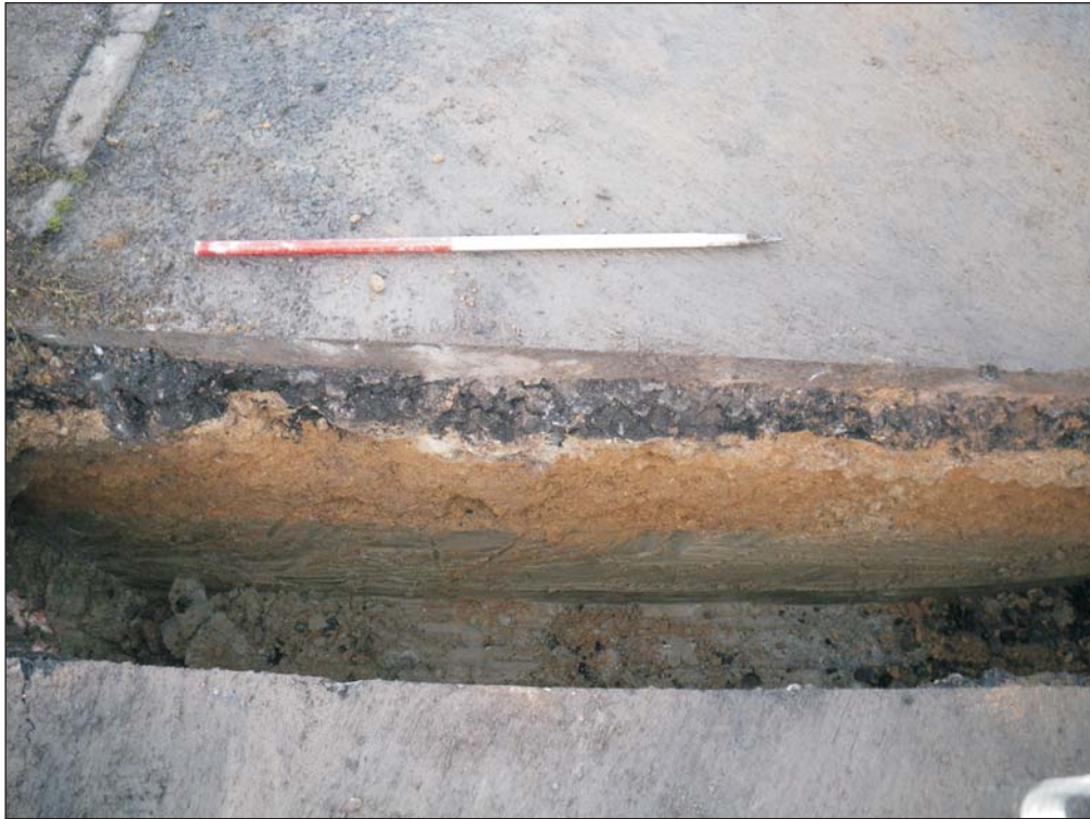
Plate 1: Representative section of verge excavations.
